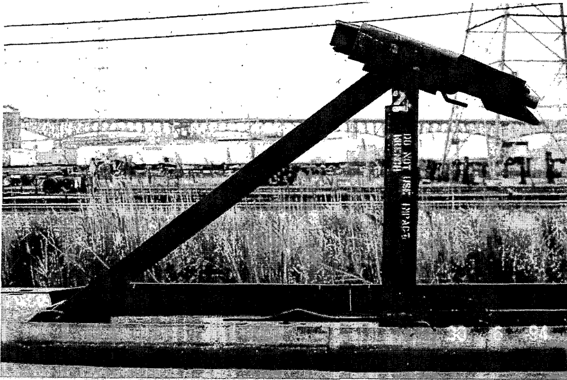
T - 17 Wrench operated retractable hitch.
