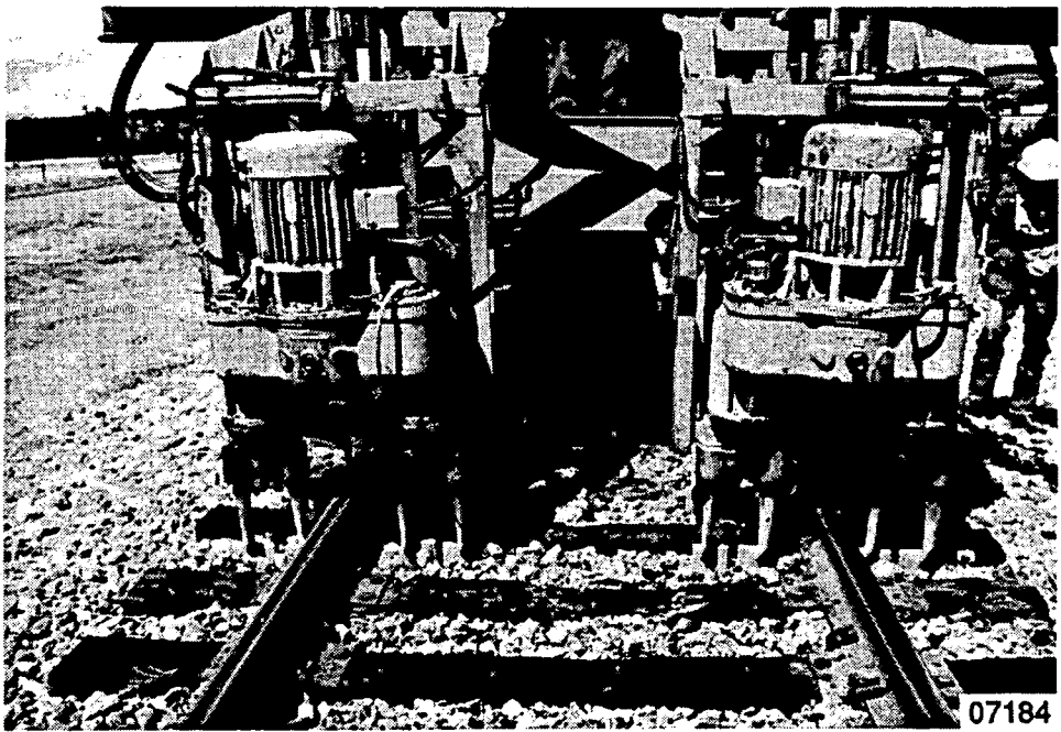
Figure C-6. Tamping in TSI
