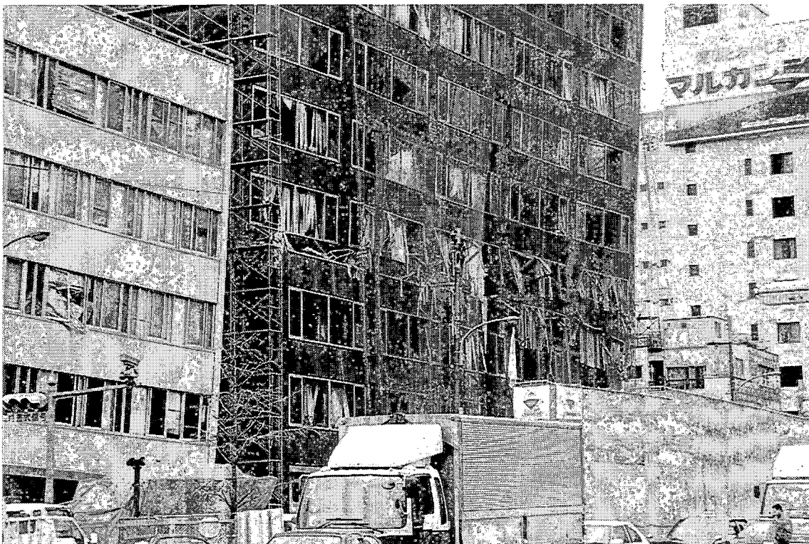
SS-7 & SS-8. These buildings next to Sannomiya Station were also heavily damaged. The one to the left is leaning. The darker building sheared about 2 meters at the fourth floor and appears quite dangerous.
