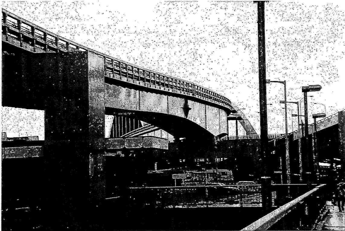
PI-11. The steel box girder span approaching the arch span was undamaged.
