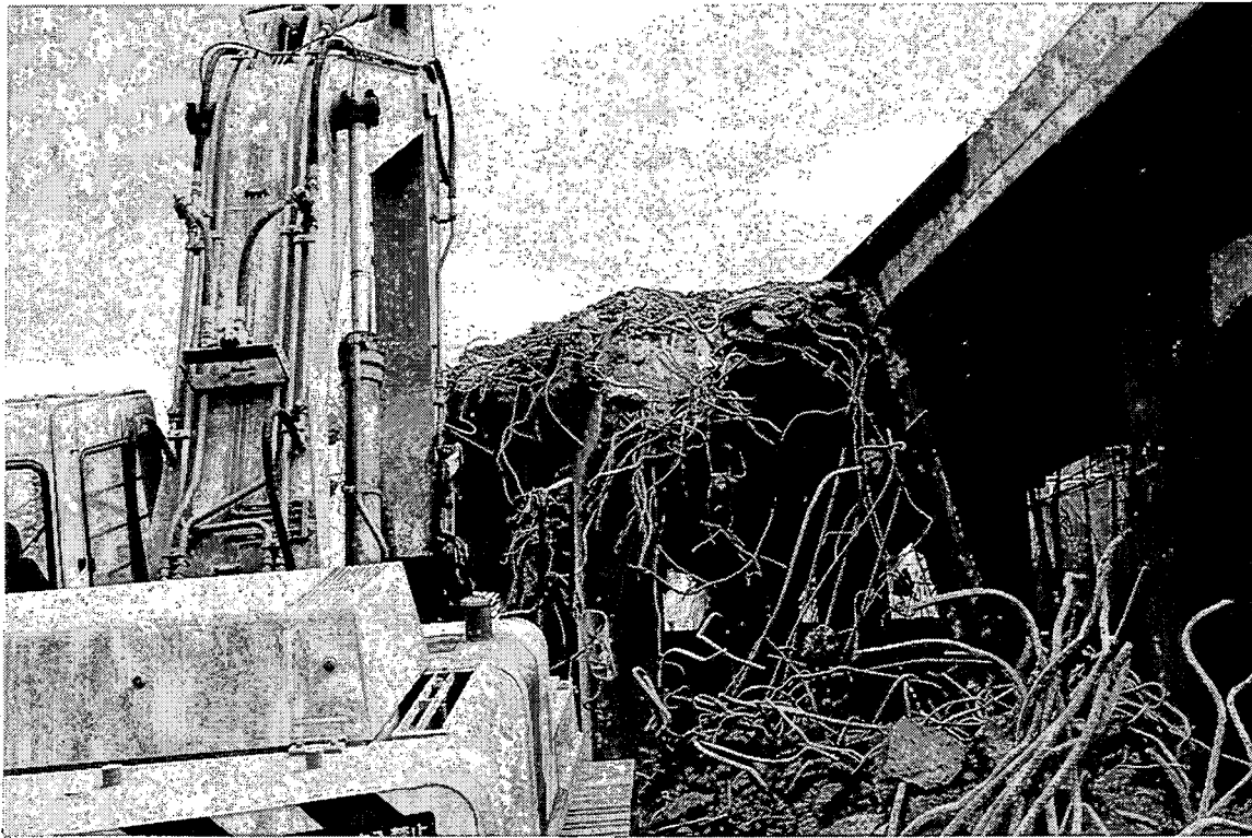
HC-8. Demolition of the final section of concrete viaduct. Note the clean edge separating the parallel structures.
