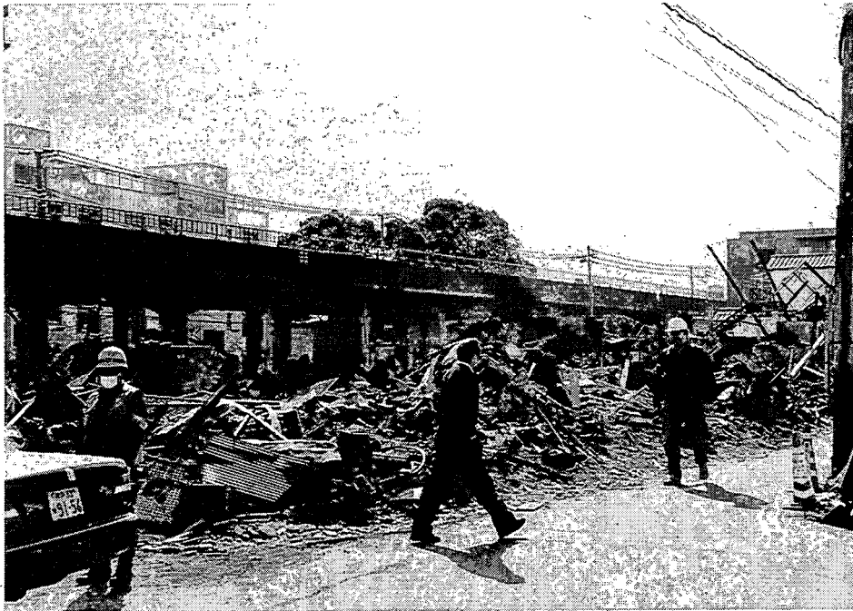
HER-35. Viaduct is seen over the remains of a residential block.
