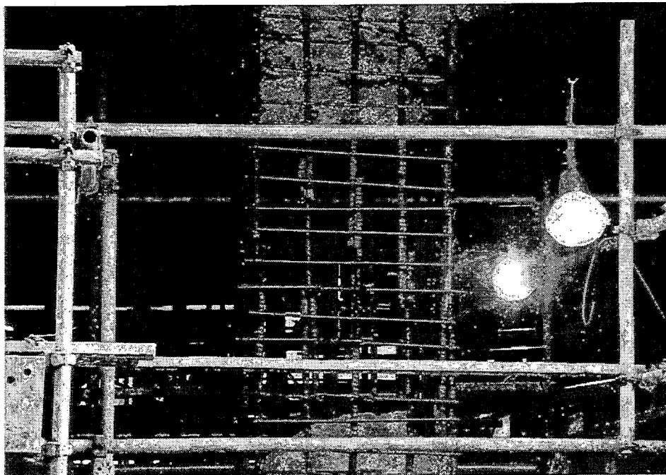
JRT-28. Typical column repair. Note the tie spacing, splices and lack of cross ties.
