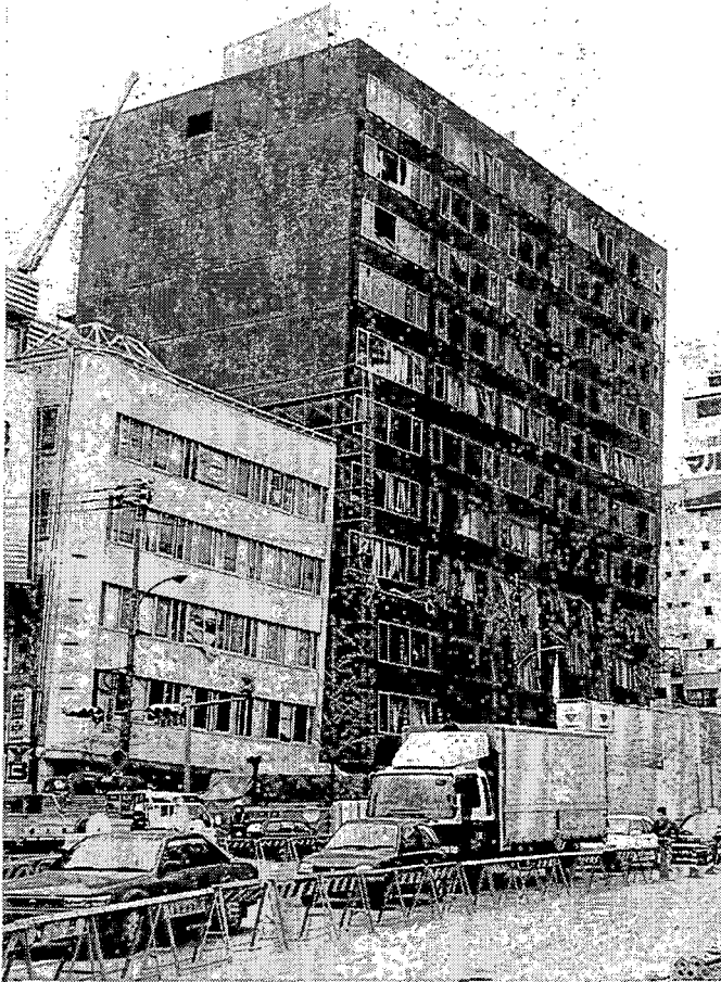
SS-7 & SS-8. These buildings next to Sannomiya Station were also heavily damaged. The one to the left is leaning. The darker building sheared about 2 meters at the fourth floor and appears quite dangerous.
