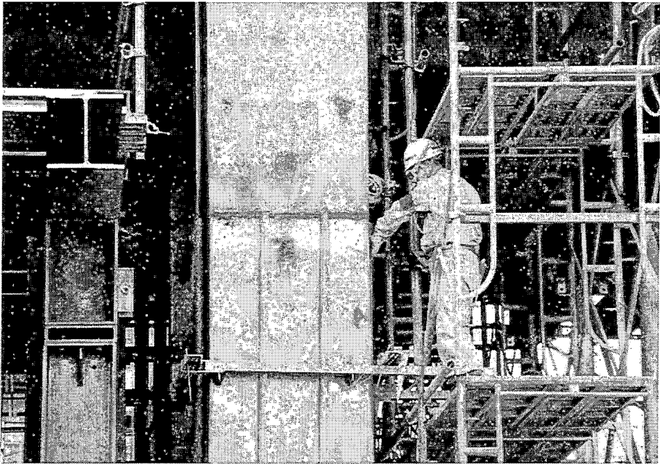
JRT-33. Welder is preparing to seal steel plate jacket.
