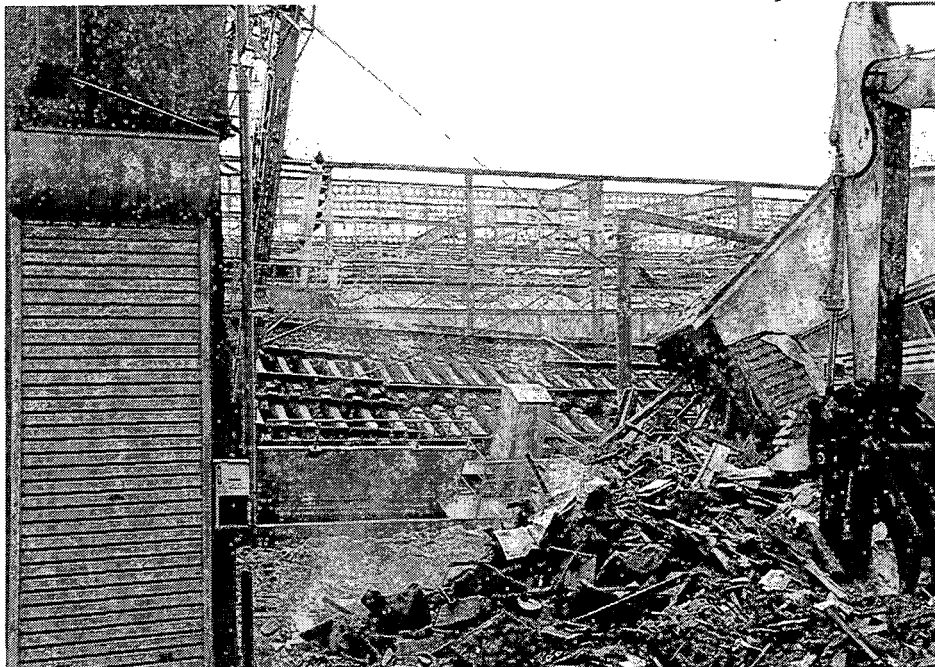
HER-24. The viaduct fell in the foreground. The train parking area in the background collapsed derailing 58 cars.
