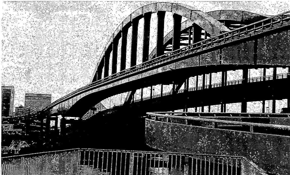
PI-13. The single arch bridge in the foreground carried the people mover south to Port Island. It appeared undamaged. The highway bridge at the bottom right was severely damaged in the next span. The double deck arch in the background supports highway traffic.
