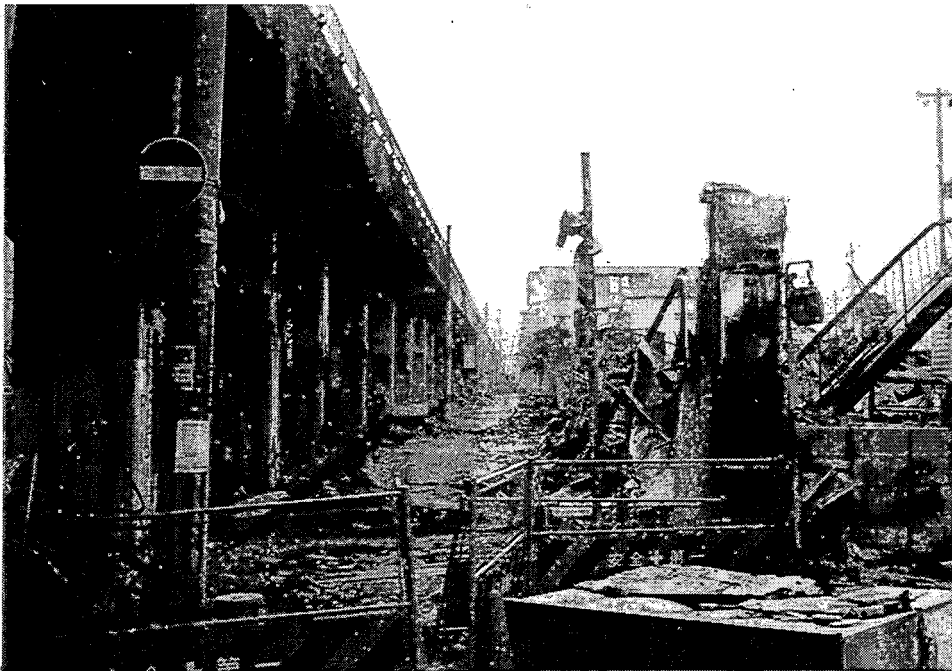
HER-34. West of the station the damaged viaduct continues for at least another kilometer. The structure was blackened by fires that consumed many blocks. There isn't as much damage here. The structure is a little taller.
