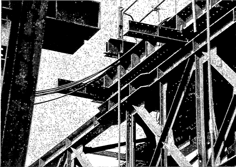
JRT-9. The hydraulic jacks lift the vertical rods which are cored through the girders. The rods look like high strength rebars.
