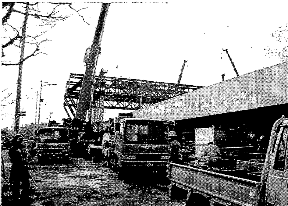
JRT-15. The viaduct here is very short and susceptible to shear forces. The collapsed sections are consistent with high shear force demand.
