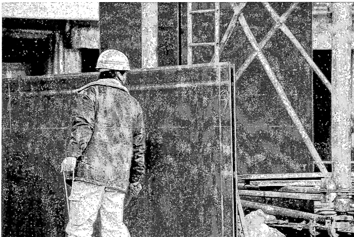
JRS-17. This construction worker is standing on a steel jacket. The jacket is nearly 1.5 meters on a side and only 9 mm thick.
