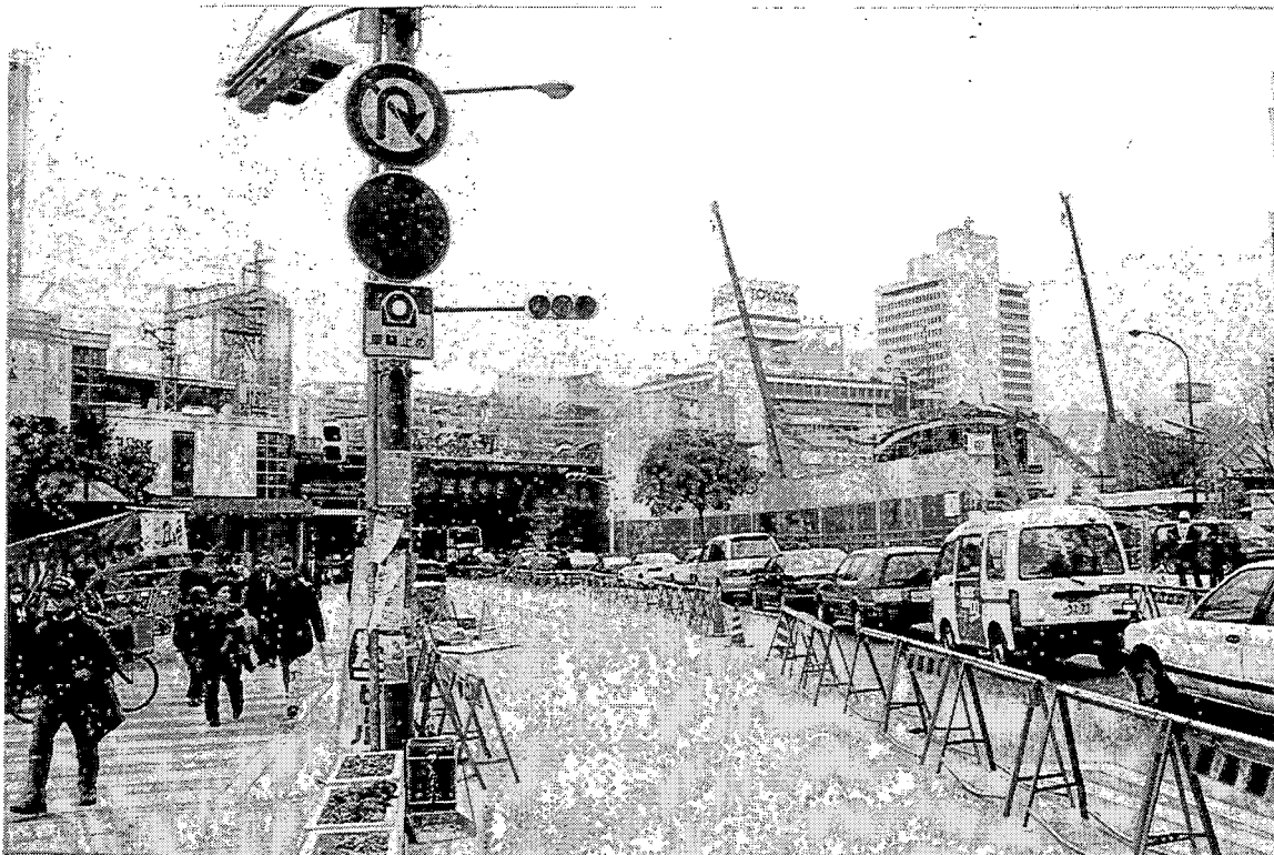
SS-4. This area of Kobe was very heavily damaged. The JR Sannomiya Station is elevated crossing the street. The Kobe Municipal Subway Station is closed for repair behind the barriers to the far left. The Hanshin Subway was damaged below the street just beyond the bridge. The Port Island Peplemover is down this street about 1km.
