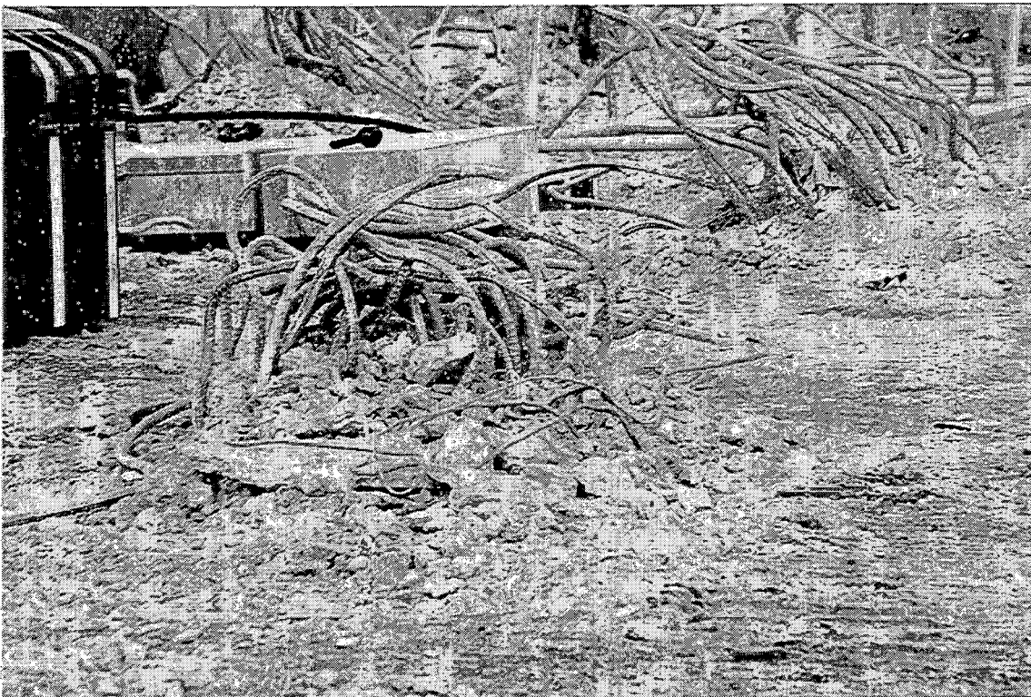
HC-17. Remnants of the failed viaduct
