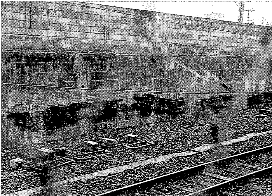
JRT-4. Retaining embankment through bolts as seen from the back face of the wall.
