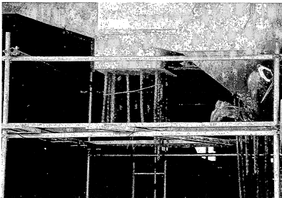
JRT-16. In some areas the columns were cut at the top with 500mm left of the main reinforcing.
