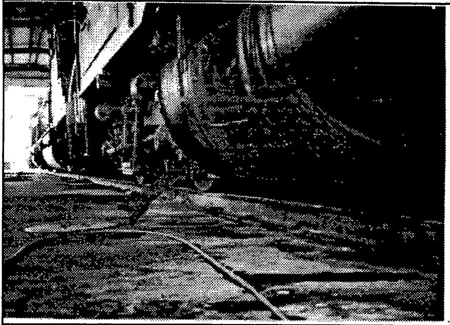
**Figure 3.22 Damage Due to Motor Vehicle Collision with Fuel Tank**
