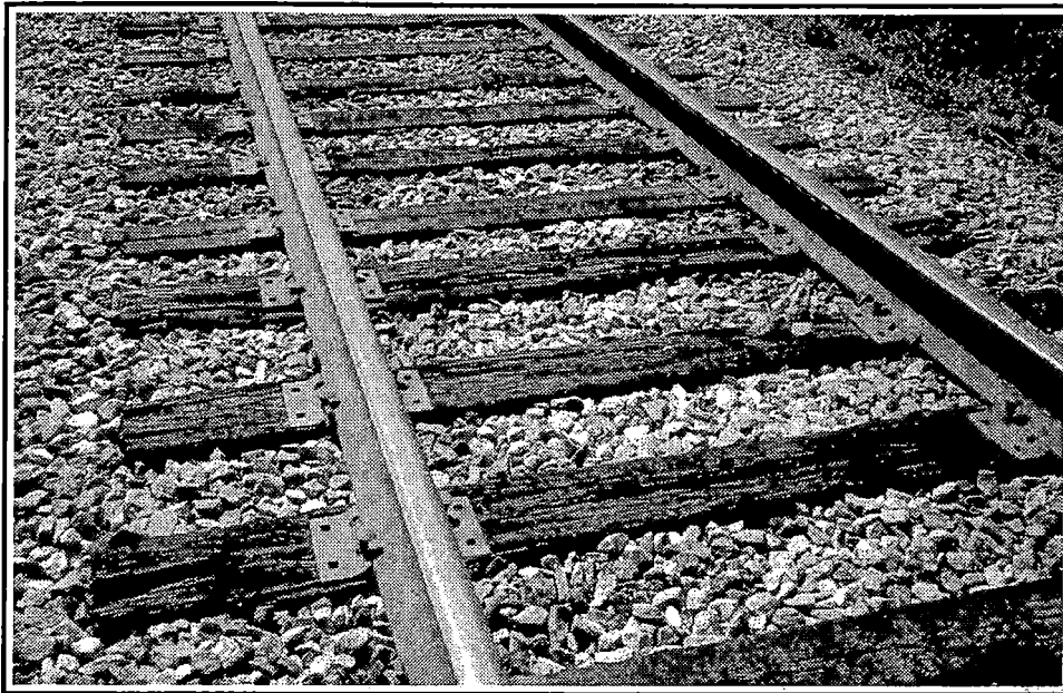
Exhibit 48. A Poorer Segment of Baseline Track near Milepost 118
