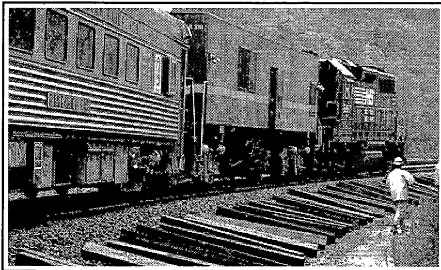
Exhibit 36 TLV Track Strength Testing in Conjunction with Track Maintenance in NS track
