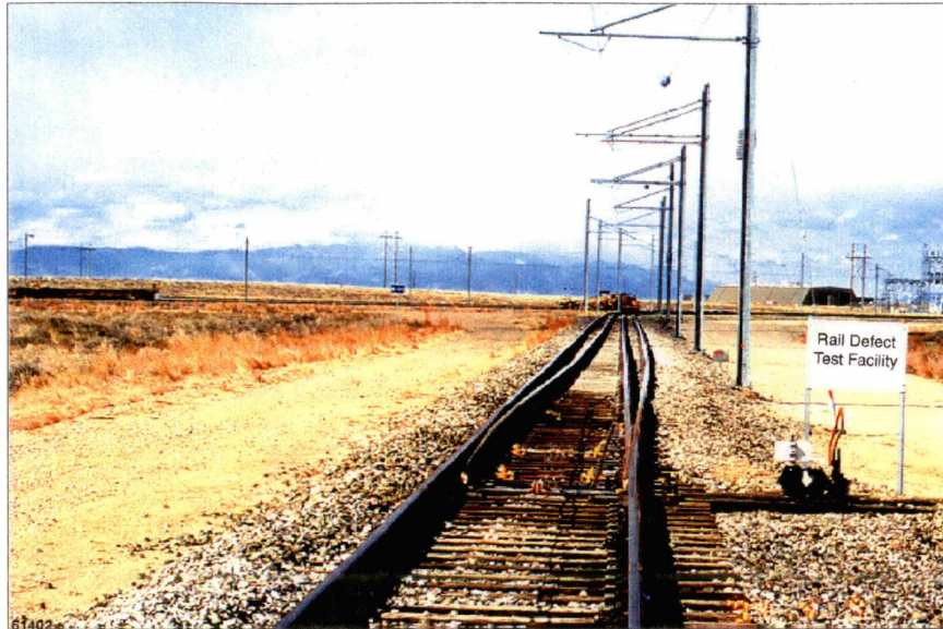
Figure 1. Tangent Section of the Rail Defect Test Facility
