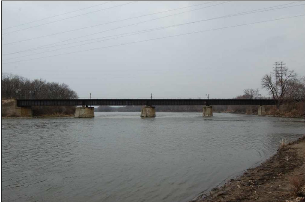
Exhibit 3-5. Kankakee River Bridge
