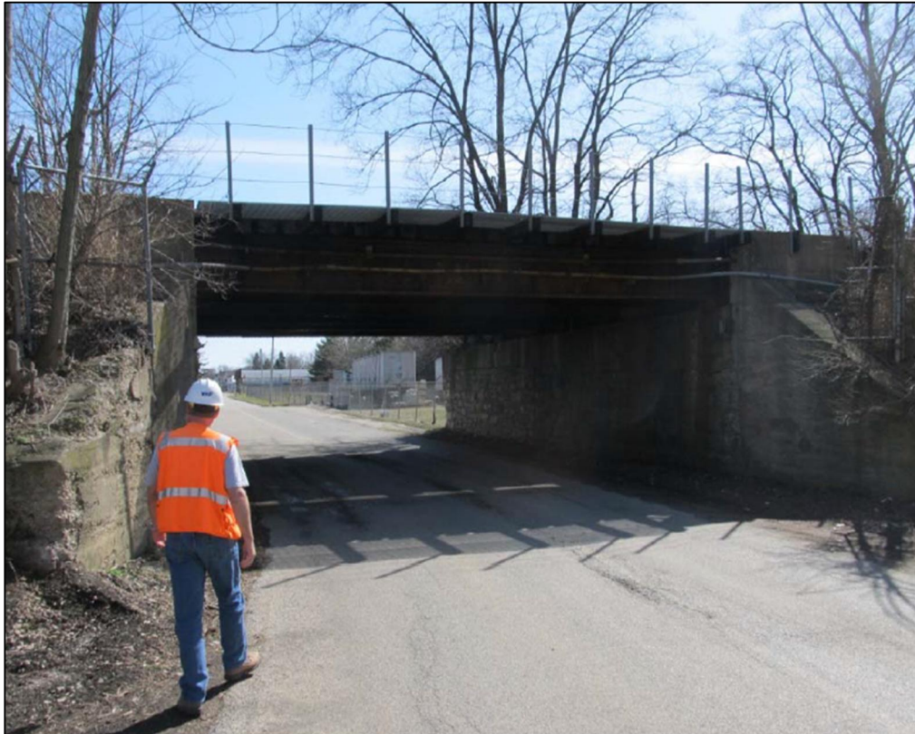
Exhibit 3-4. Water Street Bridge
