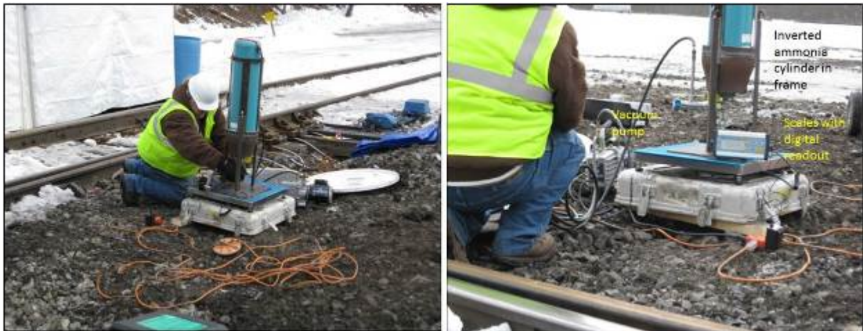
Figure 27. Charging the Heating Systems with Ammonia
