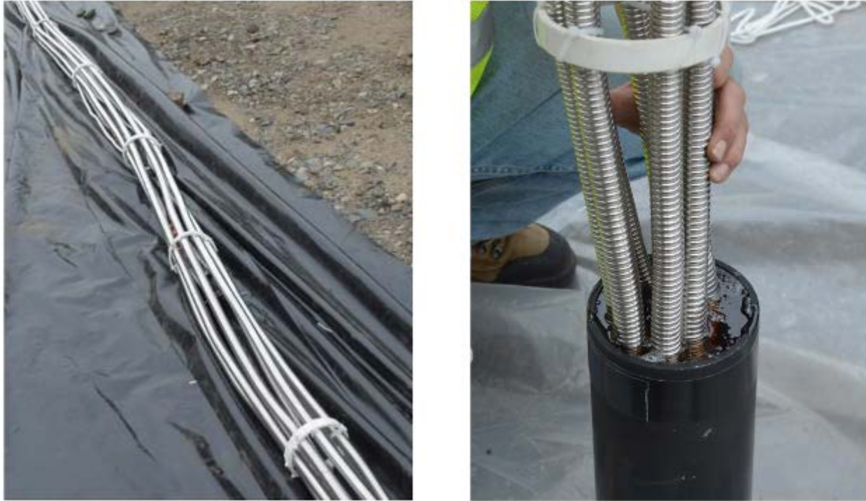
Figure 9. Tubing Preparation (left) tubing with spacers (right) epoxying the tubing
