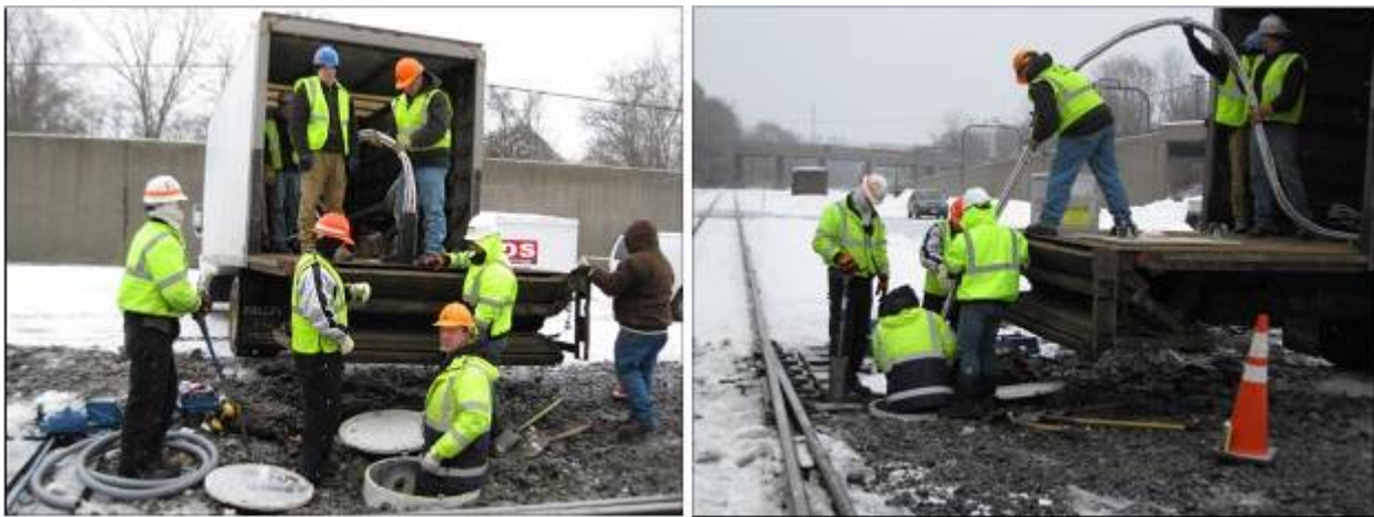
Figure 22. Installing Refrigerant Tubing into Well 2
