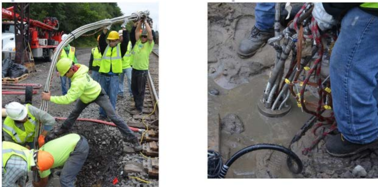
Figure 11. Insertion of Tubing into Well 1 (second successful attempt)
