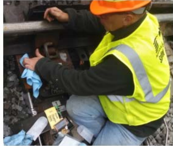
Figure 18. Preparation of Signal Wire and Installation of Switch Plate Thermocouples
