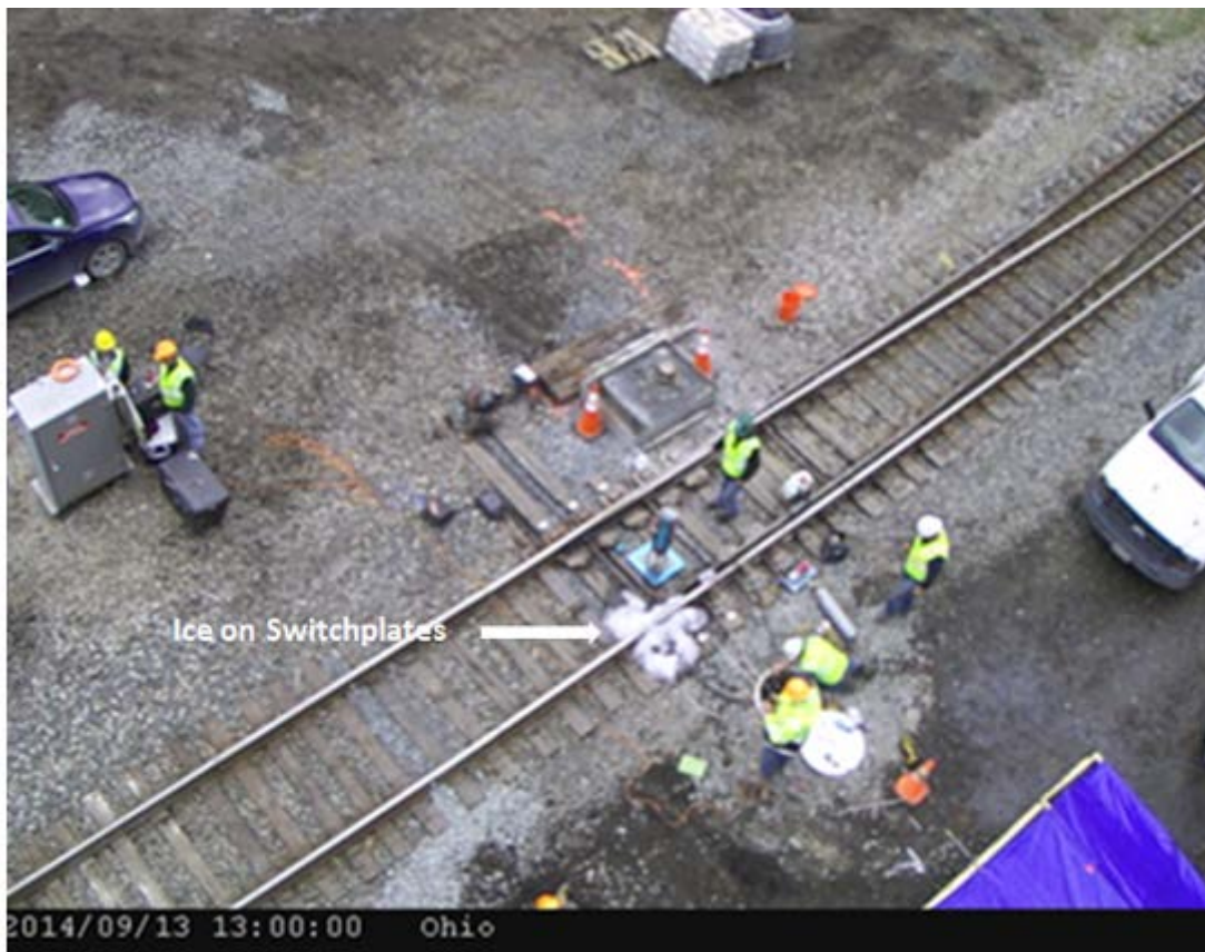
Figure 19. Overhead View of Initial Ice Melt Test
