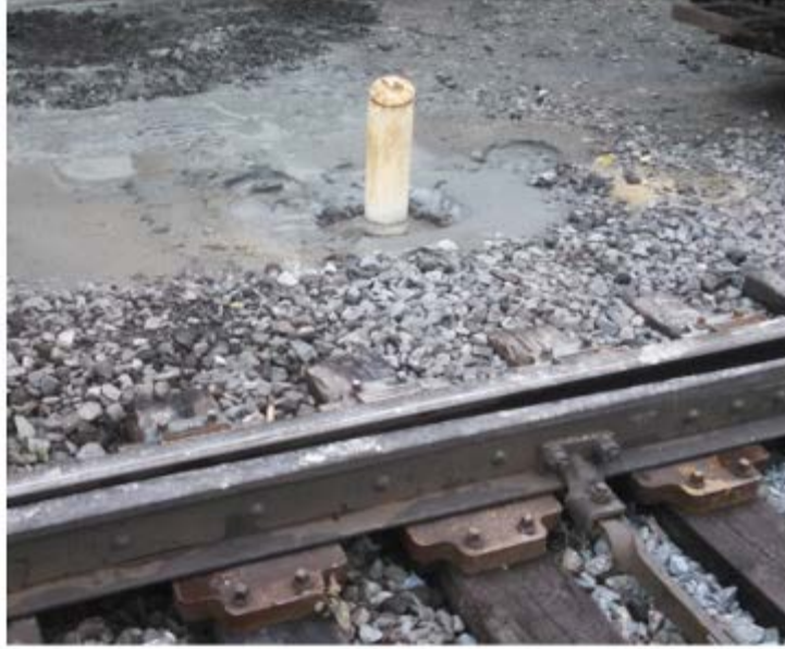
Figure 7. Bore Hole 1 Completed (casing riser was cut off before tubing installed)
