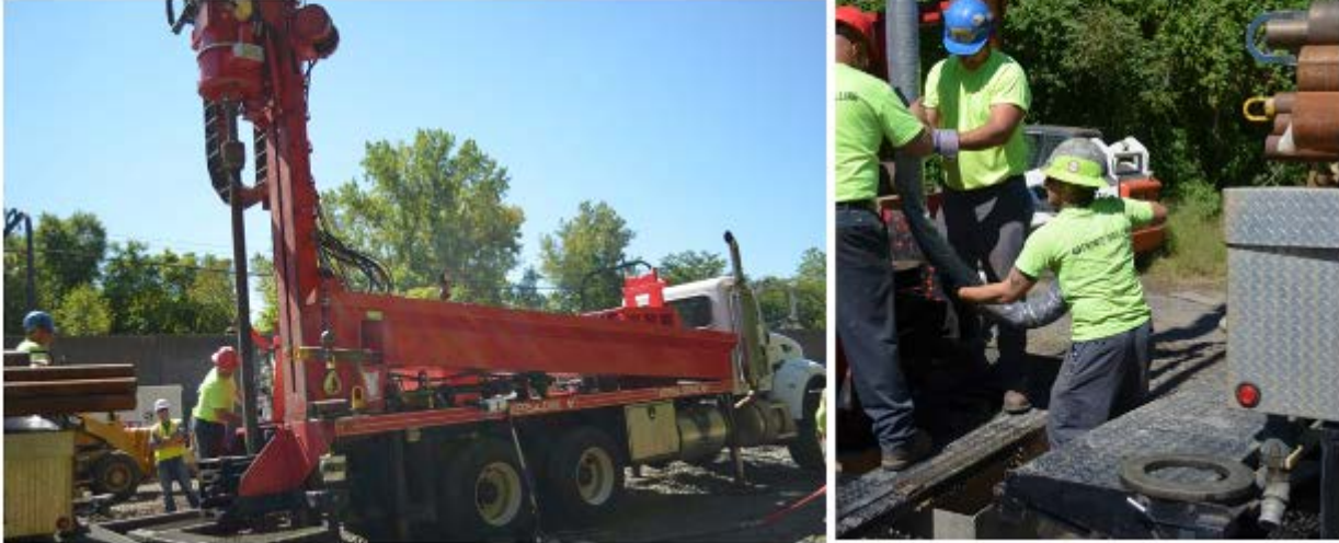
Figure 5. Drilling and Sampling Well 1
