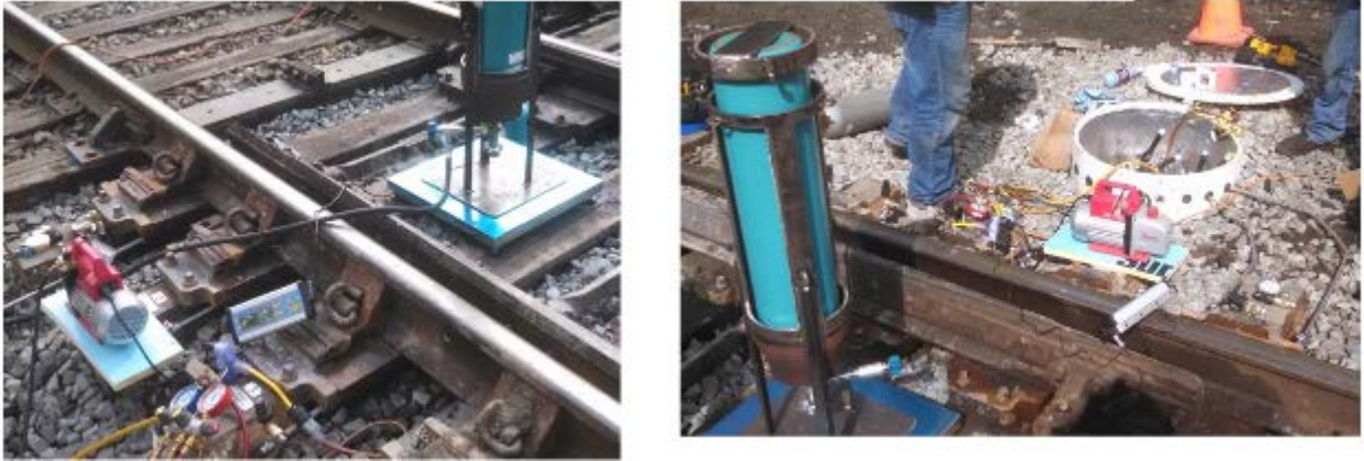
Figure 16. Filling the Refrigeration Systems
