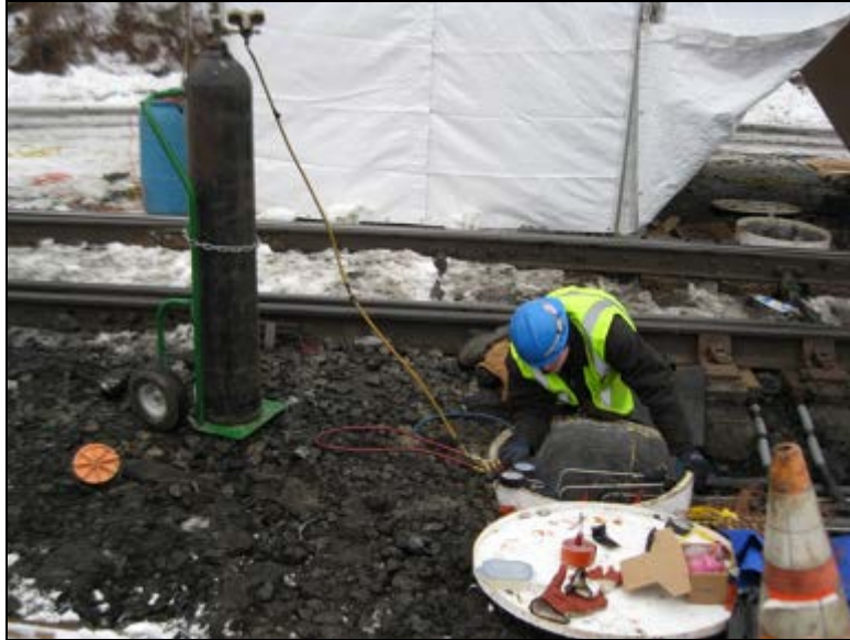
Figure 26. Purging the Systems with Nitrogen
