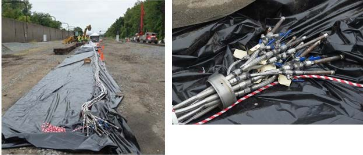
Figure 8. Tubing Layout and Assembly
