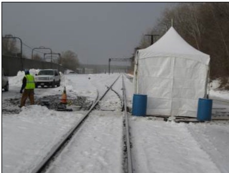
Figure 21. Phase 2 Installation of Geothermal Switch Heater
