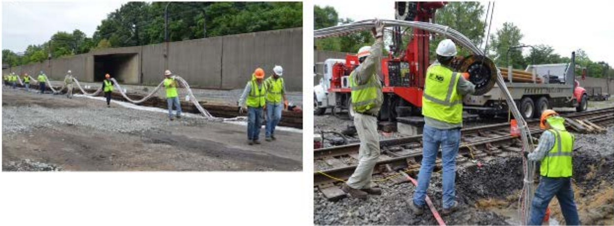
Figure 10. Tubing Placement into Well 1 (first attempt) (Note the 5-inch diameter white spacers)
