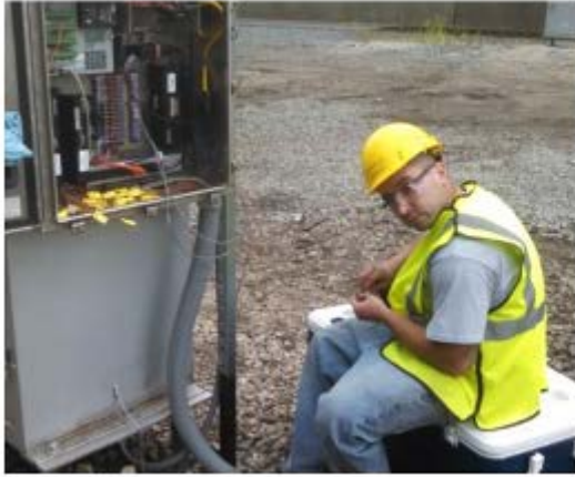
Figure 18. Preparation of Signal Wire and Installation of Switch Plate Thermocouples
