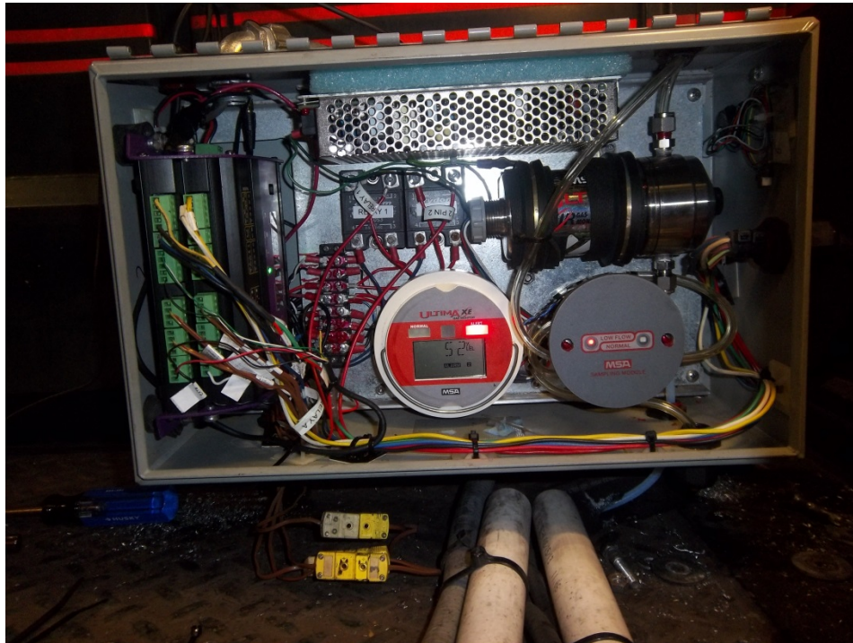
Figure 27. Powered electronics control box following maintenance at Glendive
