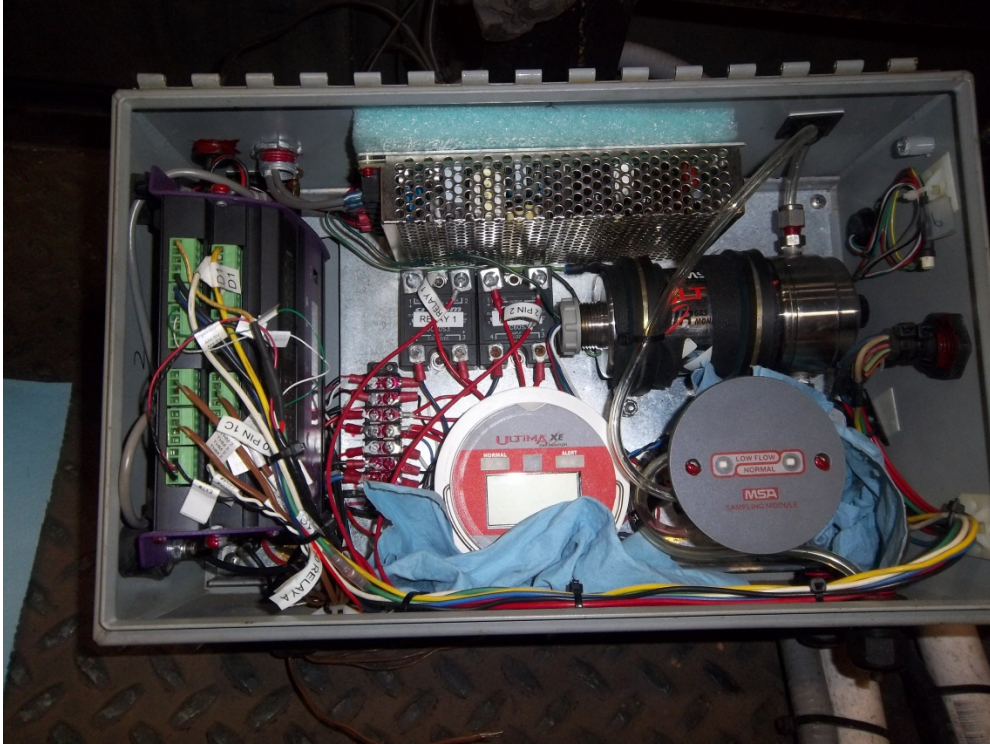
Figure 23. Water clean-up of the electronics control box at Glendive
