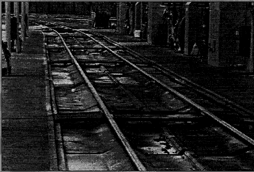
Figure 3: Track pan catchment system for oil and fuel drips
