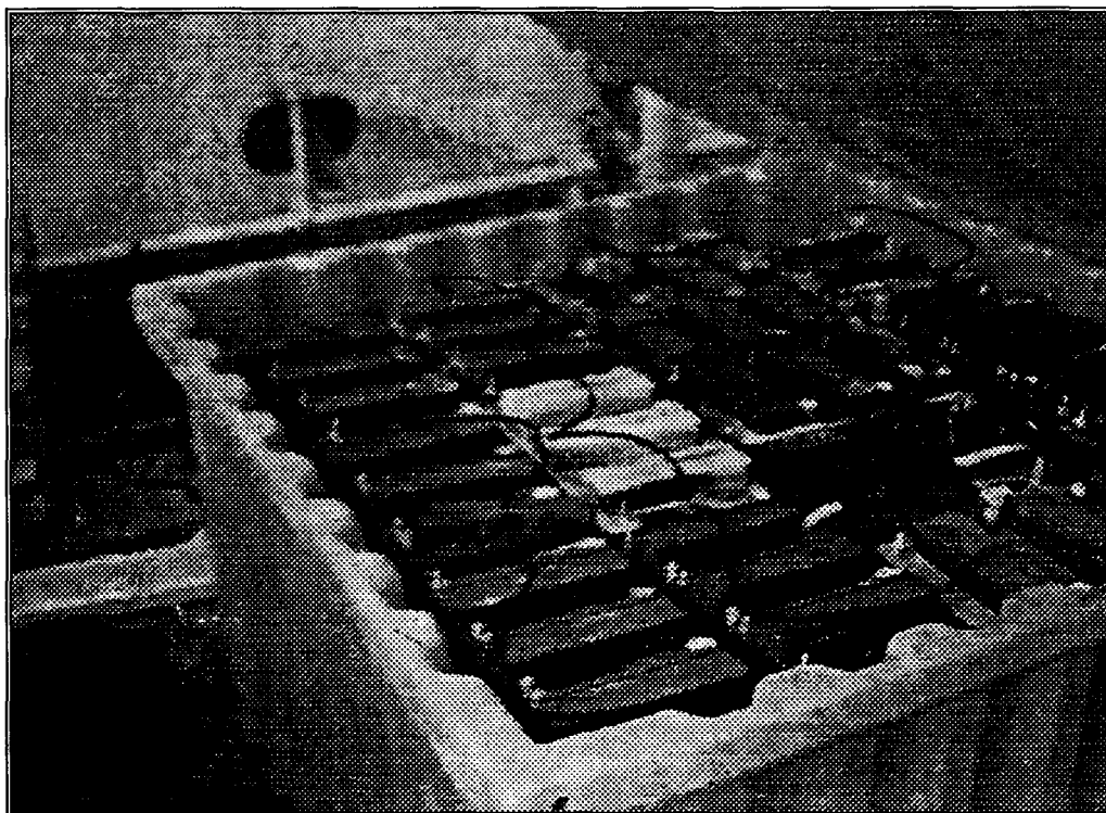
Figure 2: Properly Stored Batteries
