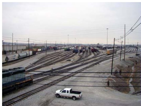
Figure 1. Railroad classification (switching) yard
