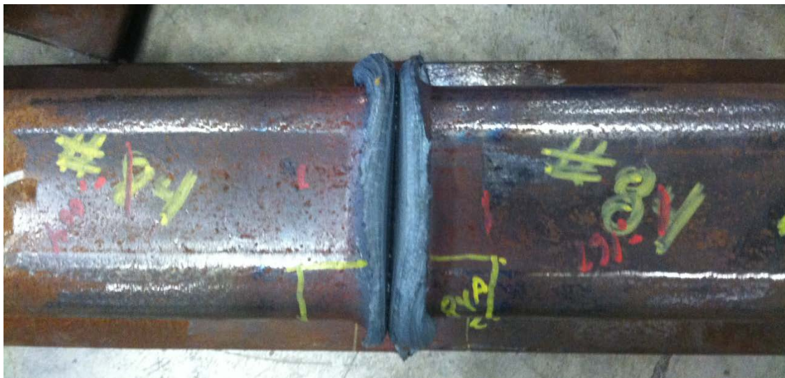
Figure 14. Weld No. 84 Viewed from above (note uniform flash curl)
