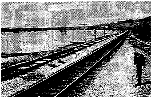
Fig. 11. Test site at Sabot, Virginia looking west.
