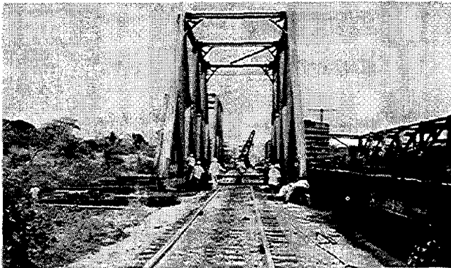
Fig. 8. New trusses for bridge over Cotaxtla River.
