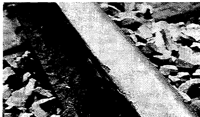
Fig. 2. Shelly rail - after less than 150 million gross tons of traffic.
