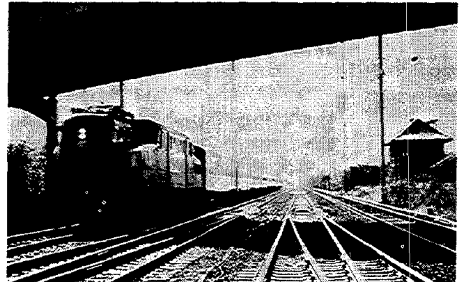
Fig. 25. Midway interlocking test site for AMTRAK track response measurements.
