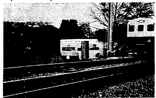
Fig. 10. Track response measurement setup on NEC track near Bowie, MD.
