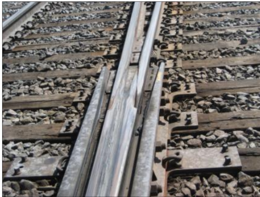
Figure 7. Multi-Tie Plate for Frog Heels
