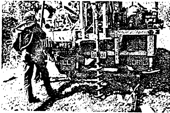
Fig. 17. Drilling in progress.
