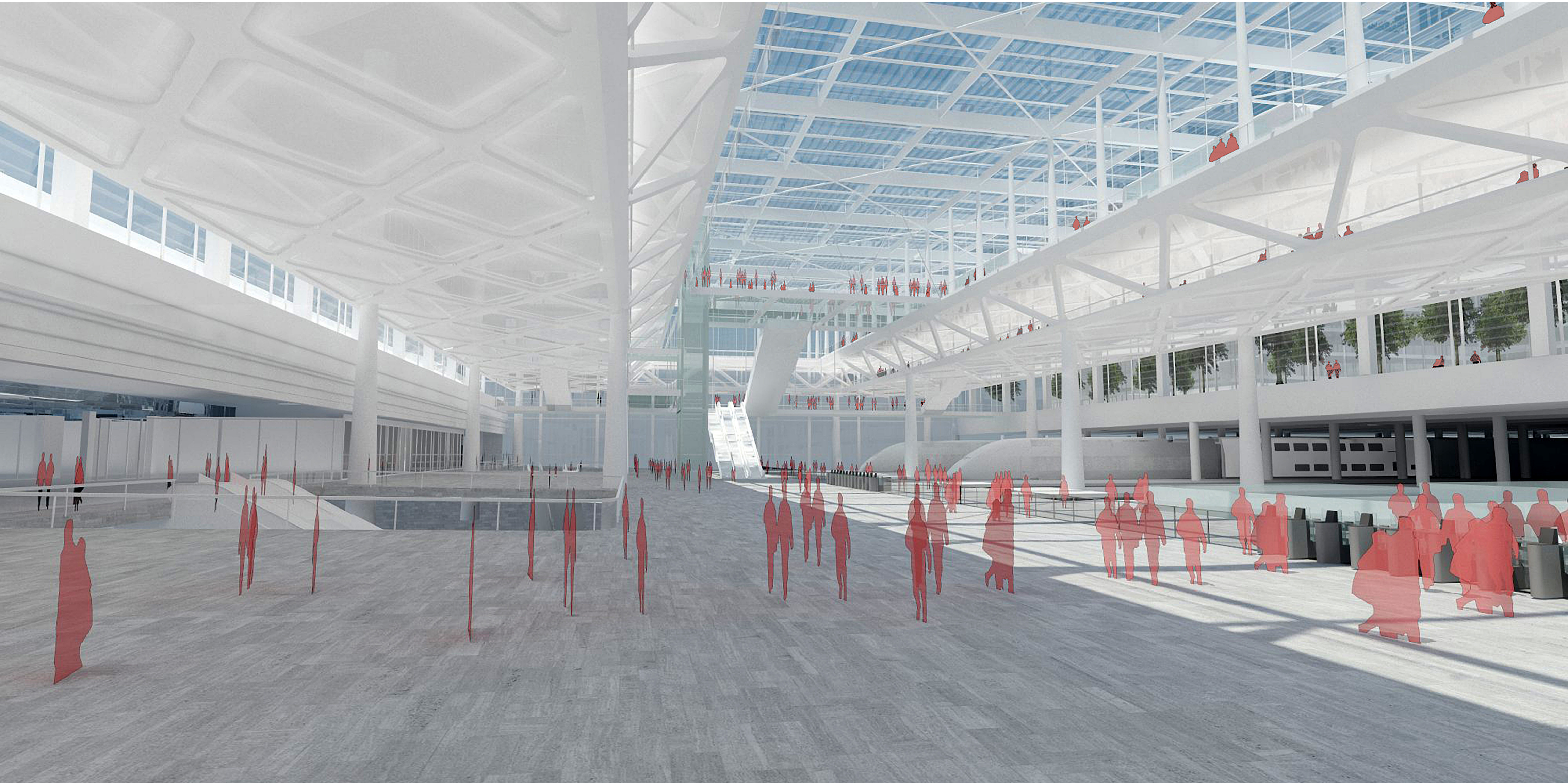
1 EAST-WEST TRAIN HALL WITH BUS ABOVE VIEW LOOKING NORTHWEST FROM MAIN/PLATFORM LEVEL
