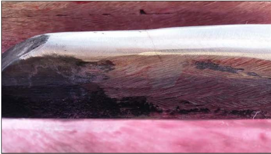
Figure 4. Frog 1: Transverse crack near the point of the frog visible with dye penetrant
