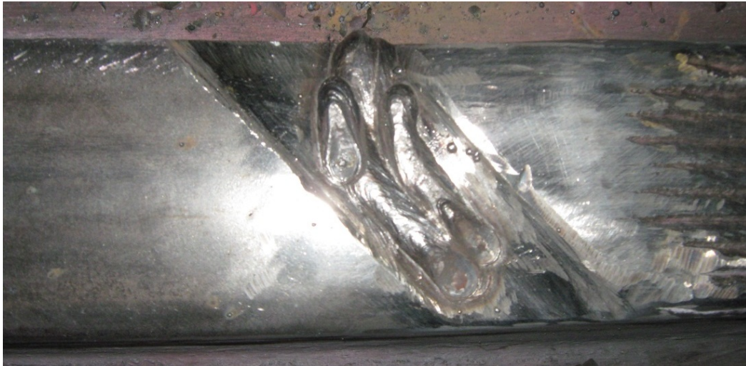
Figure 45: Filling of Cracks in Frog #1
