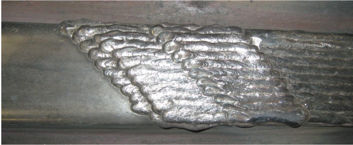
Figure 47: Weld Build-up to Complete Frog #1 Crack Repair
