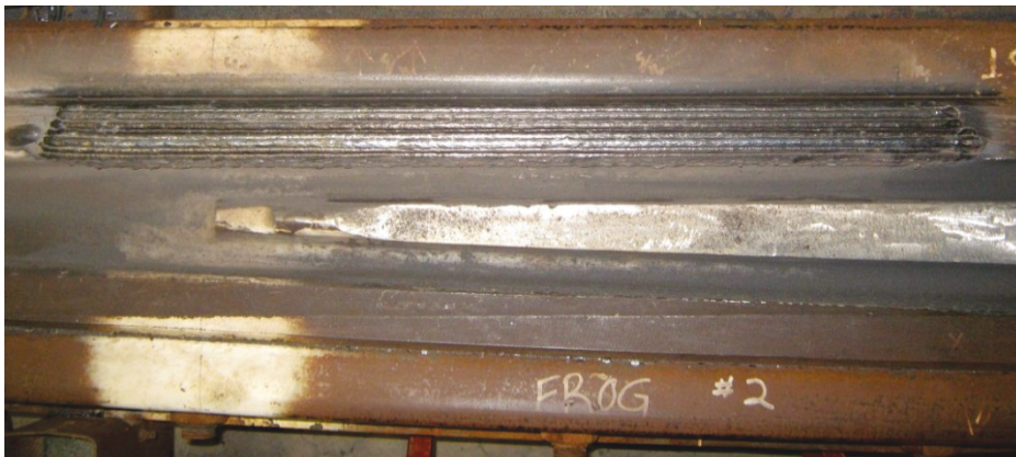
Figure 51: Frog #2 After Wing Repair
