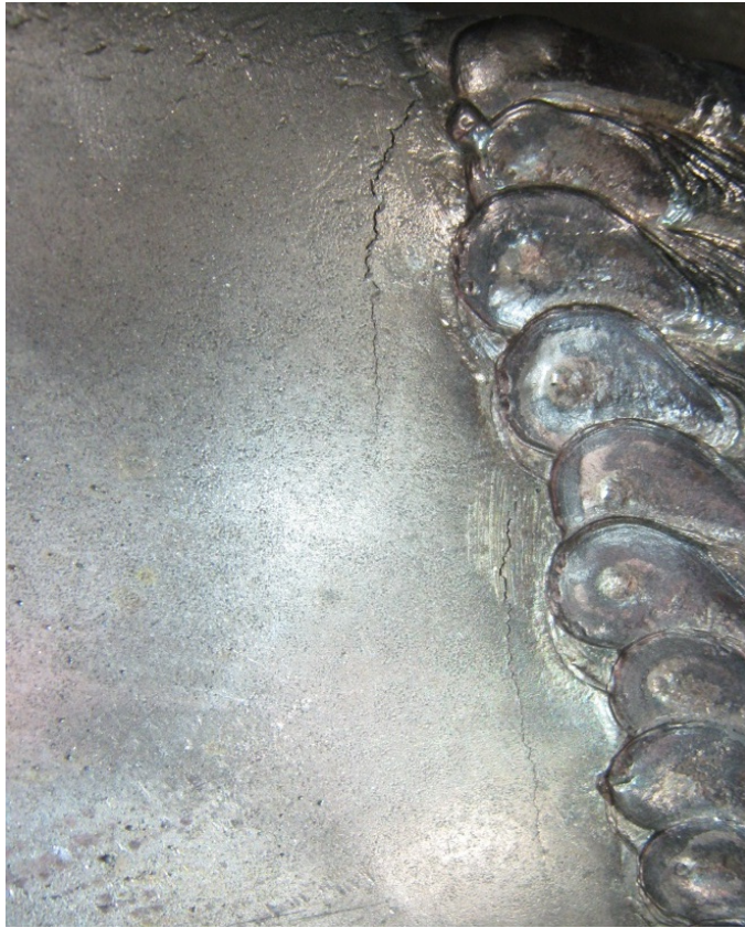
Figure 43: Base Material Cracking in Frog #1 at Interface with “Transition” Build-up
