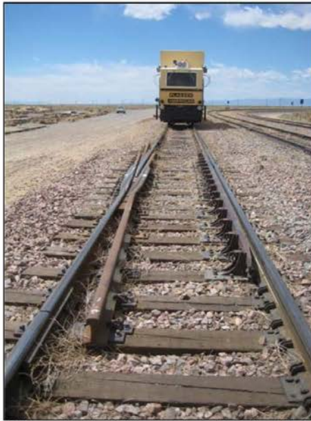
Figure 5. Frog 2 installed in Section 27 of the High Tonnage Loop
