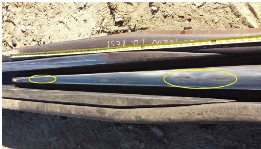
Figure 64: Point Running Surface Spalls
