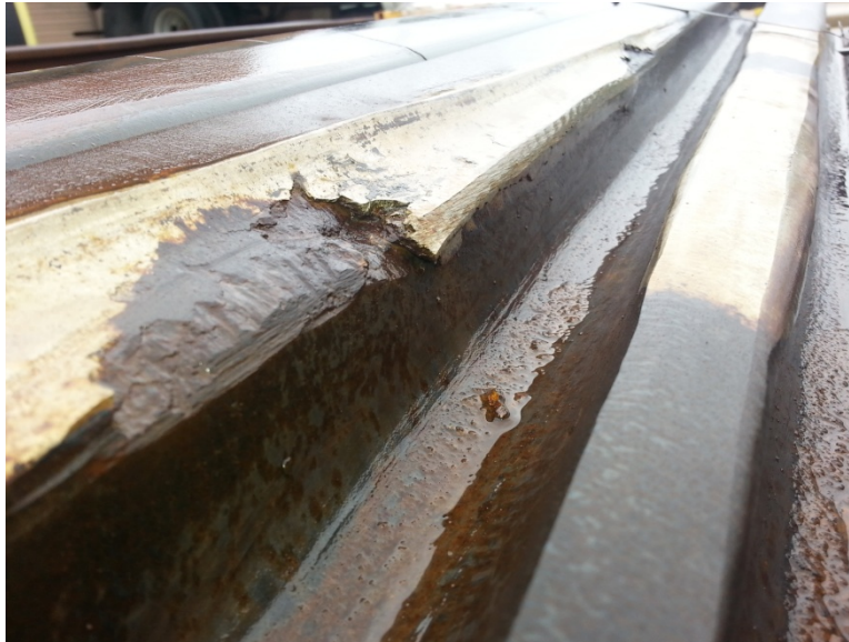
Figure 1: Breakout of Weld Repair
