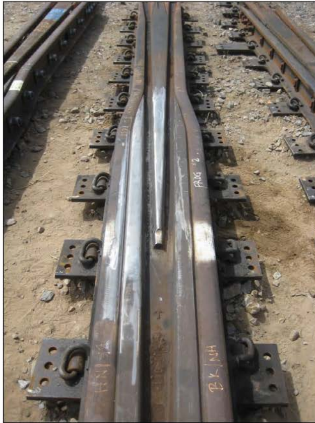
Figure 3. Weld repaired Frog 2 after grinding excess weld material
