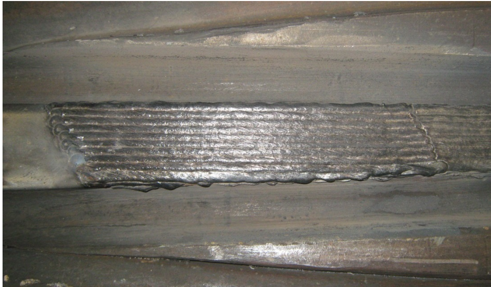
Figure 42: Frog #1 After Additional “Taper” Weld Build-up
