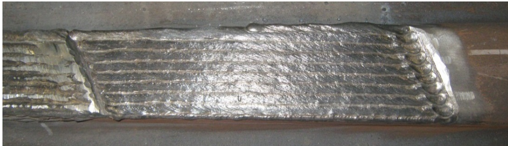
Figure 53: Layer 1 Welding of Frog #2 Transition Area
