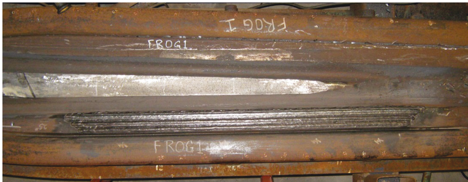
Figure 41: Frog #1 After Wing Repair
