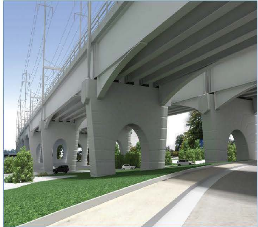
Key Hole Pier Design
