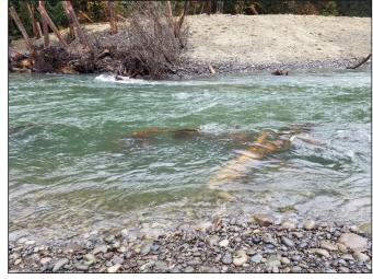
▶ Bags were used to divert water so fill could be placed in slow water areas to allow reshaping of the island.
