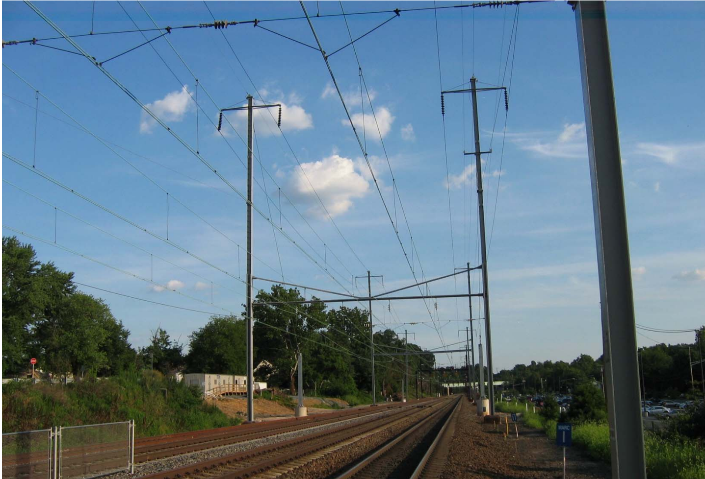
Similar Structures on Amtrak Northeast Corridor near Halethorpe Maryland
