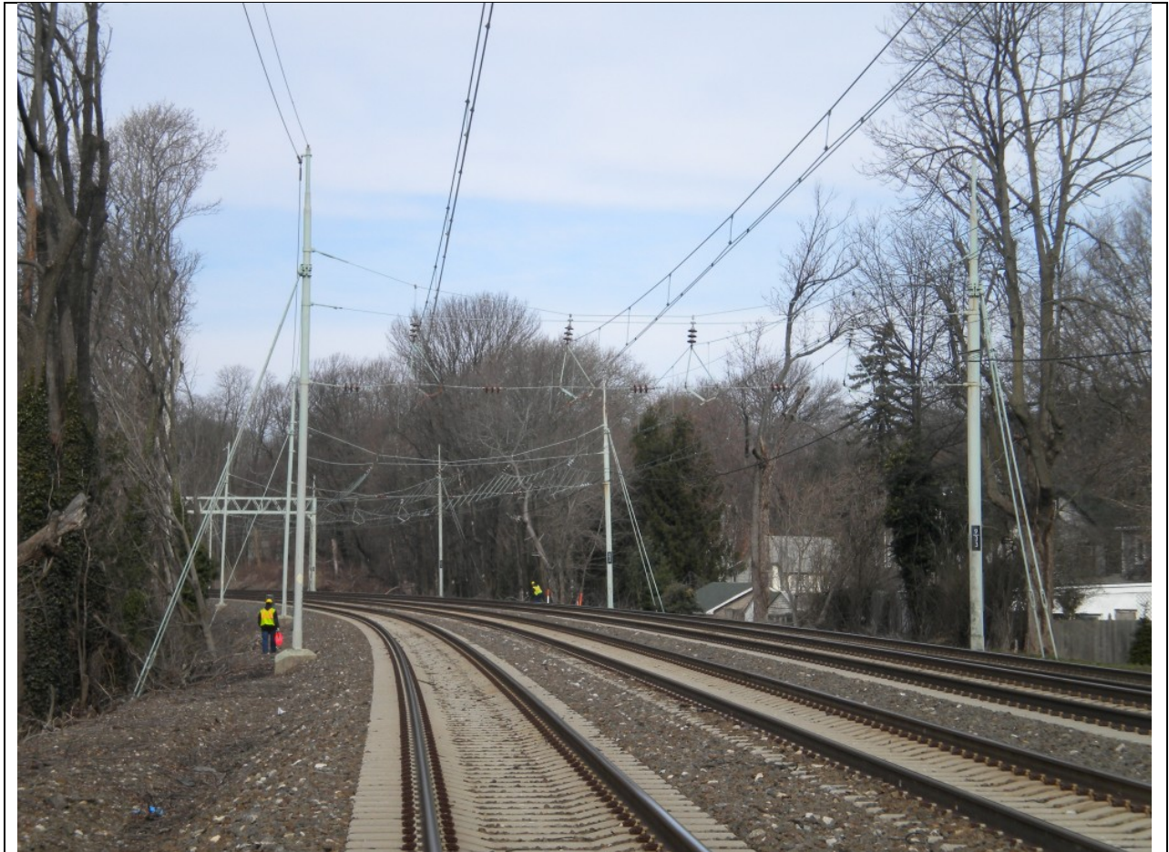
Photograph 8: Harrisburg Line, milepost 9.33, west of Haverford, looking west at existing structure P-80. HSHD is on both sides, north (right) and south (left) of the railroad. Photograph taken 12/5/2012.
