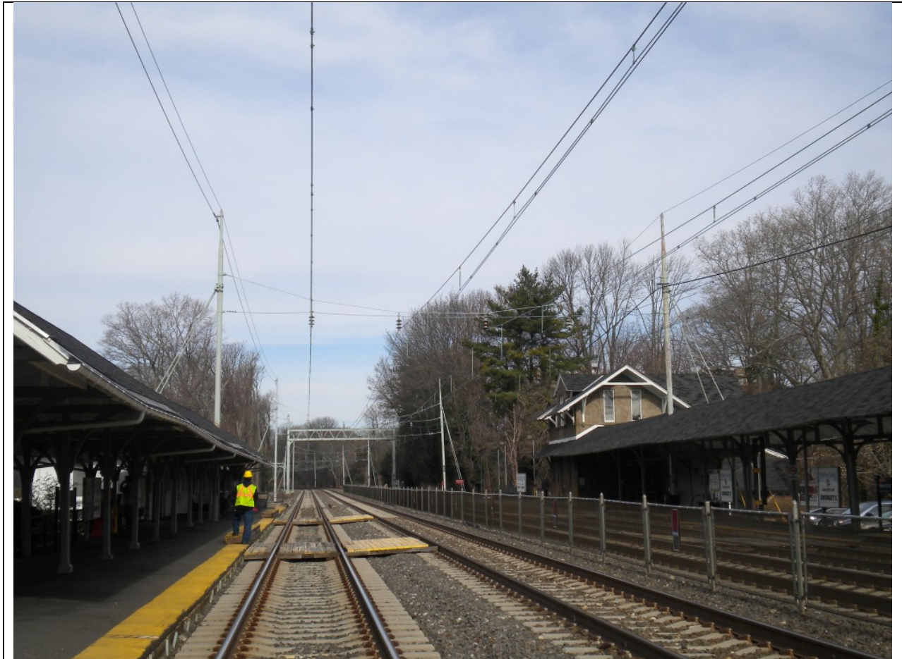
Photograph 11: Harrisburg Line, milepost 9.16, west of Haverford, looking west at existing structure P-77. Haverford Station Road passes under the railroad between this structure and the next one in the distance. HSHD is on both sides, north (right) and south (left) of the railroad. Photograph taken 12/5/2012.
