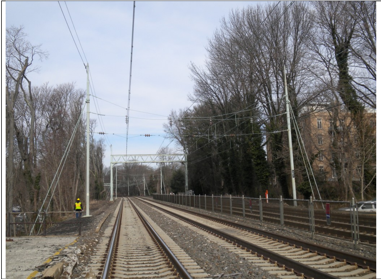
Photograph 10: Harrisburg Line, milepost 9.22, west of Haverford, looking west at existing structure P-78. HSHD is on both sides, north (right) and south (left) of the railroad. Photograph taken 12/5/2012.
