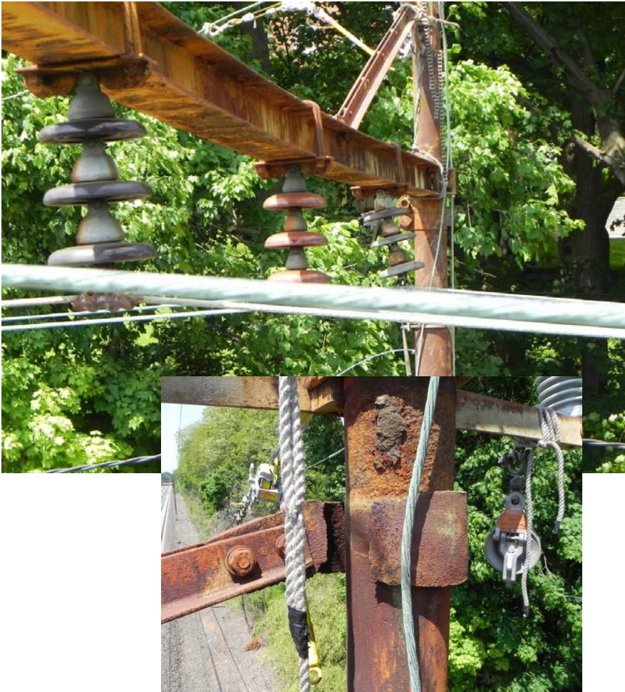
Beam failure (St. Davids), Foundation deterioration
