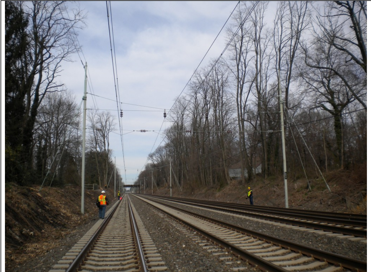
Photograph 4: Harrisburg Line, milepost 9.56, west of Haverford, looking west at existing structure P-84. Pennswood Road Bridge is in the background. HSHD is on the left, the south side of the railroad.. Photograph taken 12/5/2012.
