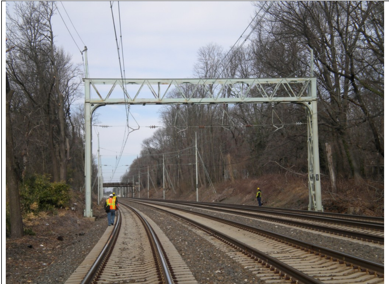
Photograph 5: Harrisburg Line, milepost 9.50, west of Haverford, looking west at existing structure P-83. HSHD is on the left, the south side of the railroad.. Photograph taken 12/5/2012.
