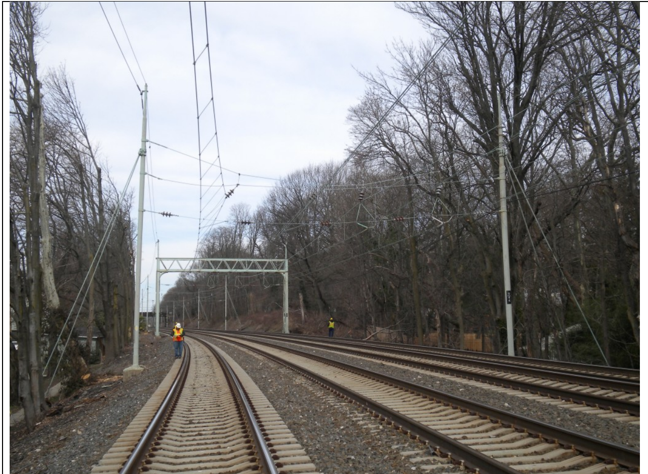
Photograph 6: Harrisburg Line, milepost 9.45, west of Haverford, looking west at existing structure P-82. HSHD is on both sides, north (right) and south (left) of the railroad. Photograph taken 12/5/2012.
