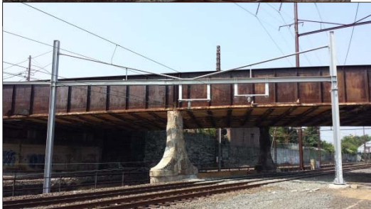
Unpainted galvanized steel
