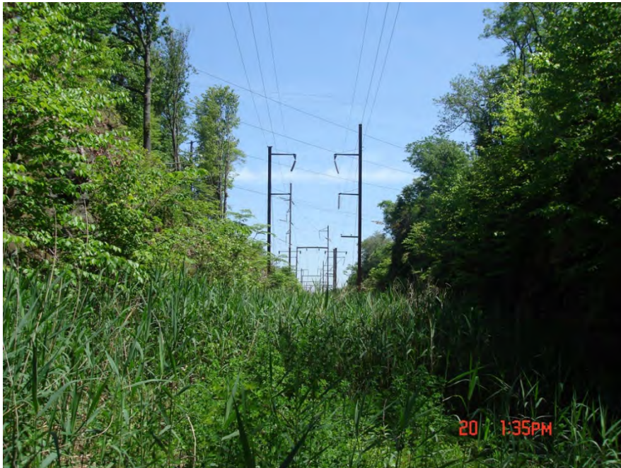
Figure 1 - Existing Transmission Right of Way
