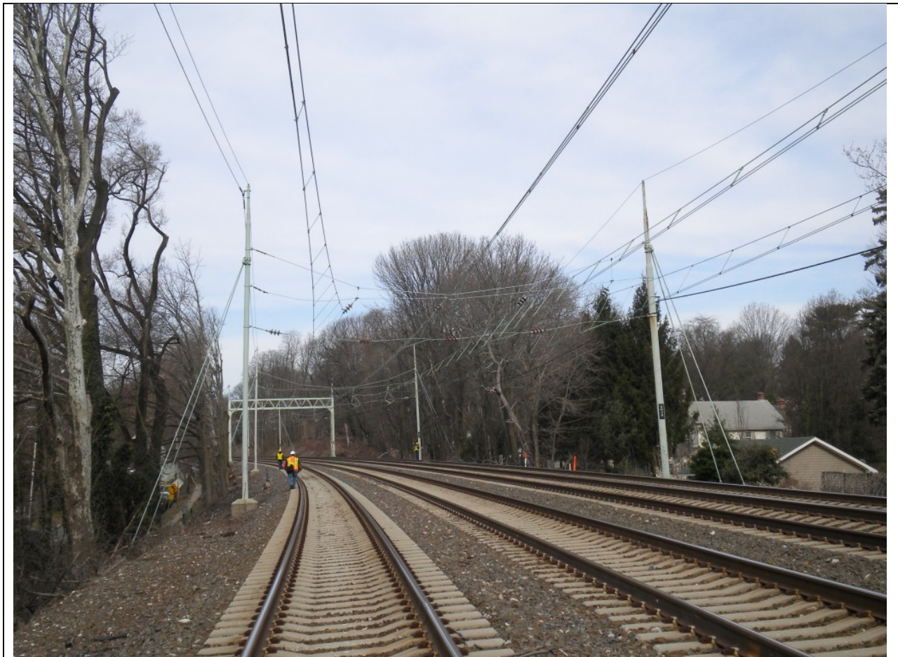
Photograph 7: Harrisburg Line, milepost 9.39, west of Haverford, looking west at existing structure P-81. Booth Lane passes under the railroad between this structure and the next one in the distance. HSHD is on both sides, north (right) and south (left) of the railroad. Photograph taken 12/5/2012.
