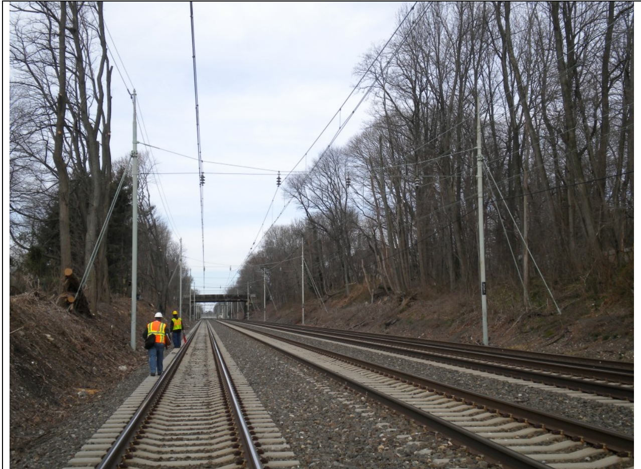
Photograph 3: Harrisburg Line, milepost 9.61, west of Haverford, looking west at existing structure P-85. Pennswood Road Bridge is in the background. HSHD is on the left, the south side of the railroad.. Photograph taken 12/5/2012.
