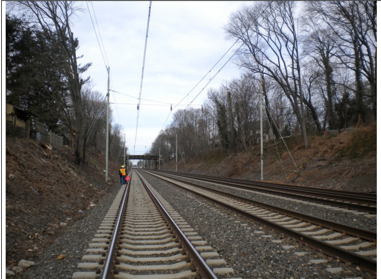
Photograph 2: Harrisburg Line, milepost 9.67, west of Haverford, looking west at existing structure P-86. Pennswood Road Bridge is in the background. HSHD is on the left, the south side of the railroad.. Photograph taken 12/5/2012.
