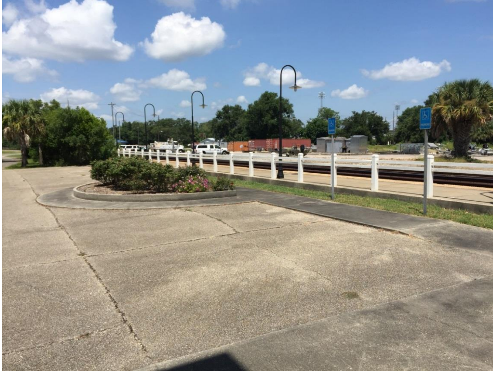
FIG BAS 01 – Cracking at parking lot, require reseal and restriping; platform lighting appears to be majority of lighting intended for parking lot
