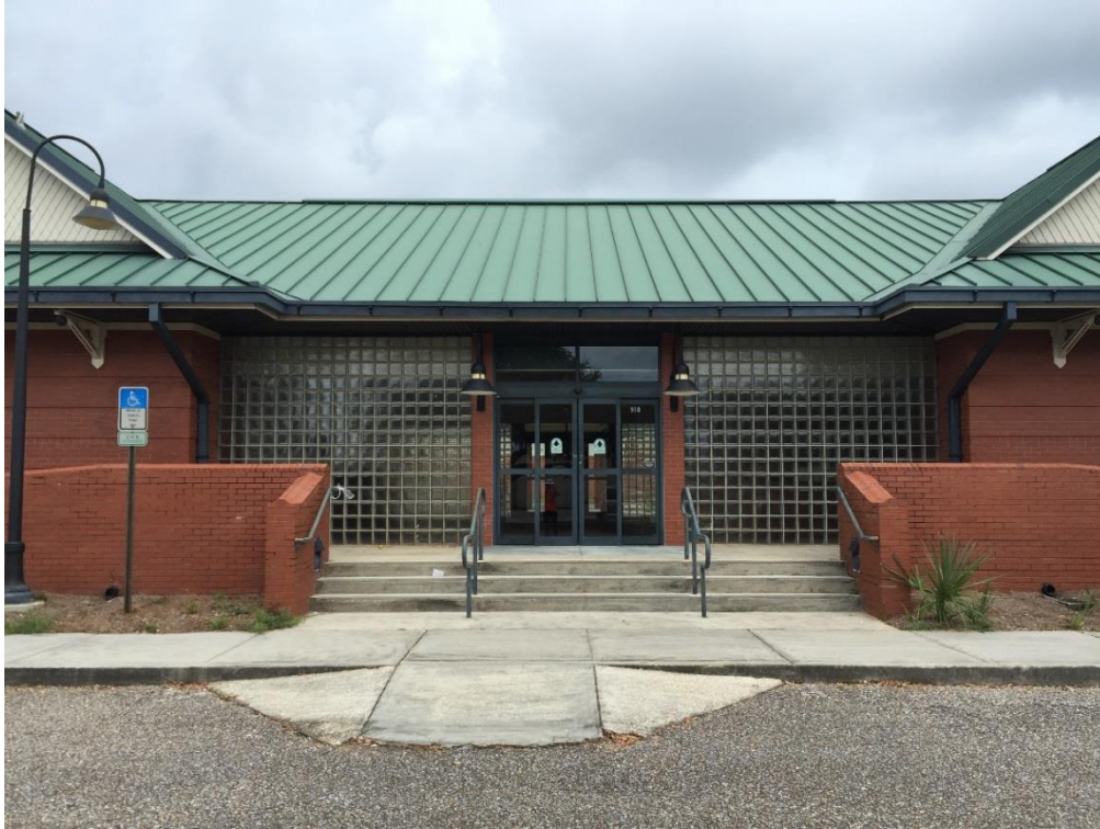
FIG PNS.07 – Stairway leading to station waiting room entrance
