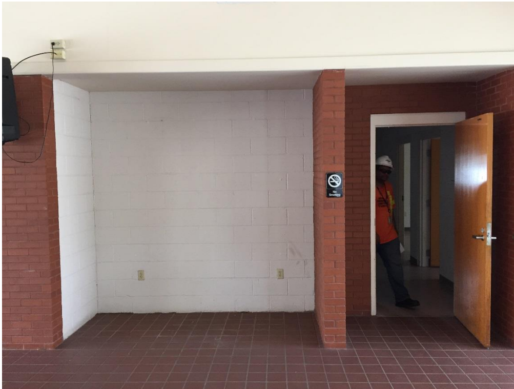
FIG PNS.20 – Interior of waiting room looking towards office area entrance door
