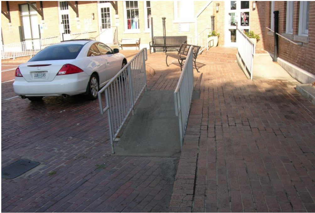
FIG GUF.07 – Access ramp #1
