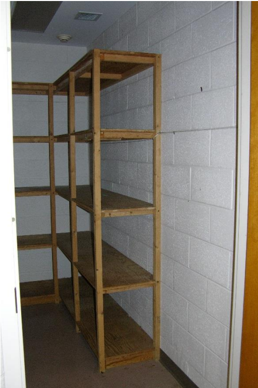
FIG PNS.31 – Baggage storage space accessible via ticket office
