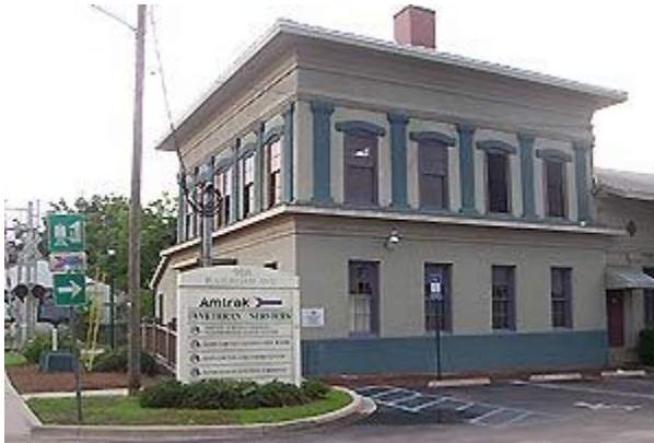
Photo of Station Shelter
