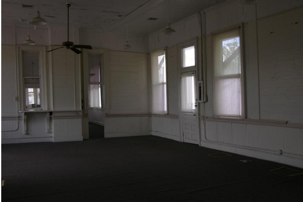
FIG PAG.11 – View from inside ticket office looking east
