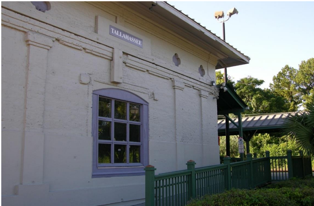
FIG TLH.54 – Westward facing wall of station building exterior
