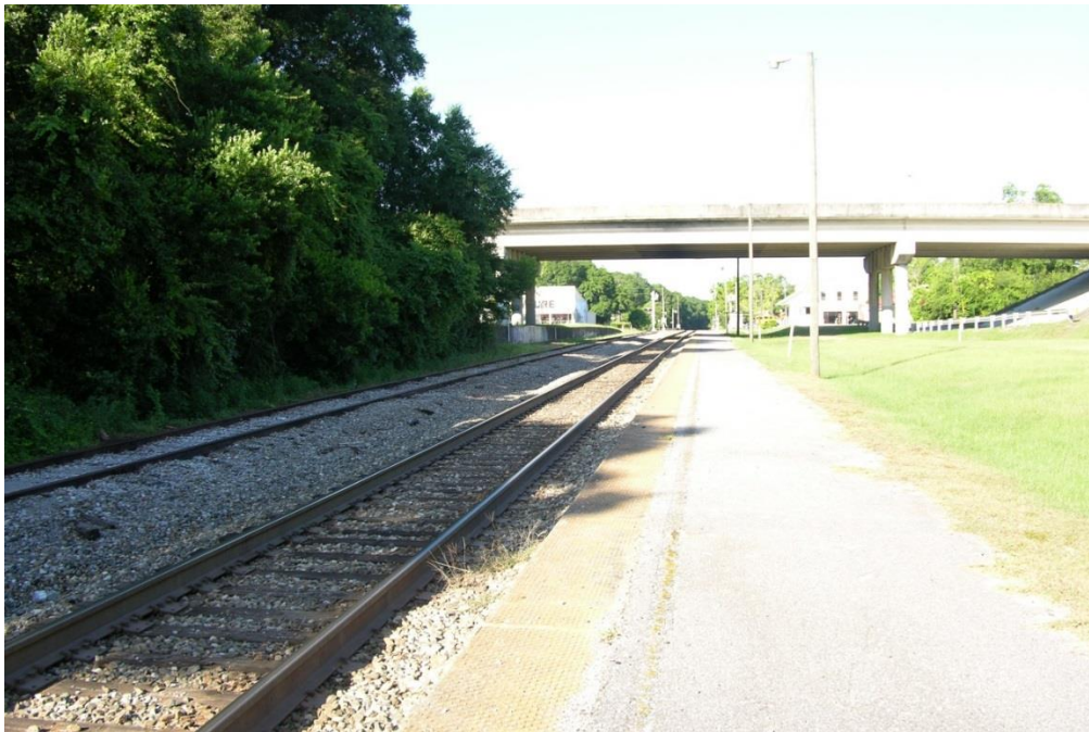
FIG CSV.04 – Platform looking southwest
