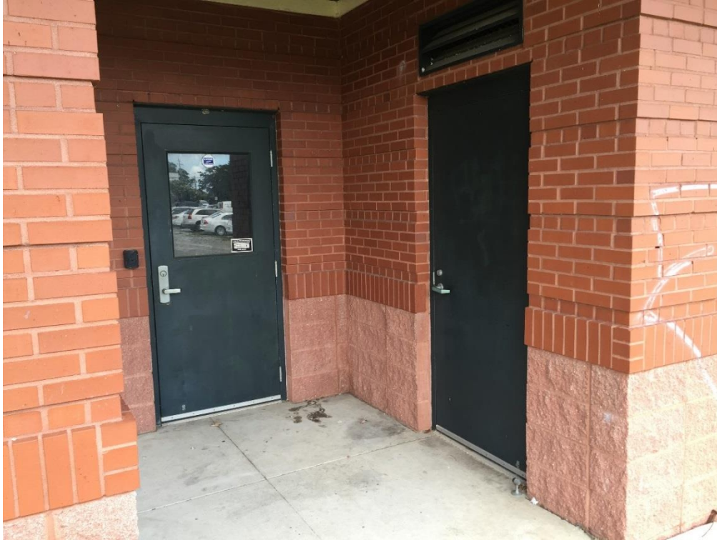
FIG PNS.39 – Side entrance on western side of the building (utility close to the right)
