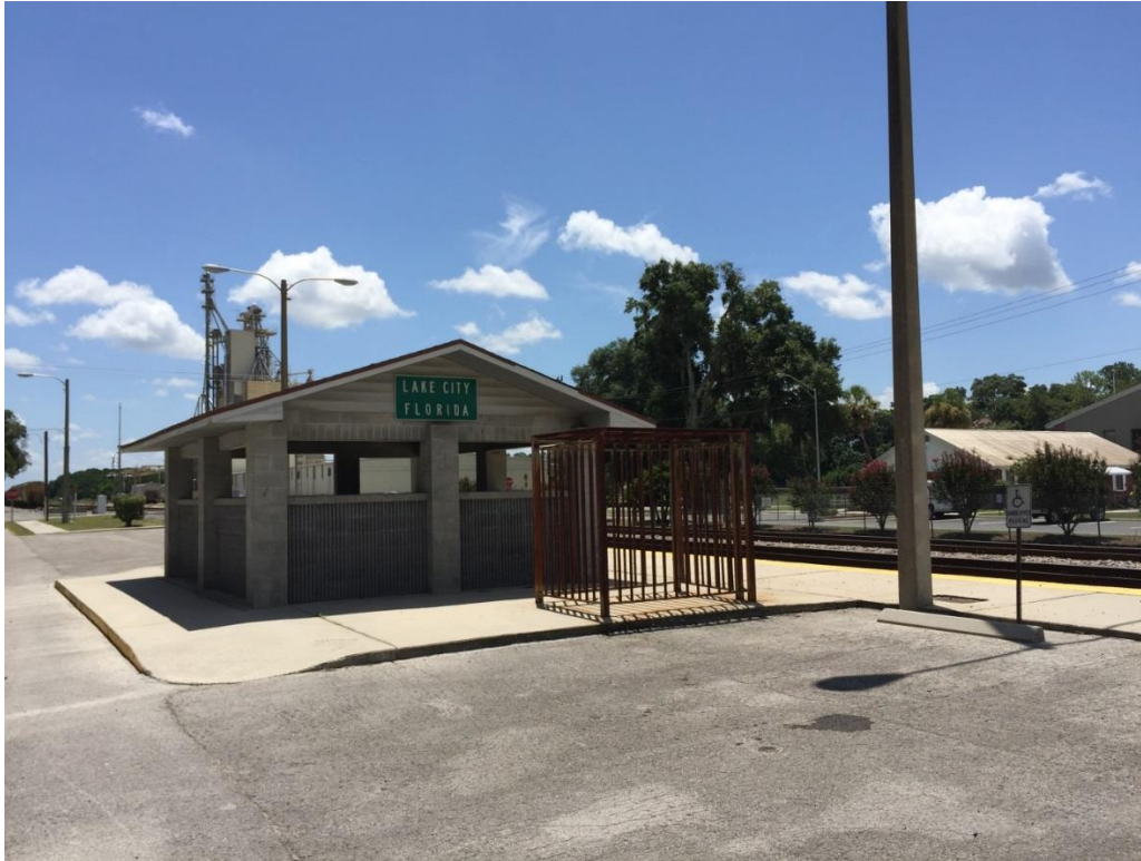
FIG LAC.19 – Overview of shelter and surrounding elements.
