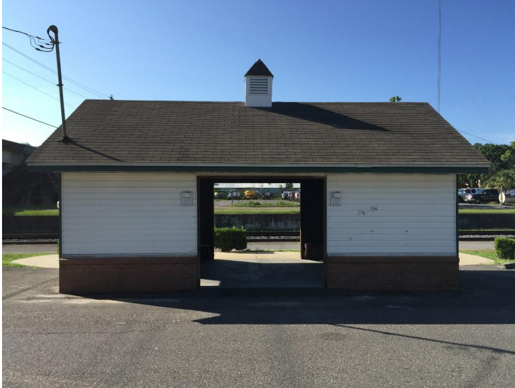
FIG CSV.17 – Roofing in adequate condition
