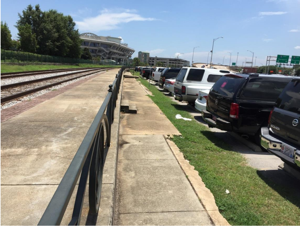
FIG MOE.01 – Adjacency of Parking Lot to platform, looking south.
