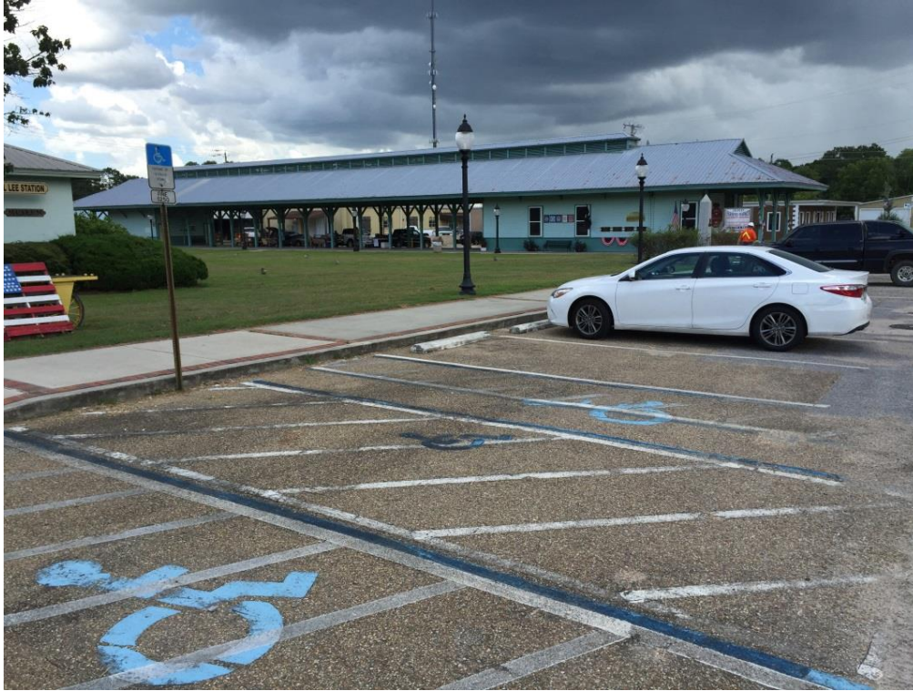
FIG CIP.19 – Accessible parking at Chipley Station
