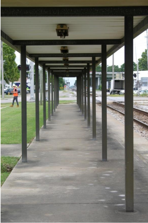
FIG BIX.05 – Platform under canopy looking west
