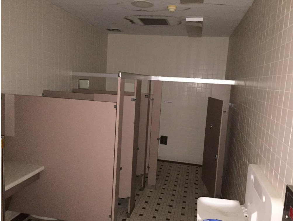
FIG PNS.35 – Women’s restroom accessible via waiting room
