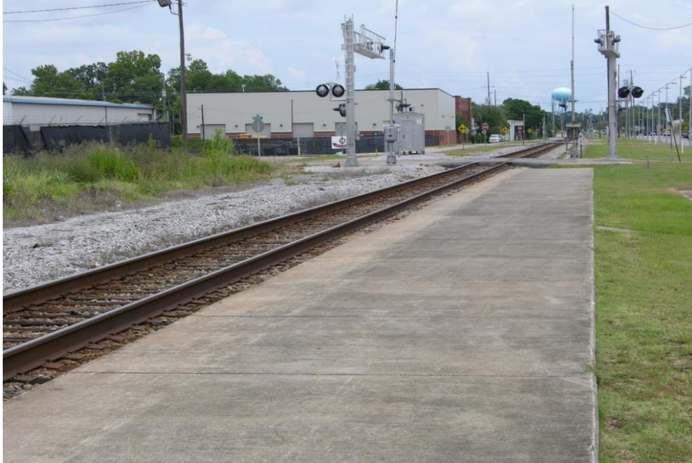
FIG BIX.01 – Platform surface looking toward grade crossing
