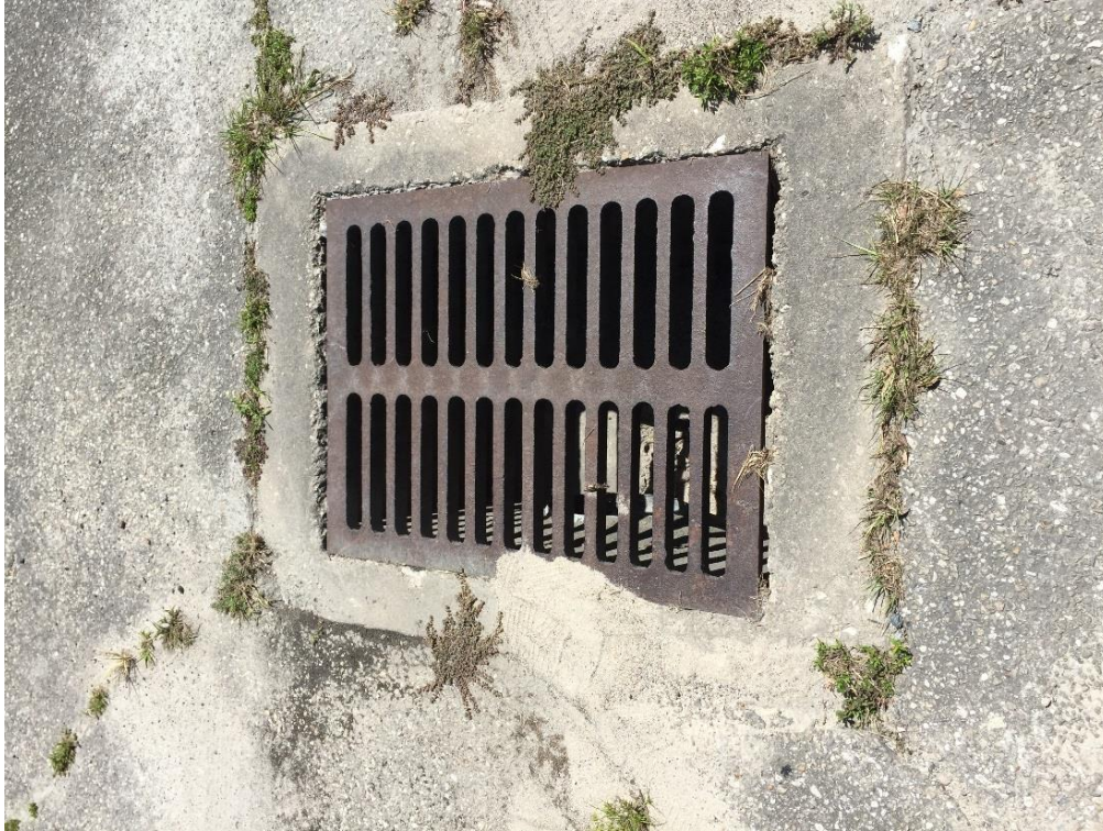
FIG MDO.09 – Close-up view of site drain shown in FIG MDO.09
