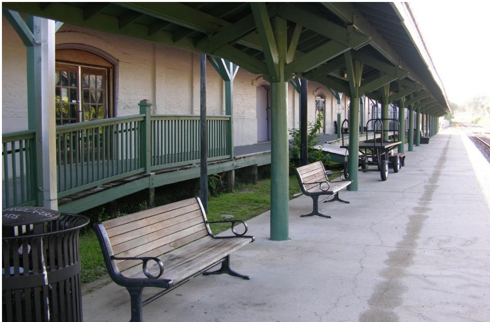
FIG TLH.52 – The double door leading from waiting to ramp connecting to platform
