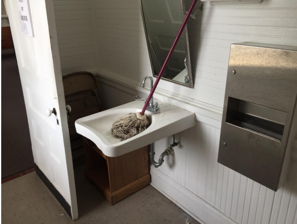
FIG PAG.15 – Sink in Men’s restroom
