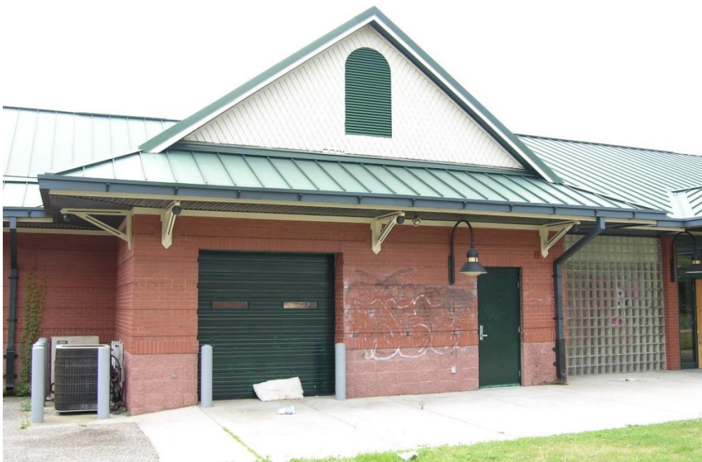
FIG PNS.40 – Back entrance to the station next to the roll up door
