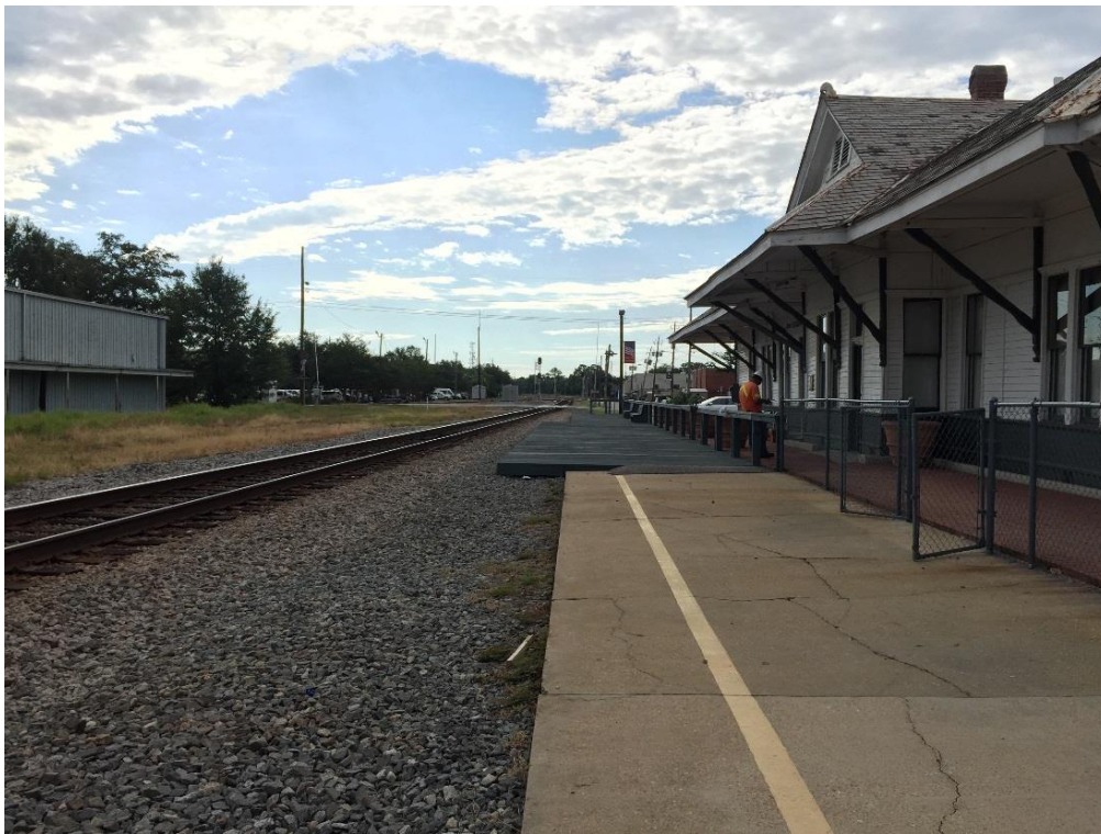
FIG PAG.08 – Platform made form dissimilar materials; building awning / canopy can be seen on the right
