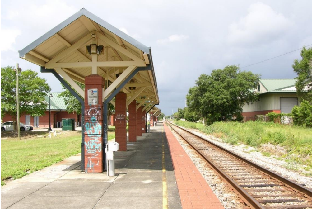
FIG PNS.17 – View from end of eastern-most canopy
