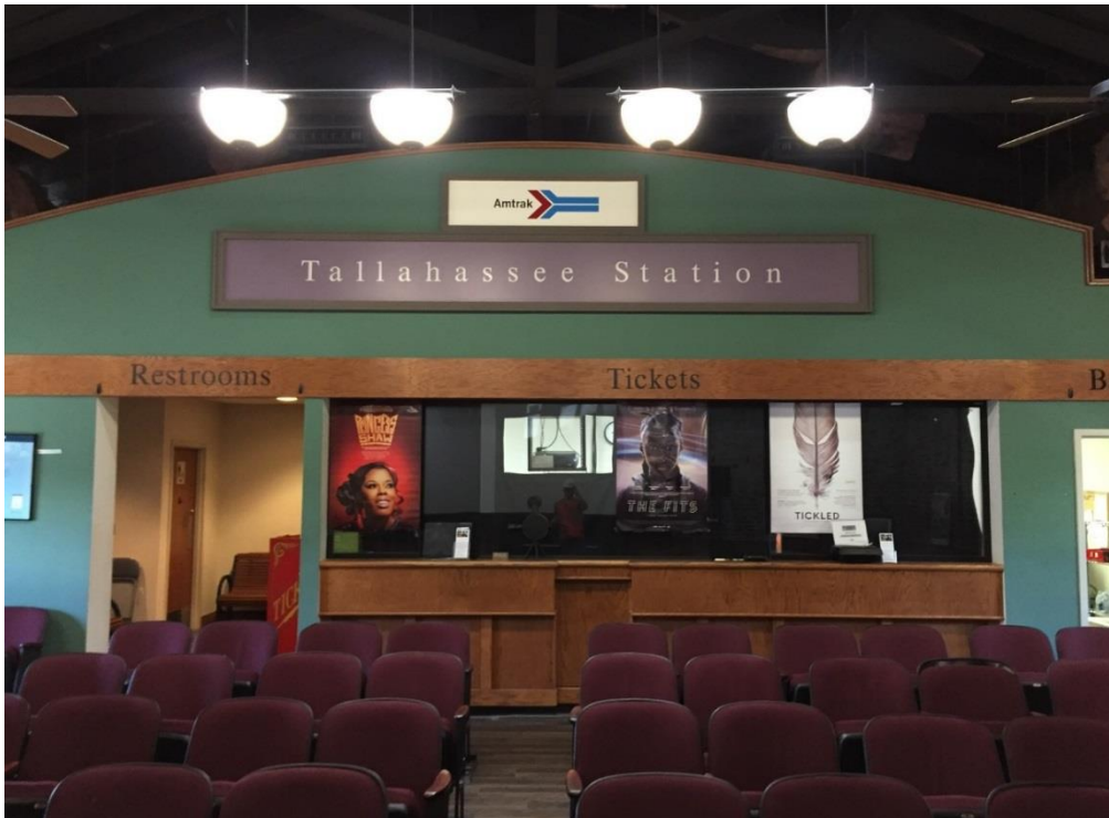
FIG TLH.36 – Outdated station interior signage
