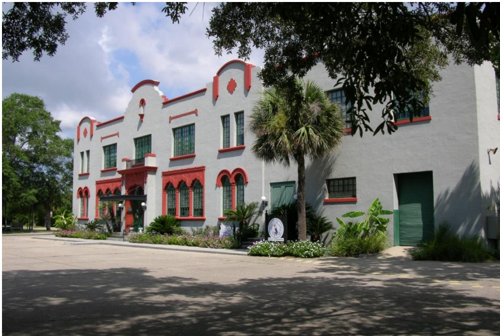
FIG BAS.06 – Historic Station Building (note roll-up door on the right)
