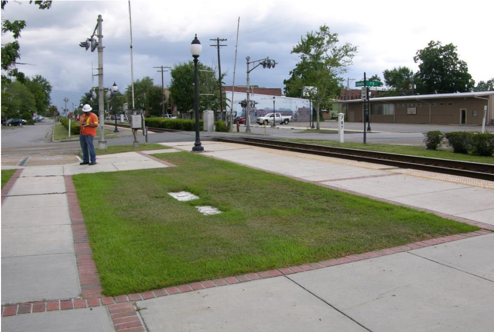
FIG CIP.06 – The sidewalk and curbs for Chipley FL station
