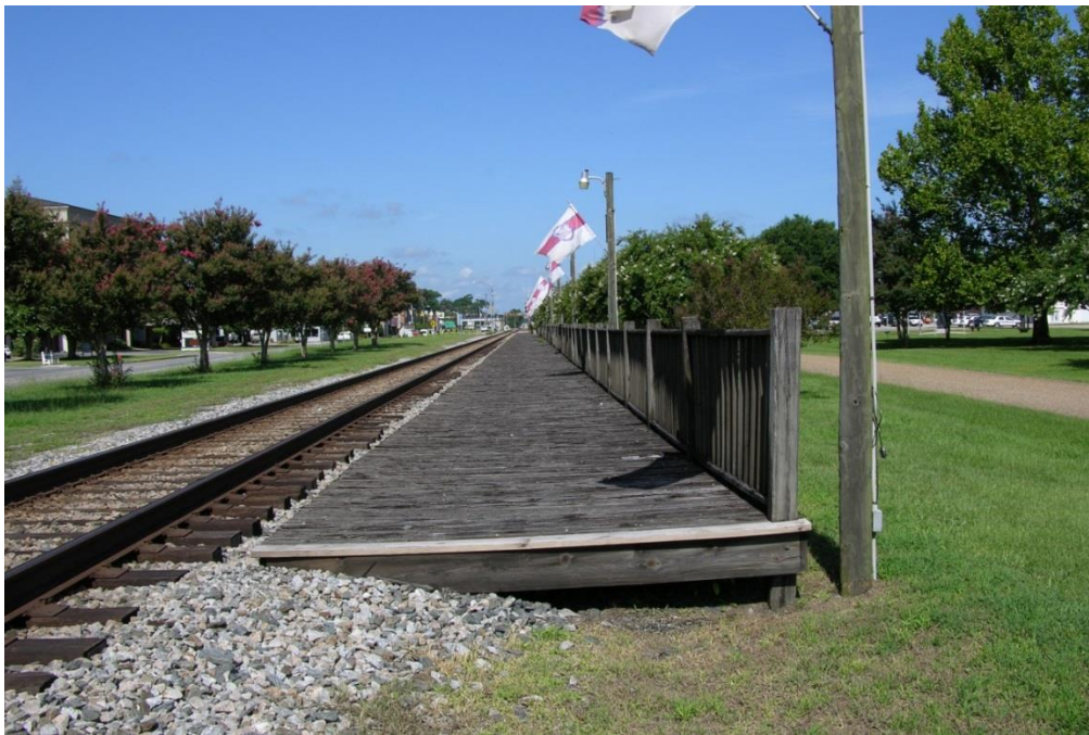
FIG ATR.08 – Existing platform – looking westward
