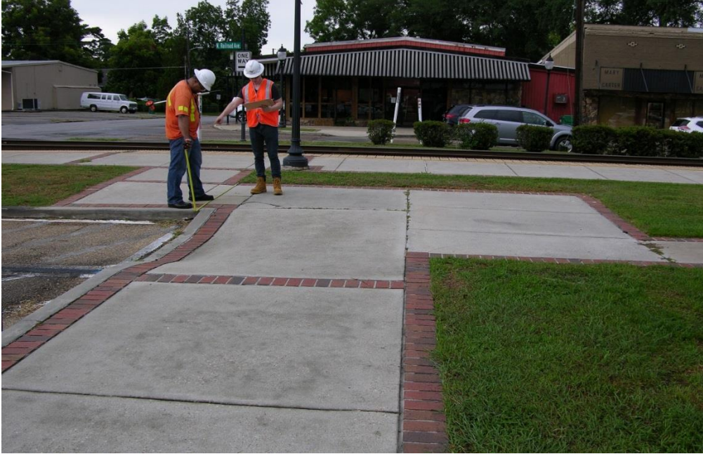
FIG CIP.05 – The sidewalk and curbs for Chipley FL station
