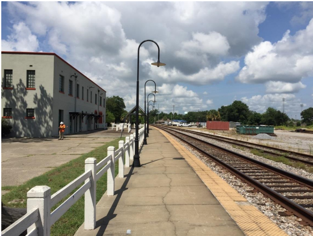
FIG BAS.02 – Platform in adequate condition
