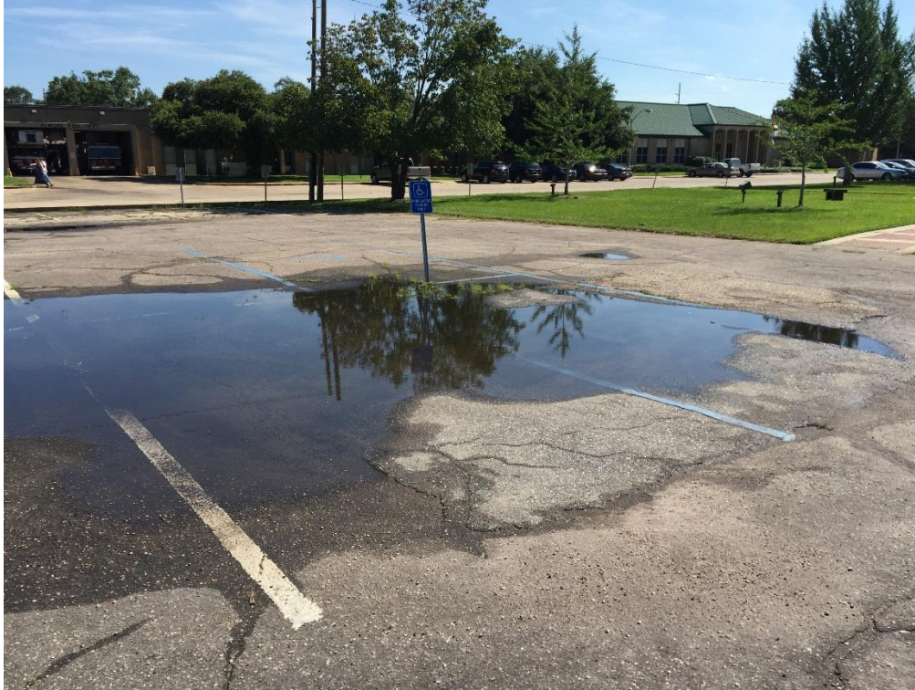
FIG ATR.21 – Current ADA parking space
