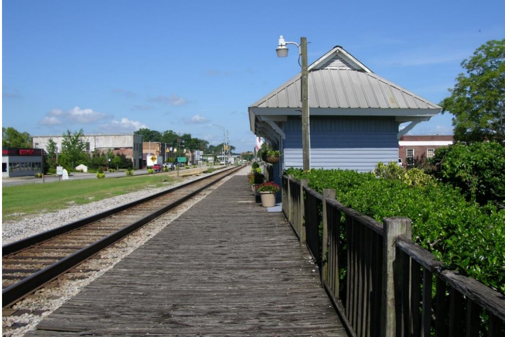
FIG ATR.07 – Existing platform
