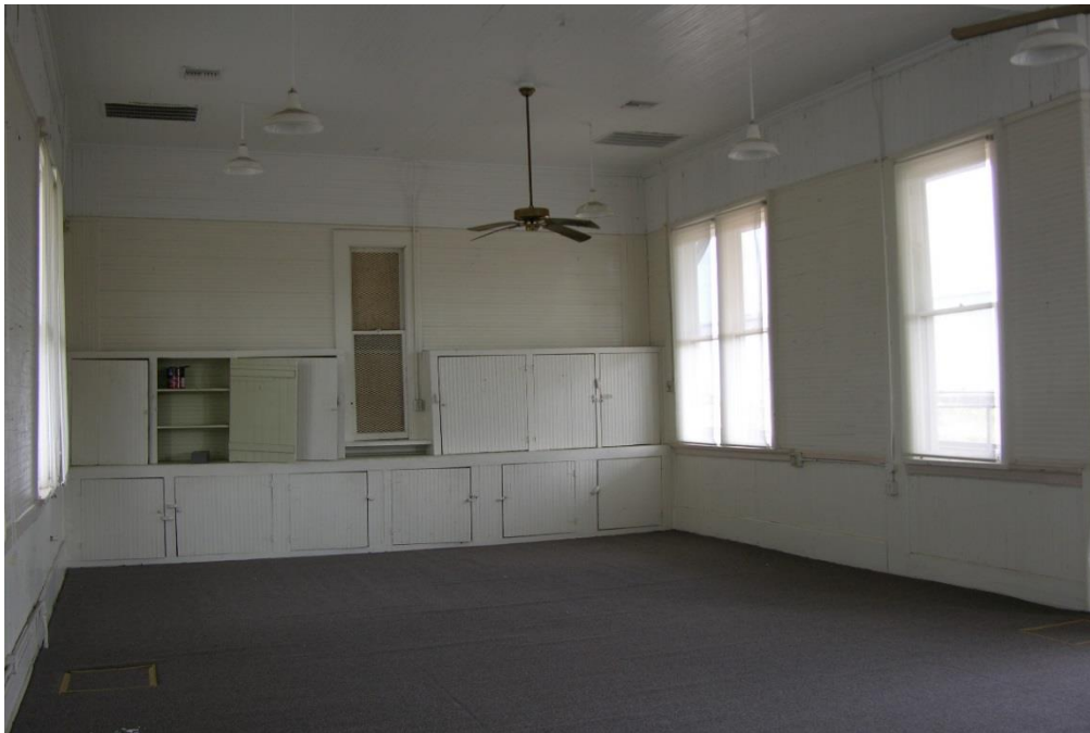
FIG PAG.12 – View from inside ticket office looking west
