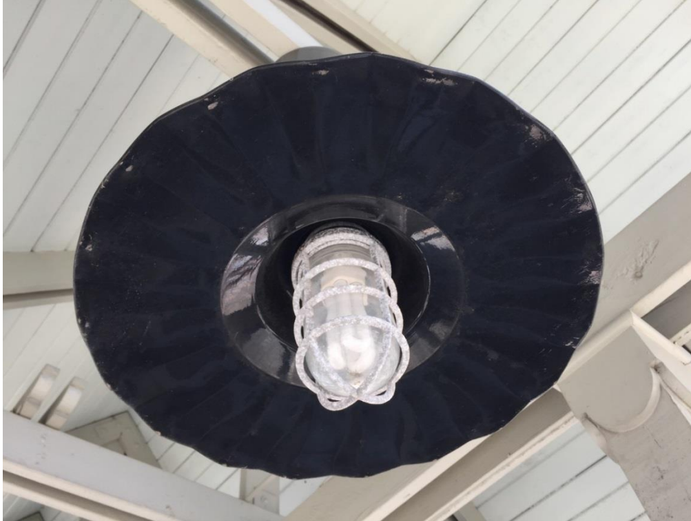
FIG BAS.07 – Lighting at platform shelter in good condition
