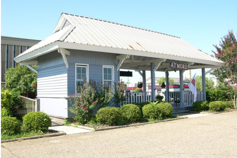
FIG ATR.01 – Station Building with shelter canopy
