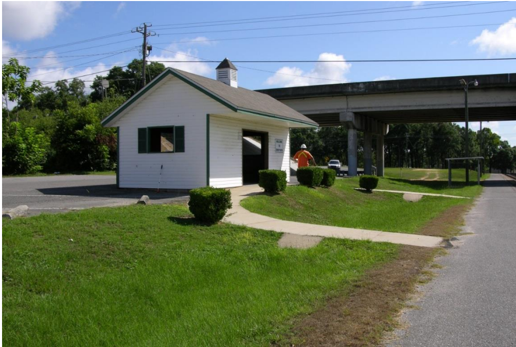
FIG CSV.08 – View of shelter building from platform looking north
