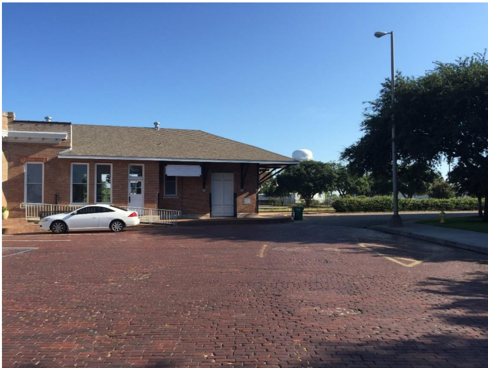
FIG GUF.14 – Parking lot / street light seen to the right
