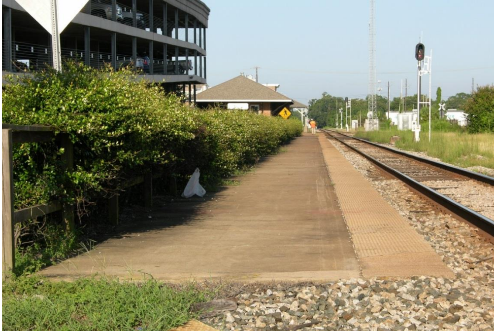
FIG GUF.05 – Platform looking west
