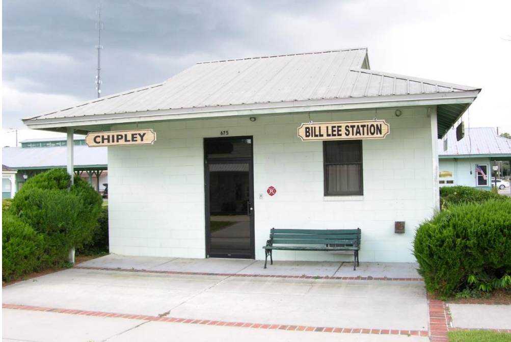
FIG CIP.09 – The station building at the Chipley FL station looking south
