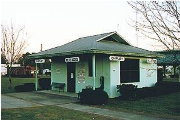
Photo of Station Shelter (Looking Southeast)
