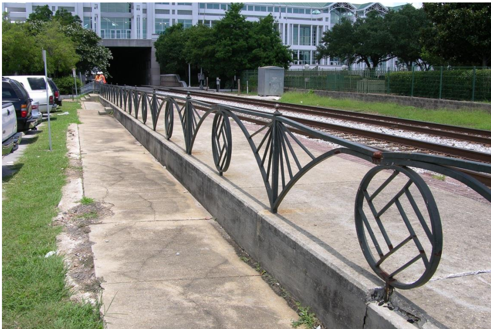
FIG MOE.04 – View of sidewalk along northern end of platform (note the bent railing to the right)
