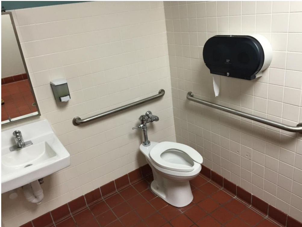
FIG TLH.48 – “ADA” stall in Women’s restroom
