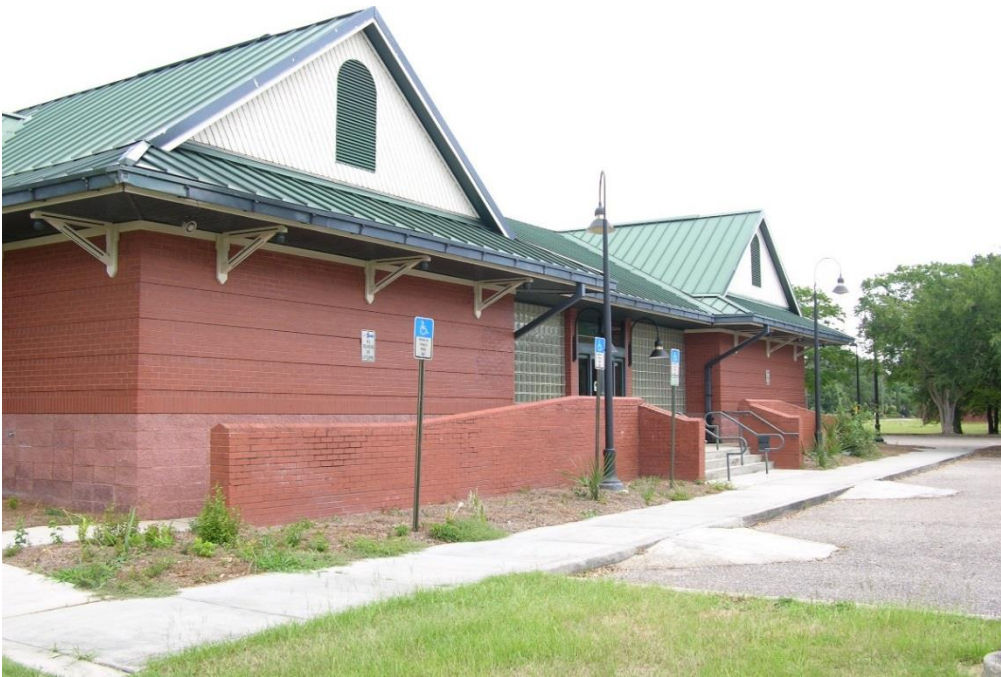
FIG PNS.49 – Candy-cane lamp in front of station that needs to be adjusted
