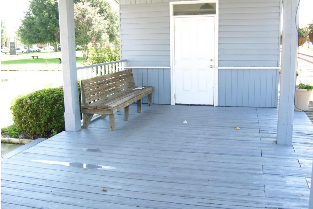
FIG ATR.13 – Covered Shelter area with door and bench
