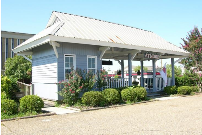
Photo of Station Shelter Looking Southwest
