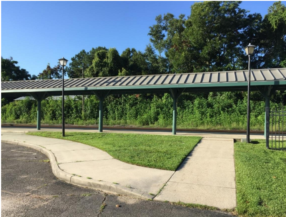
FIG TLH.12 – Different perspective of sidewalk / ramp seen in FIG TLH.09; metal standing roof of canopy; no tactile at beginning of ramp
