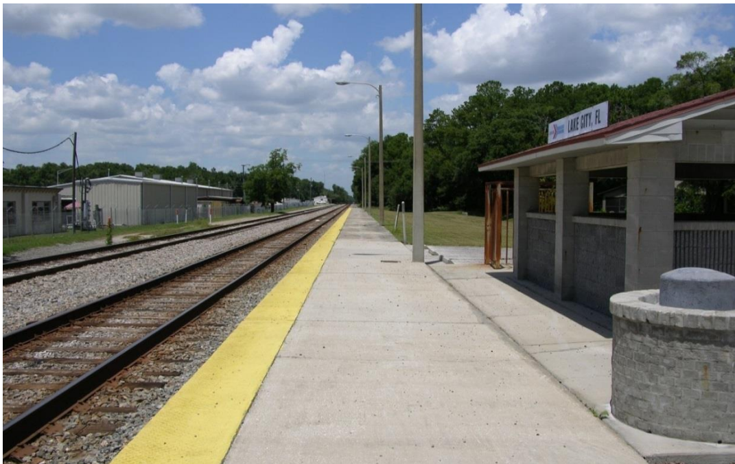
FIG LAC.04 – The platforms walking surface has minor cracks that need to be patched. Also, non-compliant site ID signage visible on shelter. Tactile surface is worn and needs replacing due to “nubs” being worn down.
