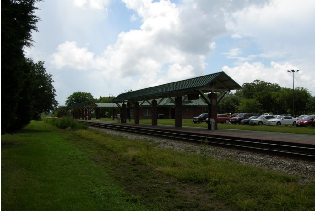
FIG PNS.15 – View from across tracks of all three platform canopies
