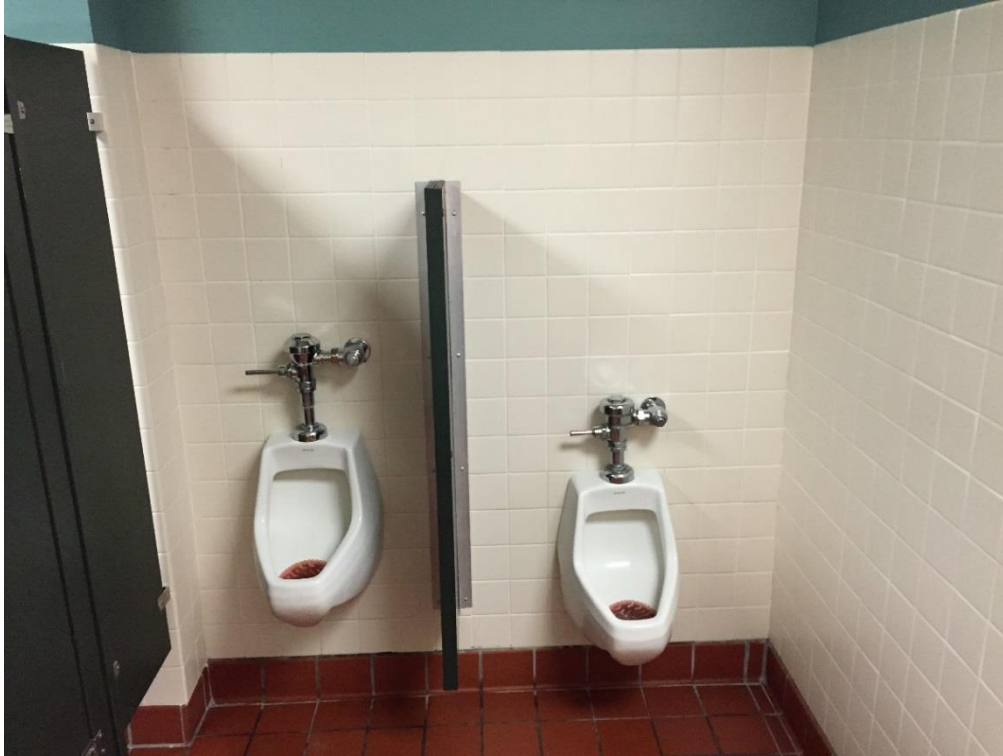
FIG TLH.43 – Urinals in Men’s restroom
