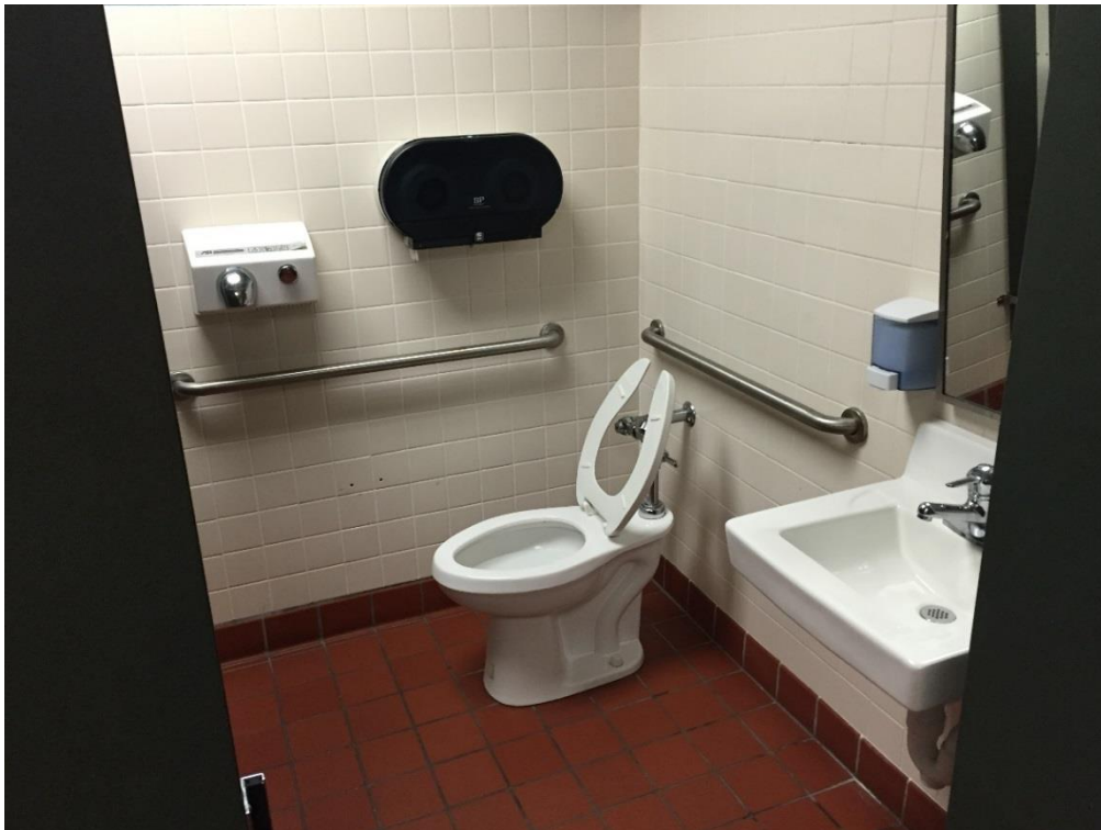
FIG TLH.44 – Toilet stall in Men’s restroom
