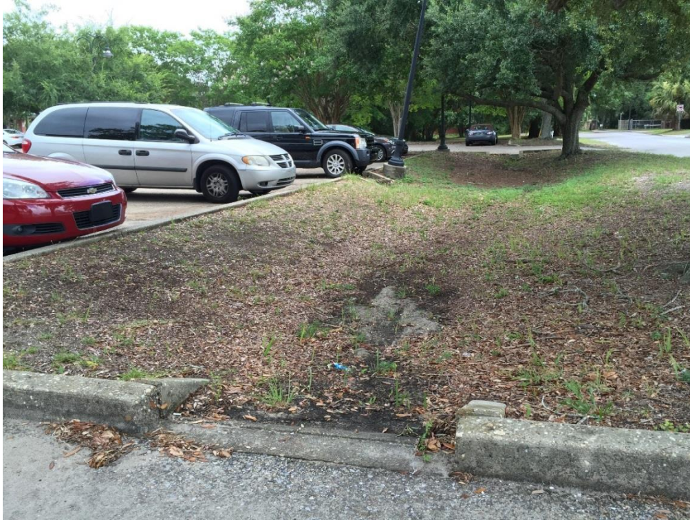
FIG PNS.09 – Swale located between entrance driveways
