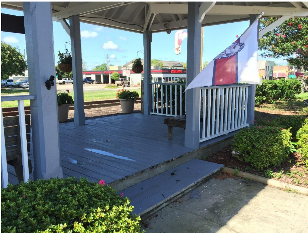
FIG ATR.14 – Platform / Canopy entrance
