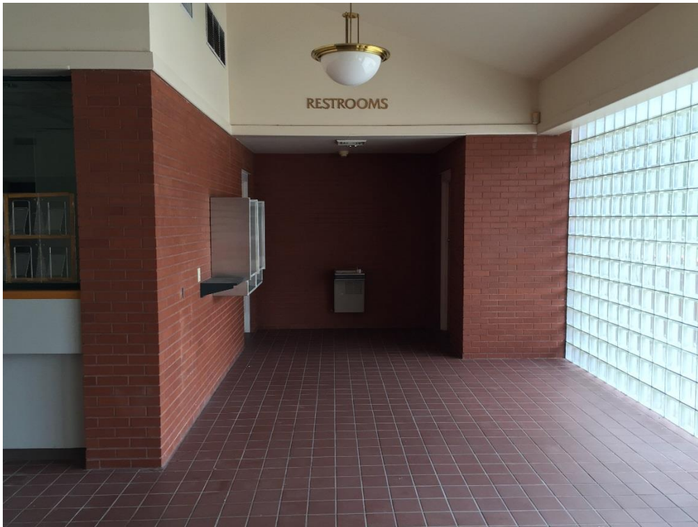
FIG PNS.22 – Interior of waiting room looking towards restrooms
