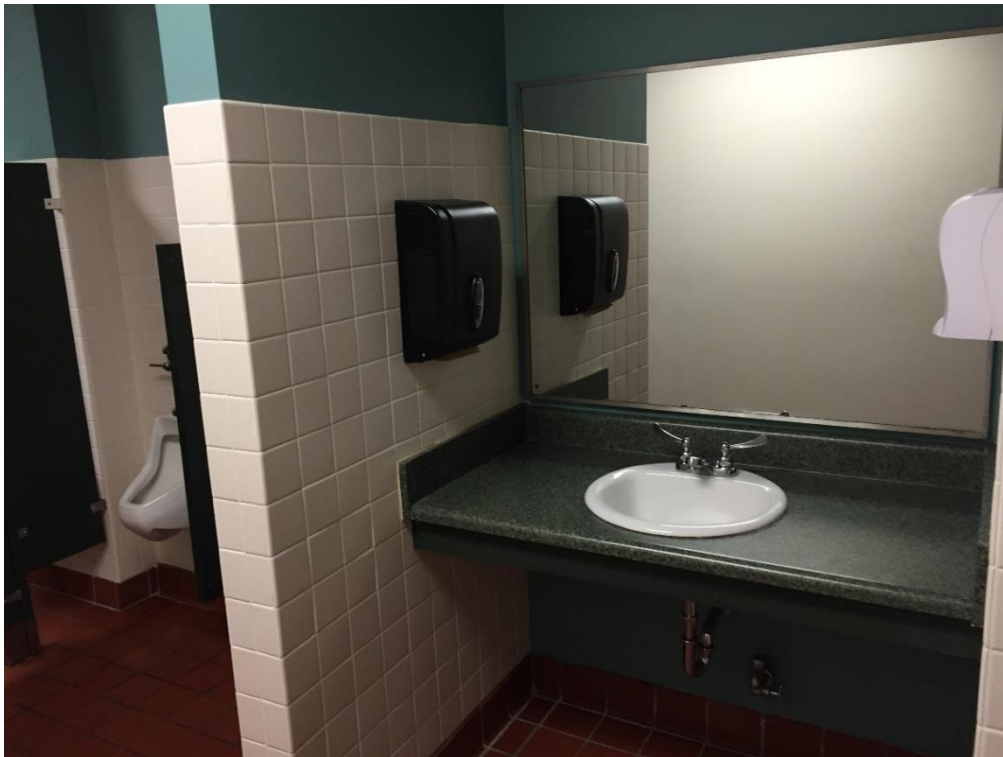
FIG TLH.42 – Sink in Men's restroom
