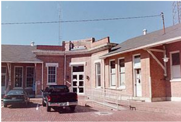
Photo of Station Building (Looking Northwest)
