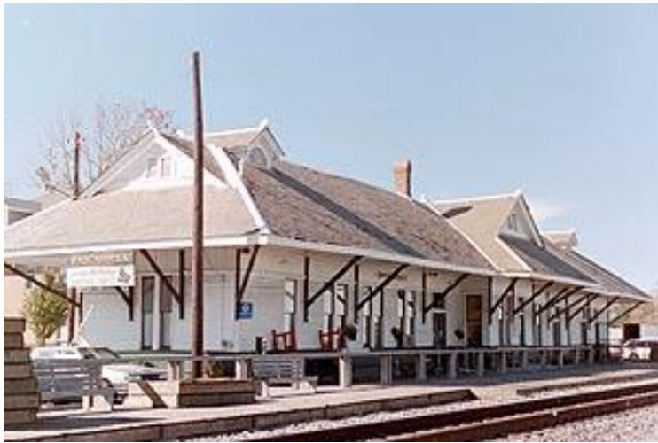
Photo of Station Building (Looking Southwest)
