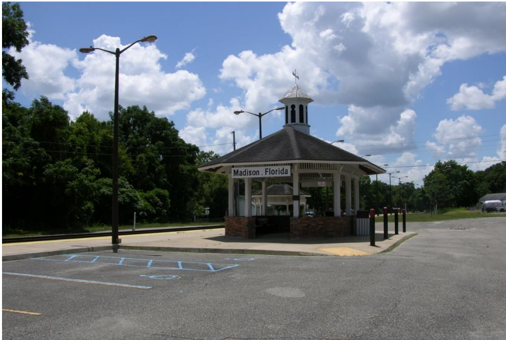
FIG MDO.20 – Structure with site lighting on left
