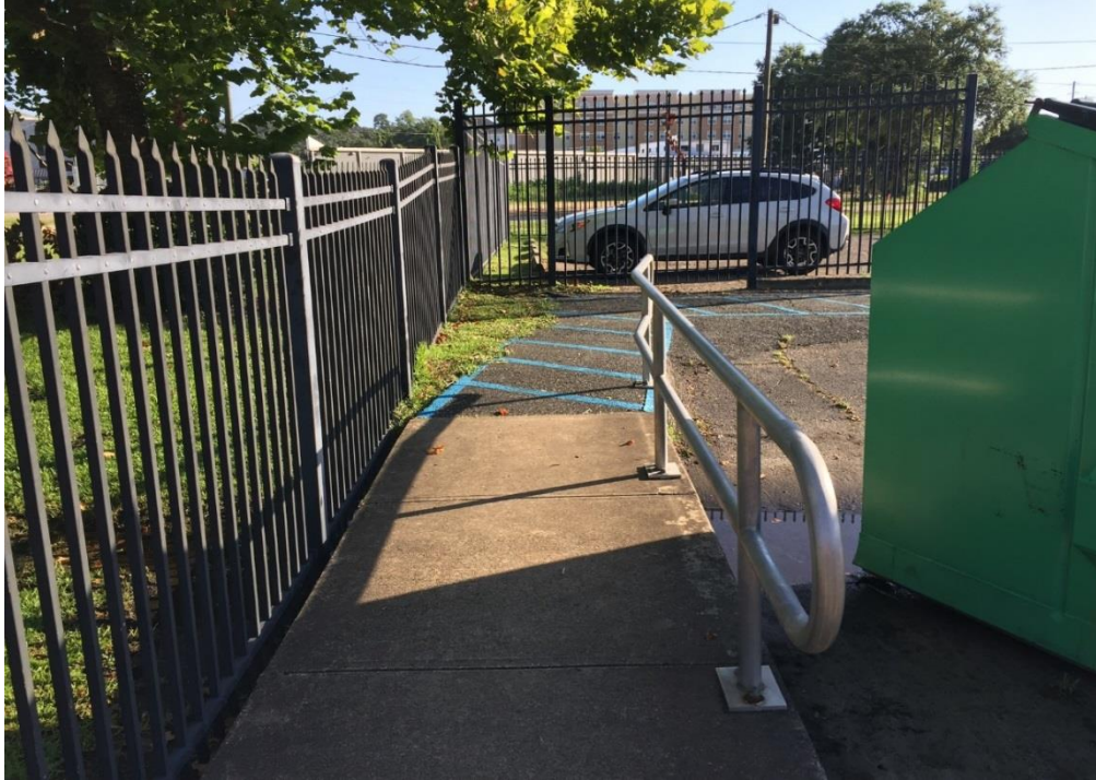
FIG TLH. 59 – Ramp leading from Amtrak ADA parking space to building across the driveway from station (See FIG TLH.14 for connection to ADA parking space)
