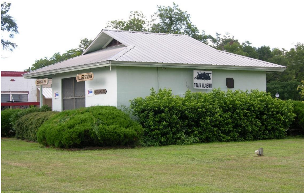
FIG CIP.08 – The station building at the Chipley FL station looking northeast
