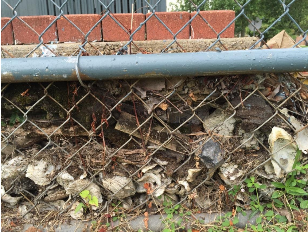
FIG PAG.05 – Cross-sectional view of brick apron
