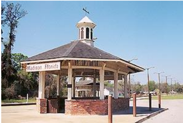
Photo of Station Shelter (Looking Southwest)
