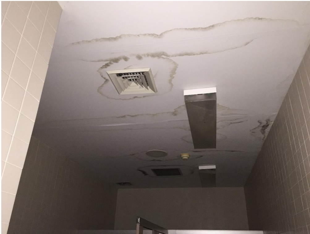
FIG PNS.36 – Women’s restroom ceiling
