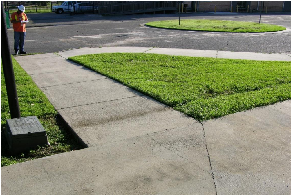
FIG TLH.20 – Minor cracking at end of ramp connecting parking area to platform
