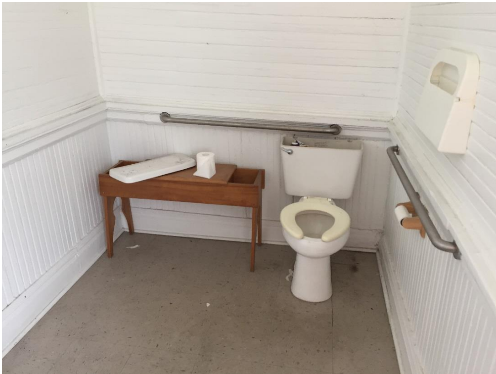
FIG PAG.14 – Toilet in Men’s restroom
