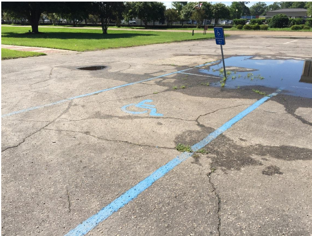
FIG ATR.20 – Current ADA parking space
