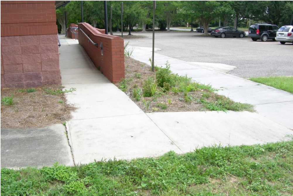
FIG PNS.06 – Sidewalk on western side of station building
