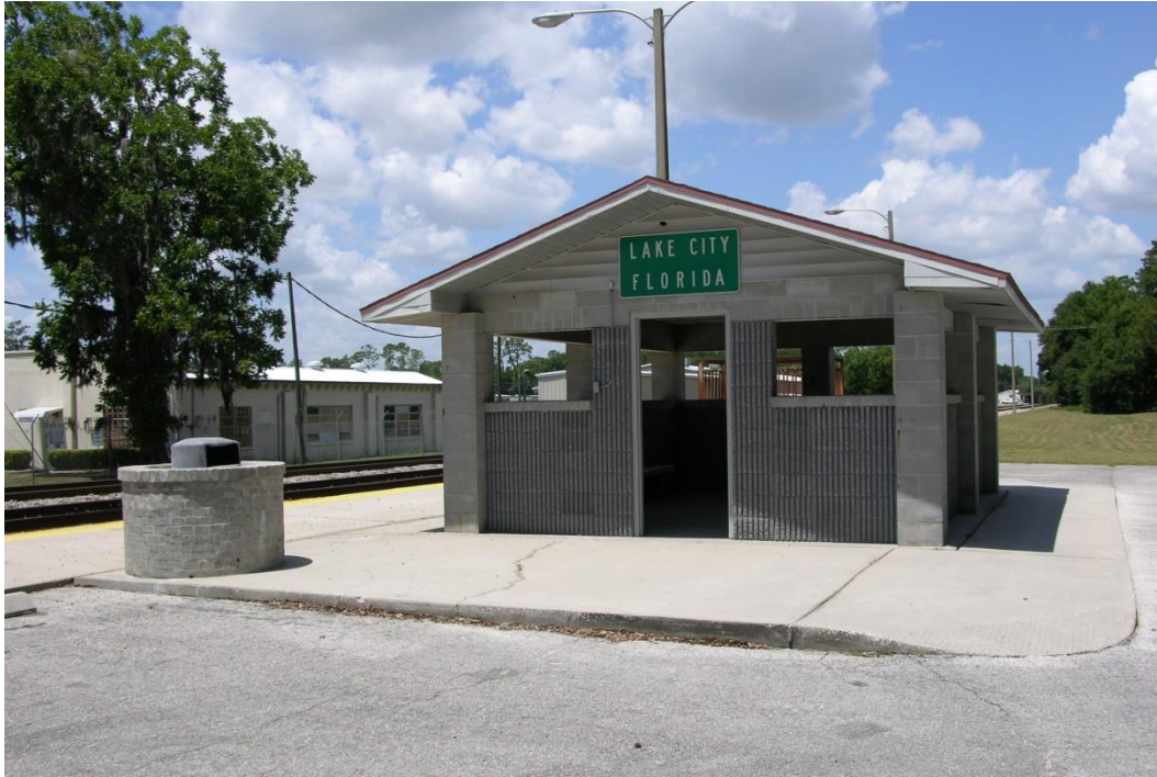
FIG LAC.01 – sidewalks and curbs with shelter; curb ramps not complaint
