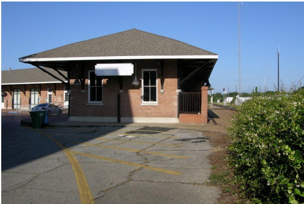
FIG GUF.04 – Asphalt adjacent to platform
