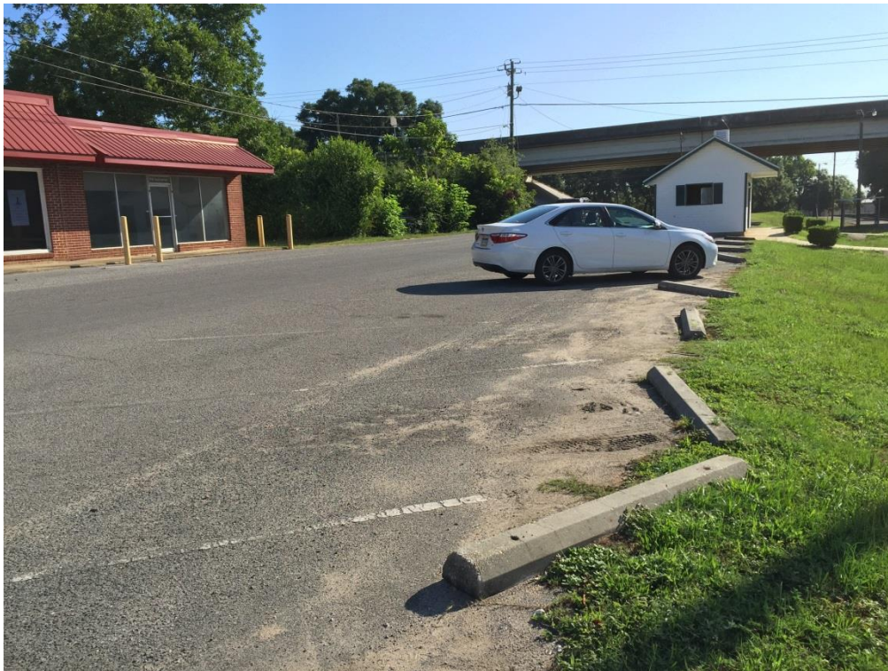
FIG CSV.02 – Parking Lot looking east with shelter in background
