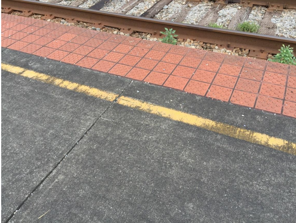
FIG PNS.56 – Tactile edge on platform
