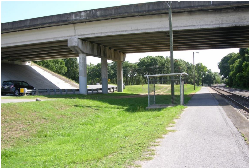
FIG CSV.10 – Platform view showing wheel chair lift shelter and grass encroaching on platform
