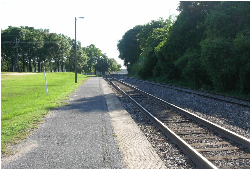
FIG CSV.03 – Platform looking northeast
