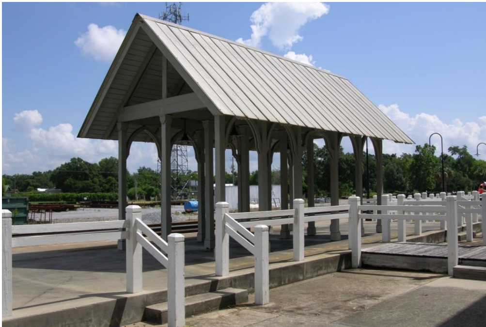
FIG BAS.04 – Platform Canopy structure
