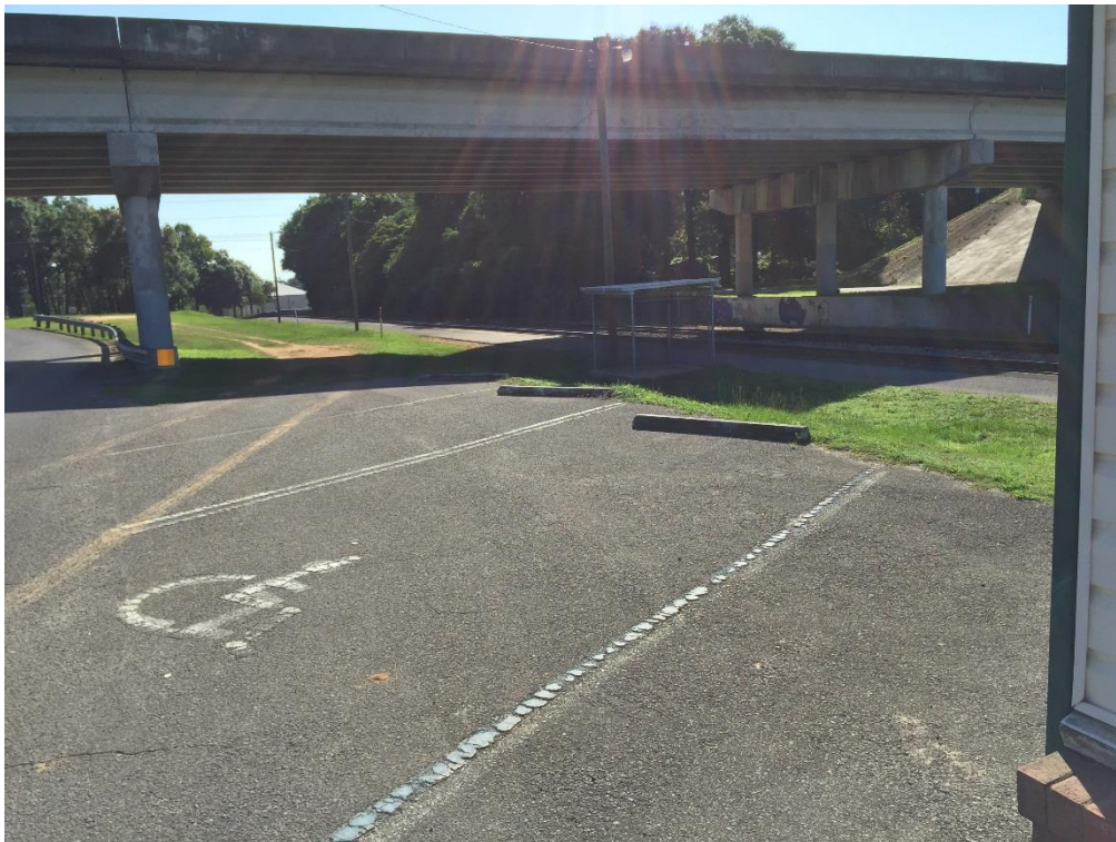
FIG CSV.16 – Additional parking to northeast of station building
