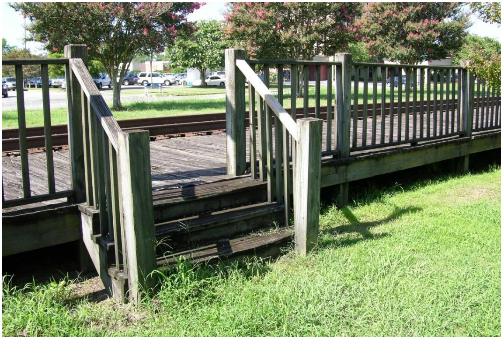
FIG ATR.04 – Stairs leading to platform
