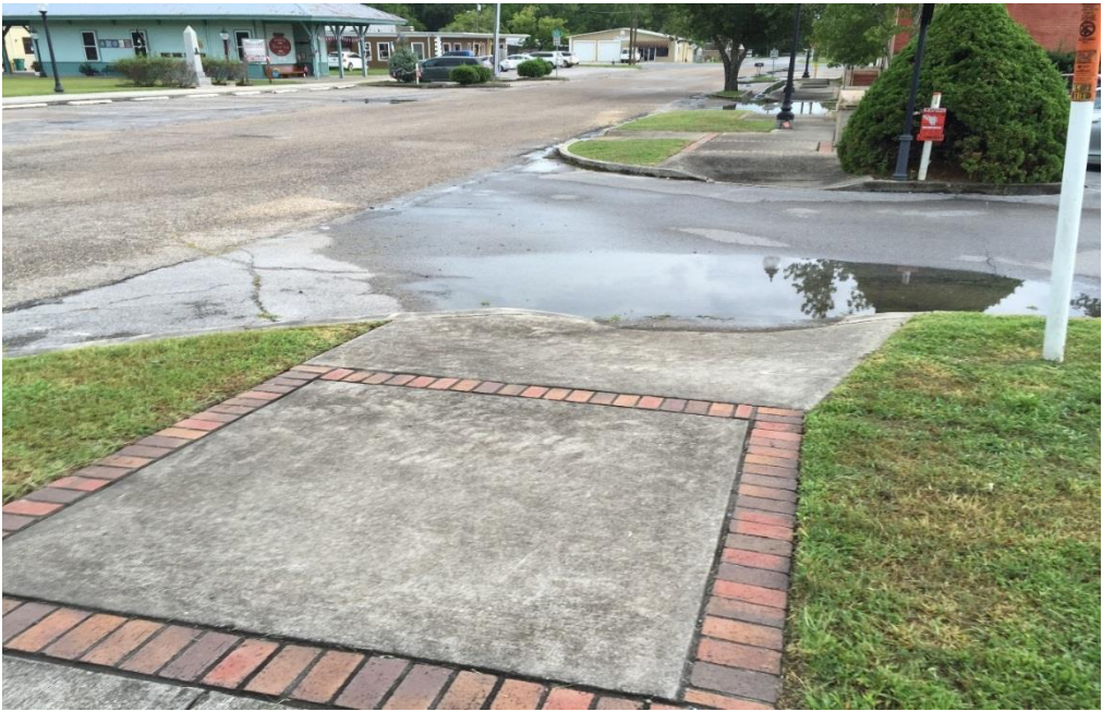
FIG CIP.04 – The sidewalk and curbs for Chipley FL station
