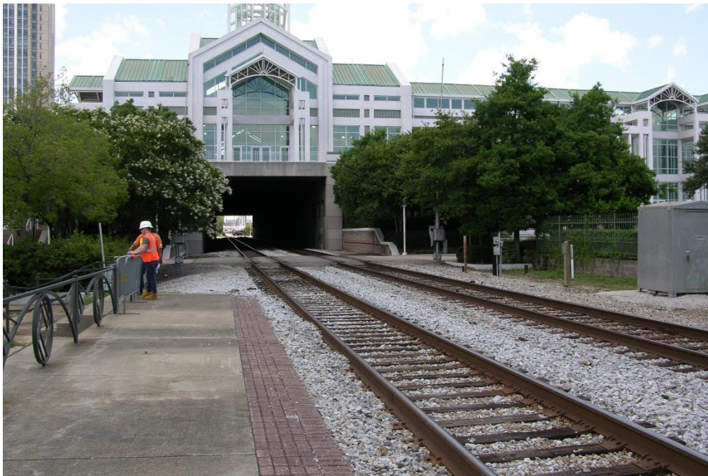
FIG MOE.16 – View of the tunnel beneath the convention center located north of the platform
