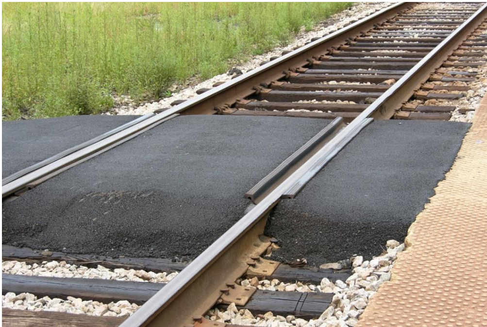
FIG GUF.16 – Close-up view of pedestrian grade crossing with ramp leading to crosswalk seen in FIG GUF.15 located to the right (out-of-view in this picture)
