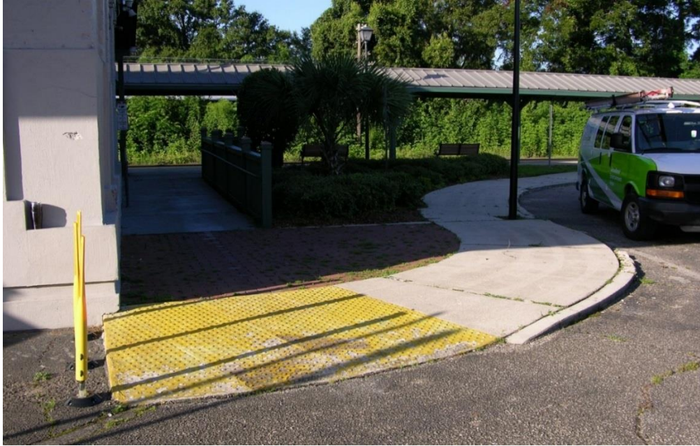
FIG TLH.11 – Curbs, ramps, and sidewalks at end of roundabout / leading to steps into station waiting room
