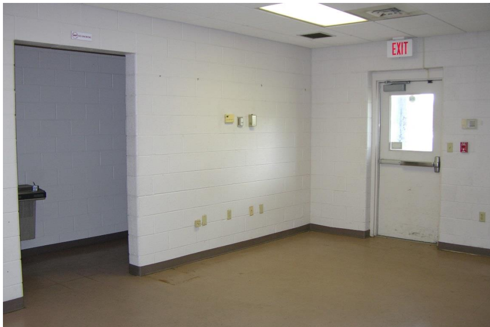
FIG PNS.32 – Office space lobby (restrooms—unable to be surveyed due to odor—located to the left; two (2) offices located to the left)
