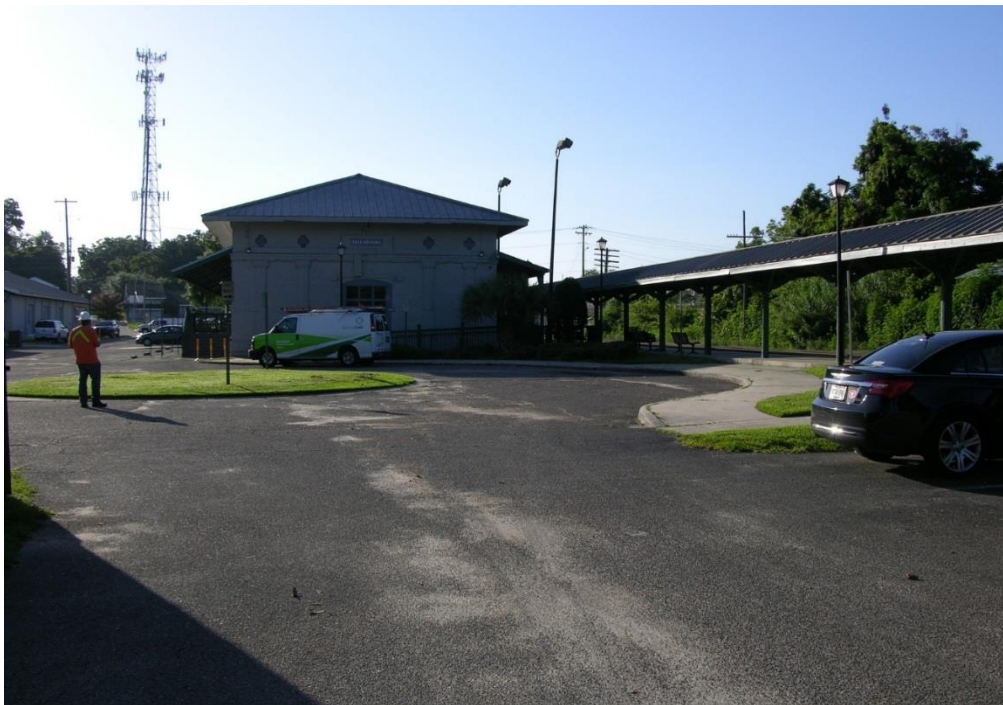
FIG TLH.04 – Potholes and standing water evidence in Parking Lot for Tallahassee FL station
