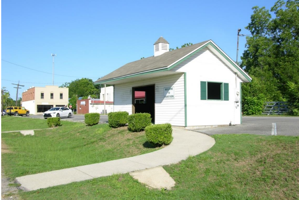
FIG CSV.01 – View from NW of station open air shelter with sloped semicircular ramp from platform
