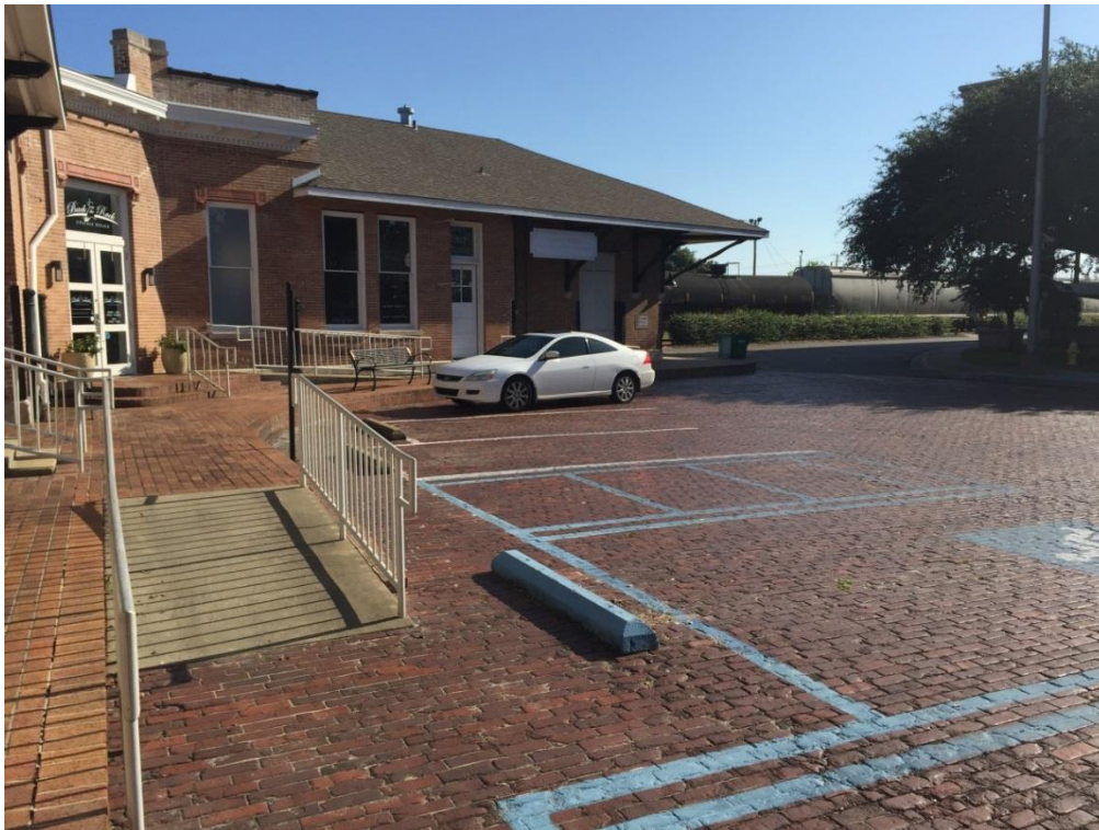
FIG GUF.02 – View of station building and ADA parking
