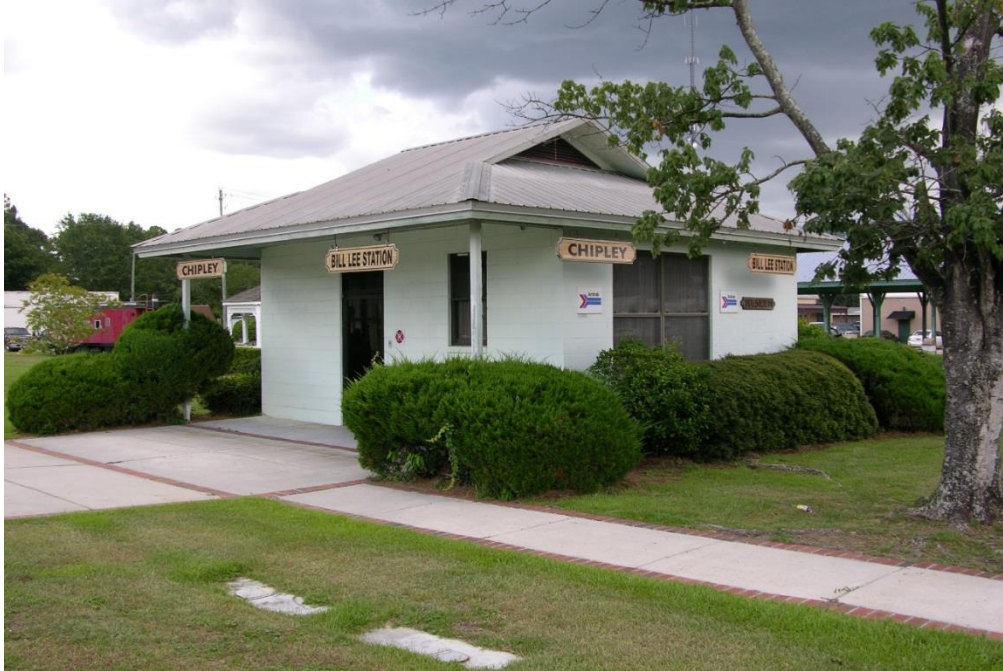
FIG CIP.07 – The station building at the Chipley FL station looking southwest
