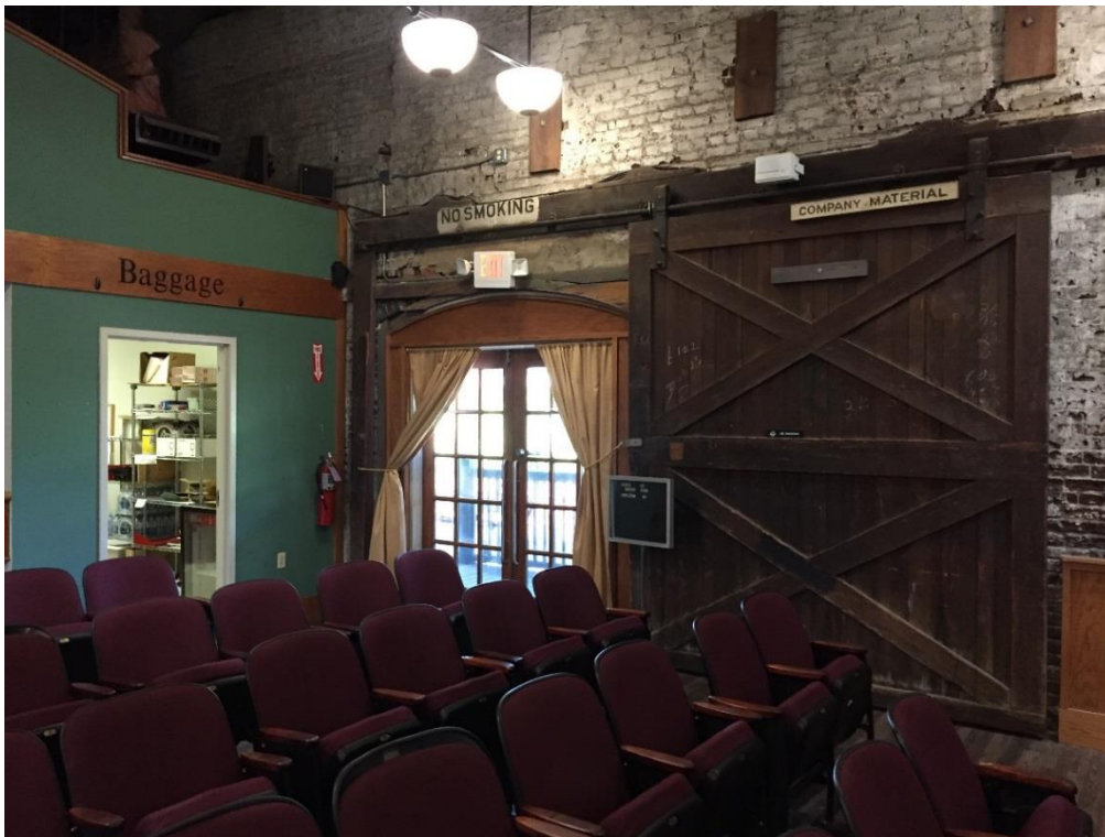
FIG TLH.38 – Convenience outlet can be see in the back lefthand corner, next to the fire extinguisher
