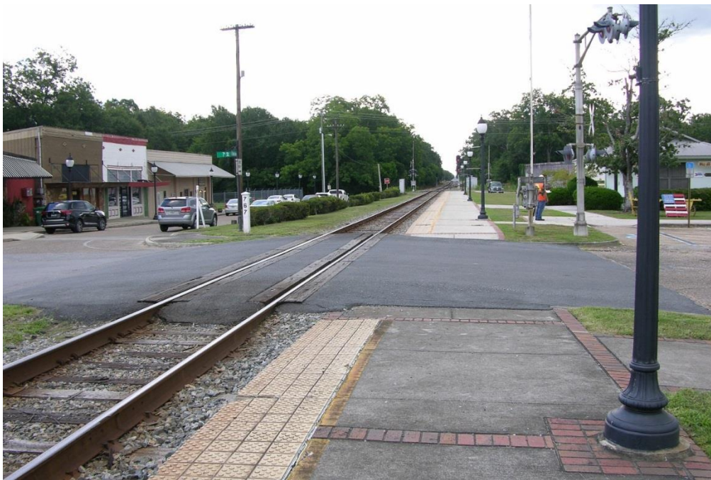
FIG CIP.02 – Rail crossing at Martin Luther King Drive (east of station building)
