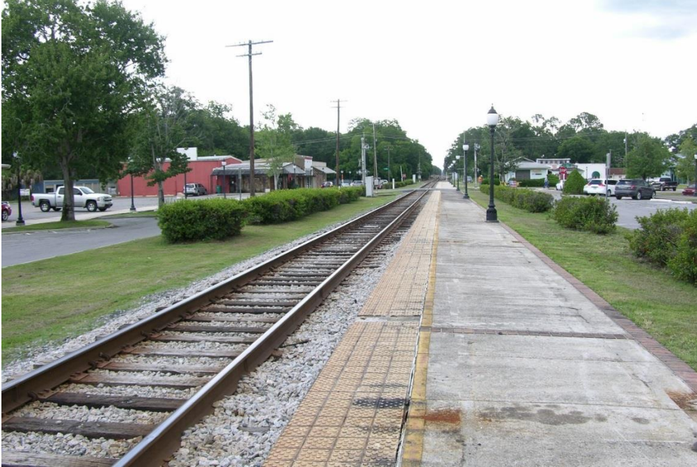
FIG CIP.13 – View from end of western platform
