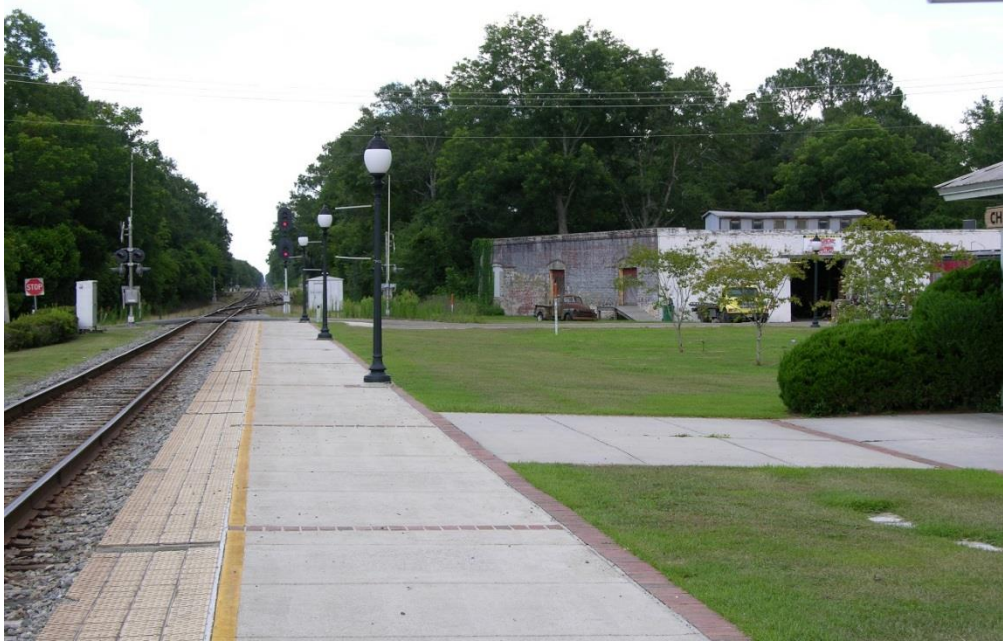
FIG CIP.11 – The poured in place concrete platform for the Chipley FL station
