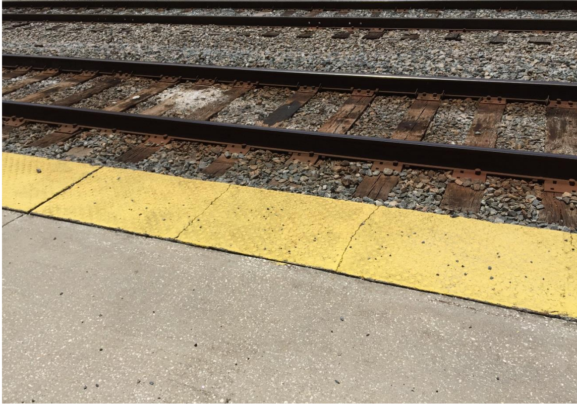
FIG LAC.07 – The “nubs” on the system for Lake City FL station have been worn and system is cracking
