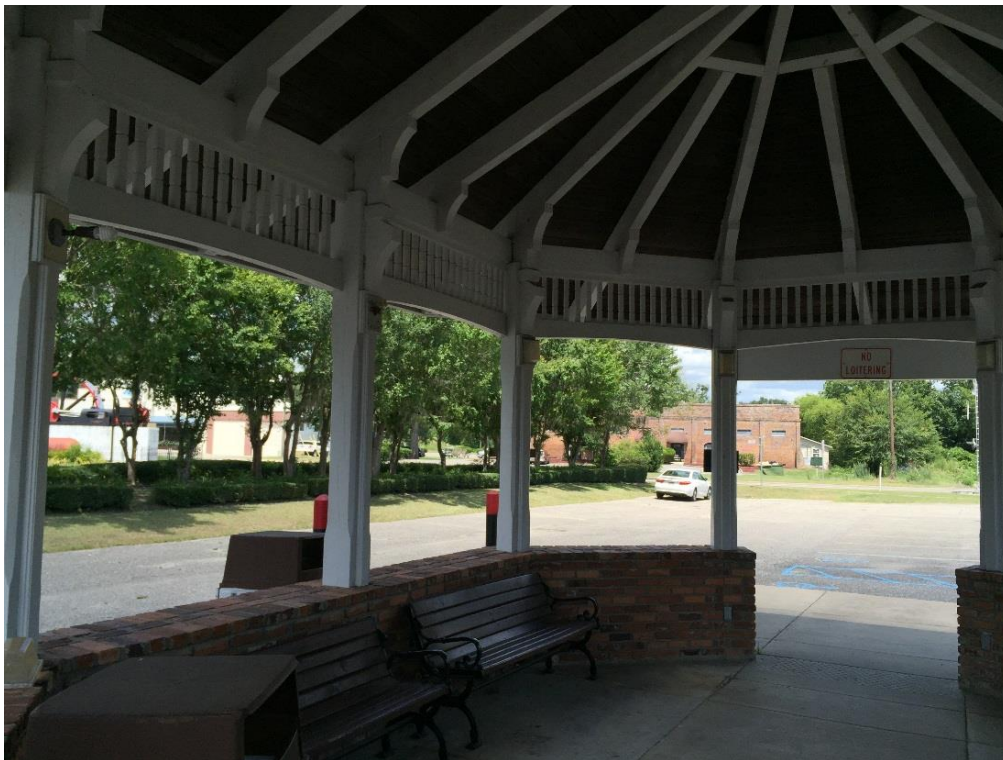
FIG MDO.21 – Wall packs can be see attached to each column
