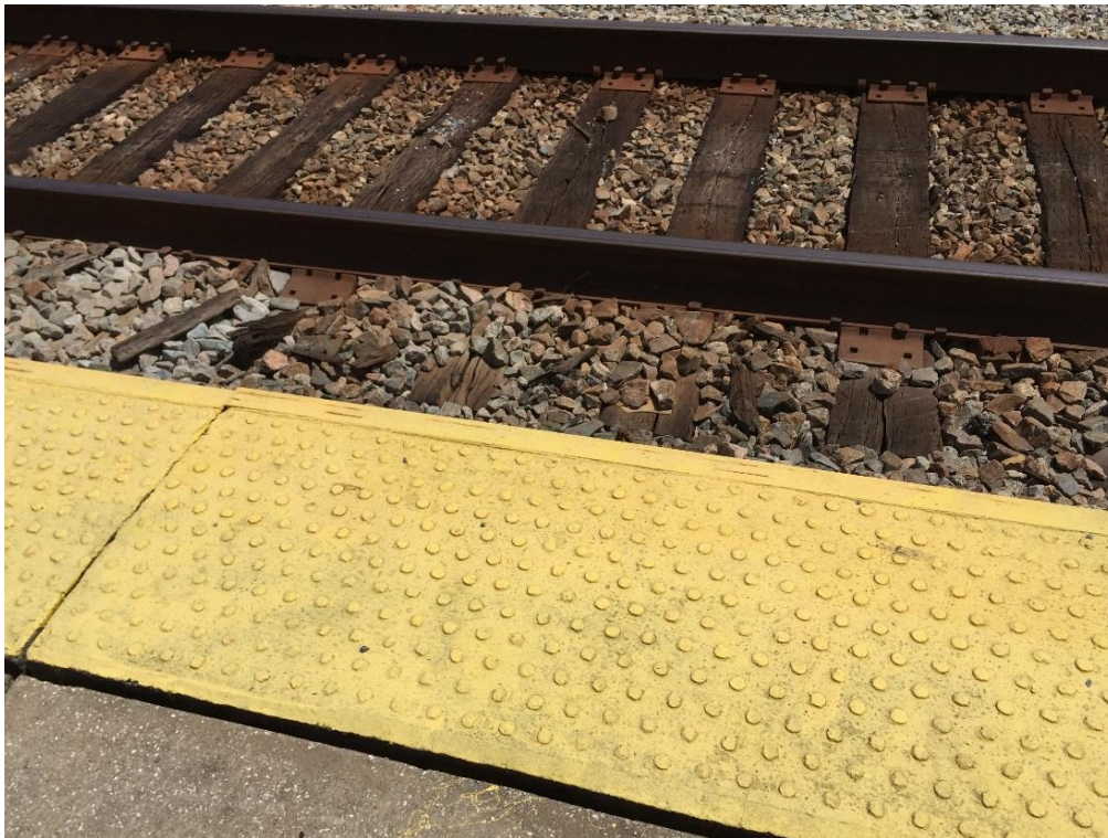
FIG MDO.14 – Typical tactile strip at this station—seems to have been painted a few months prior to site survey.
