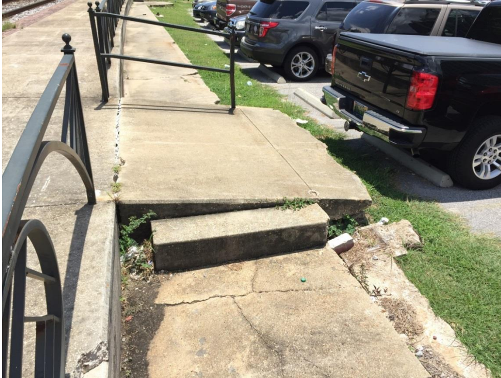
FIG MOE.03 – Partially demolished ramped at northern end of platform
