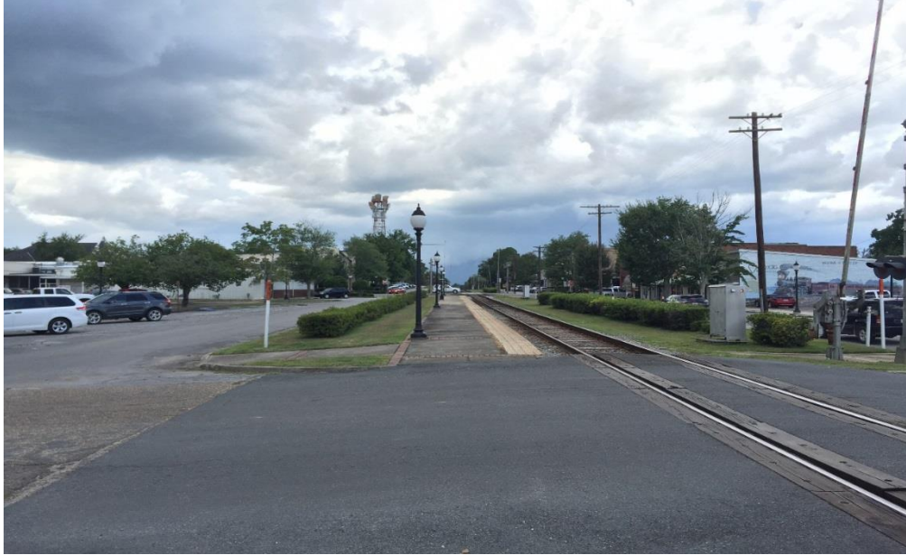
FIG CIP.01 – Rail crossing at 7 th street (west of station building)
