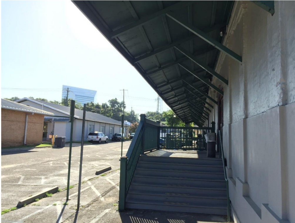
FIG TLH.13 – Stairway leading to waiting room
