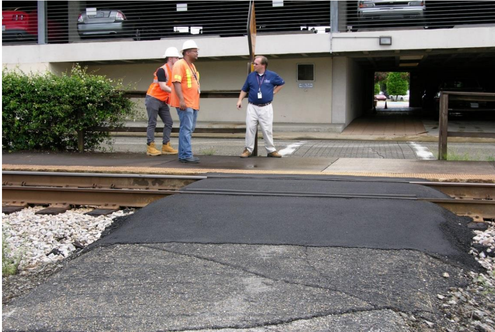
FIG GUF.15 – Pedestrian grade cross with ramp (no tactile) leading to cross-walk / parking garage
