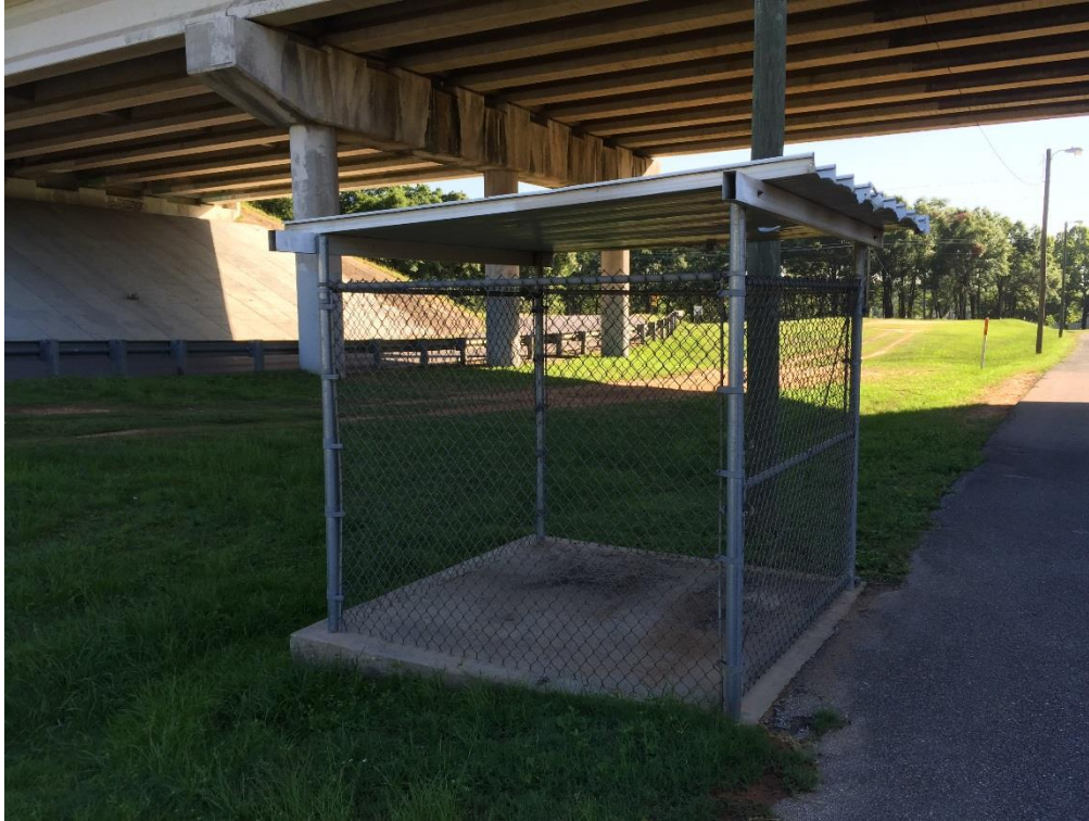
FIG CSV.19 – Close-up view of wheelchair lift enclosure
