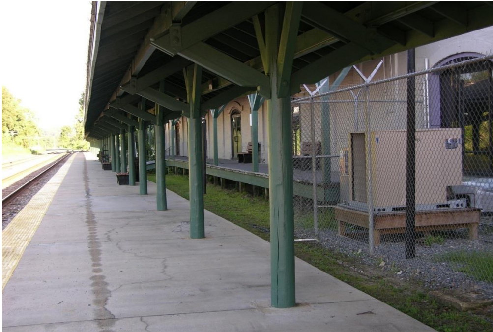
FIG TLH.26 – View of lower portion of platform canopy
