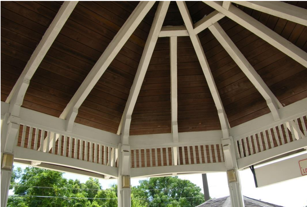
FIG MDO.18 – Roof construction inside shelter
