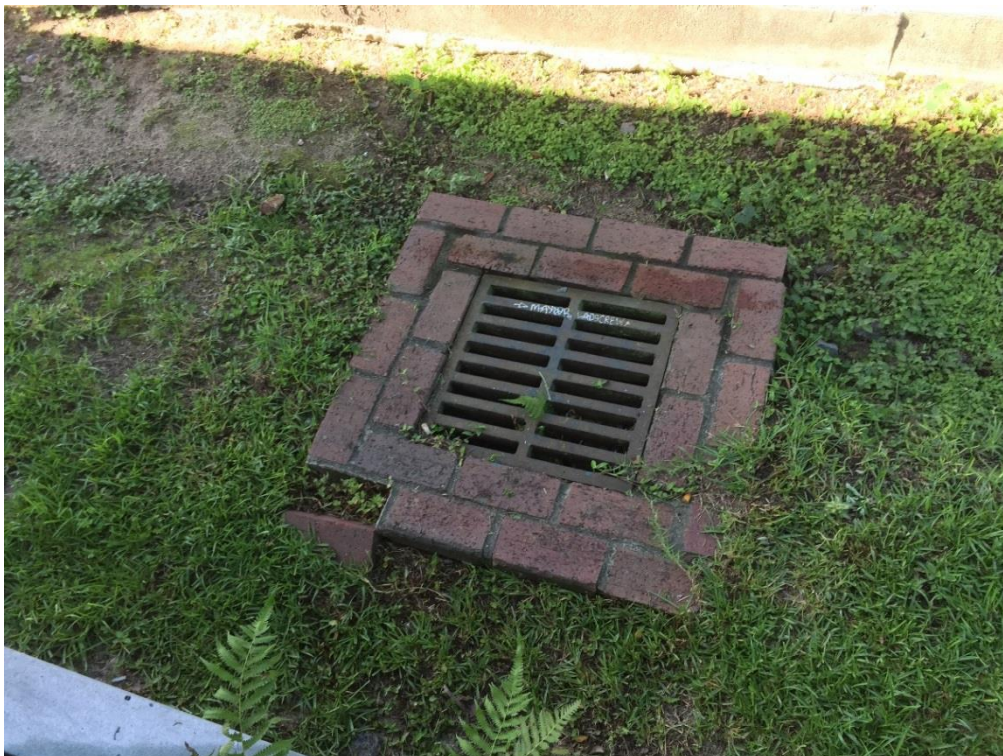
FIG TLH.62 – Site drain located in swale between platform and station building – one brick paver has come loose
