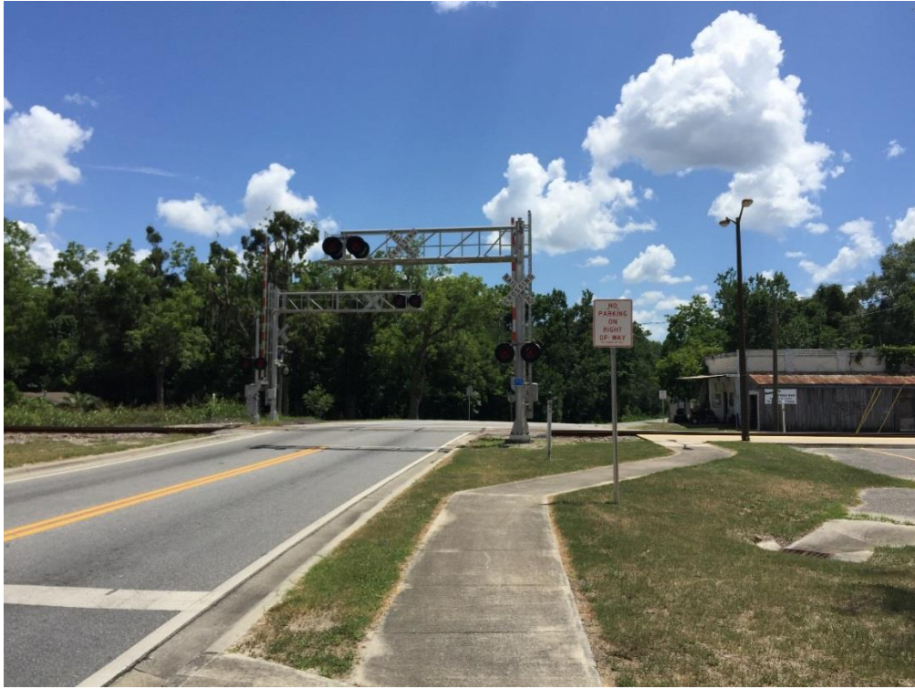
FIG MDO.03 – Sidewalk connecting platform to public right of way (site drain can be seen to the right).
