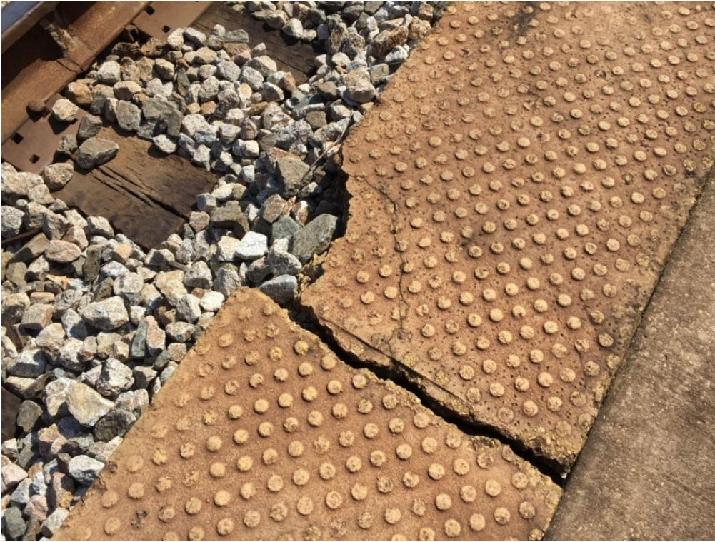
FIG GUF.11 – Tactile Surface
