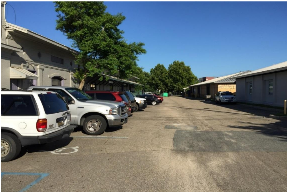
FIG TLH.08 – Potholes and standing water evidence in driveway / parking area leading to parking lot
