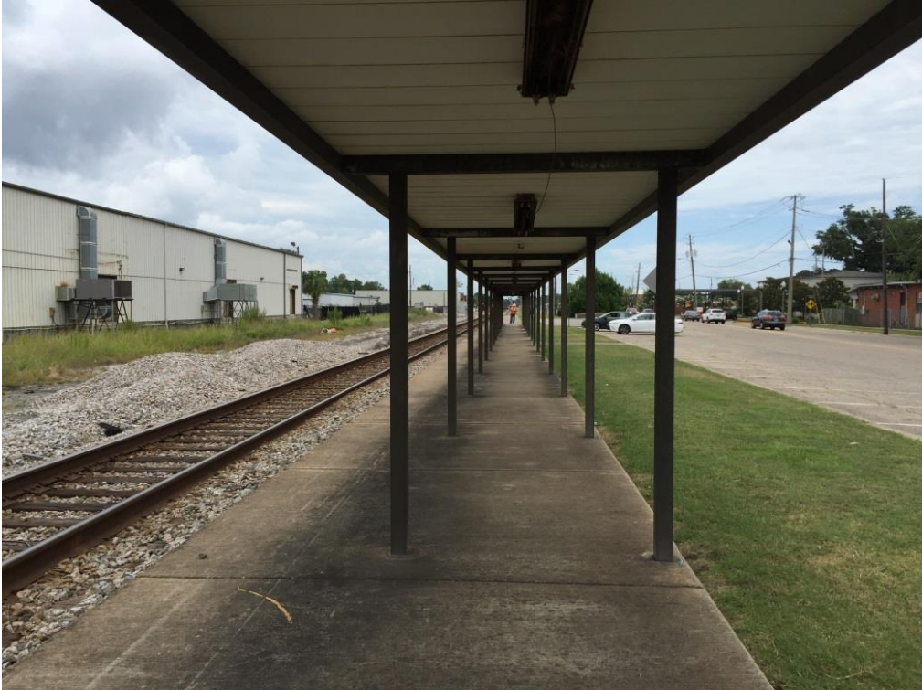
FIG BIX.06 – Platform under canopy looking east
