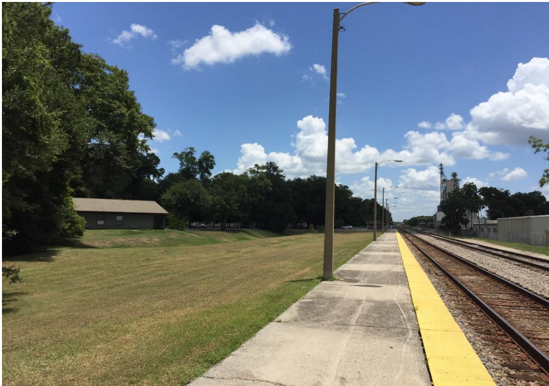
FIG LAC.06 – The platforms walking surface has minor cracks that need to be patched for Lake City FL station
