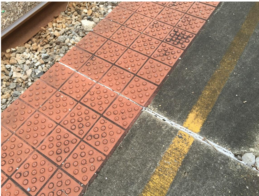
FIG PNS.55 – Tactile edge on platform with expansion joint
