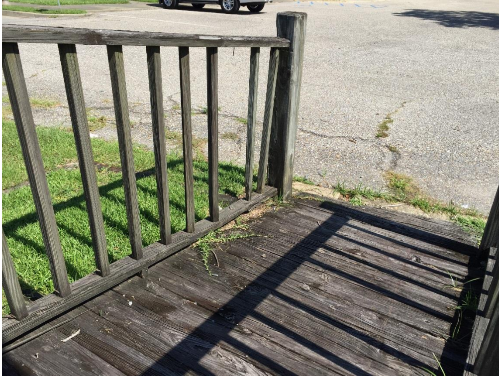
FIG ATR.19 – Street-to-platform access ramp at western-end of platform
