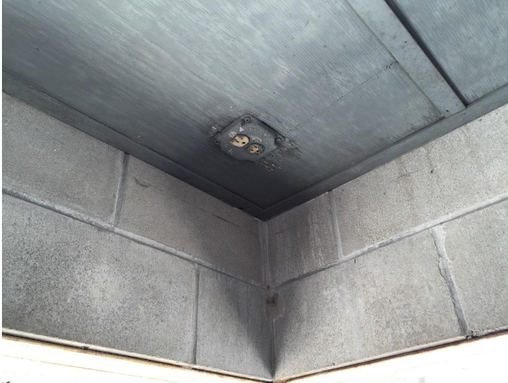
FIG LAC.22 – One of the outlets located on the shelter
