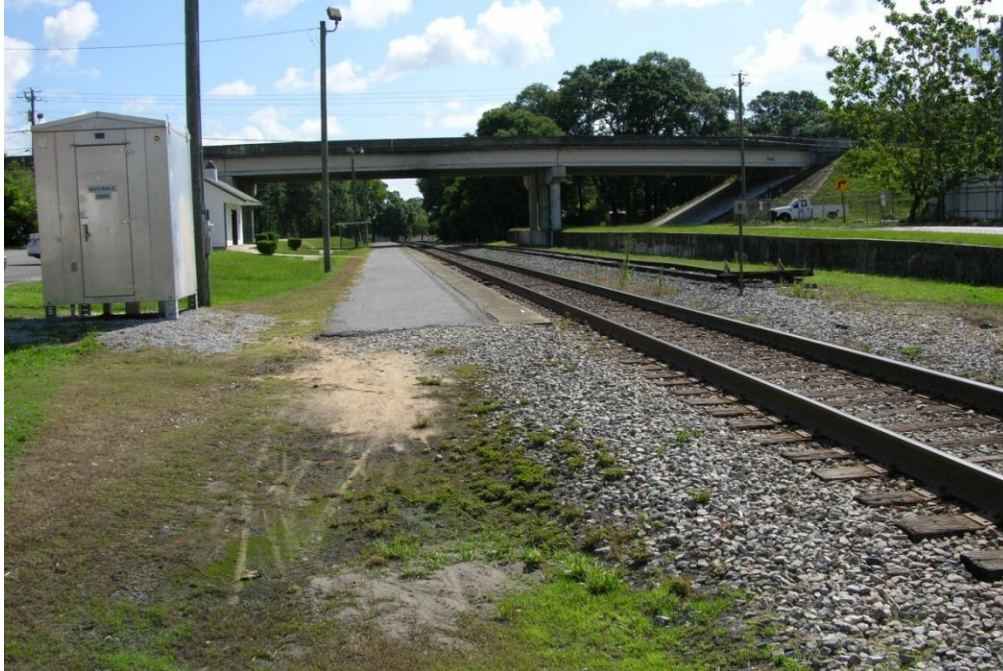
FIG CSV.09 – View of western platform end – looking northeast
