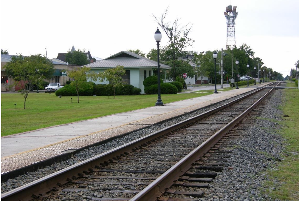
FIG CIP.21 – View of eastern platform from opposite side of the tracks
