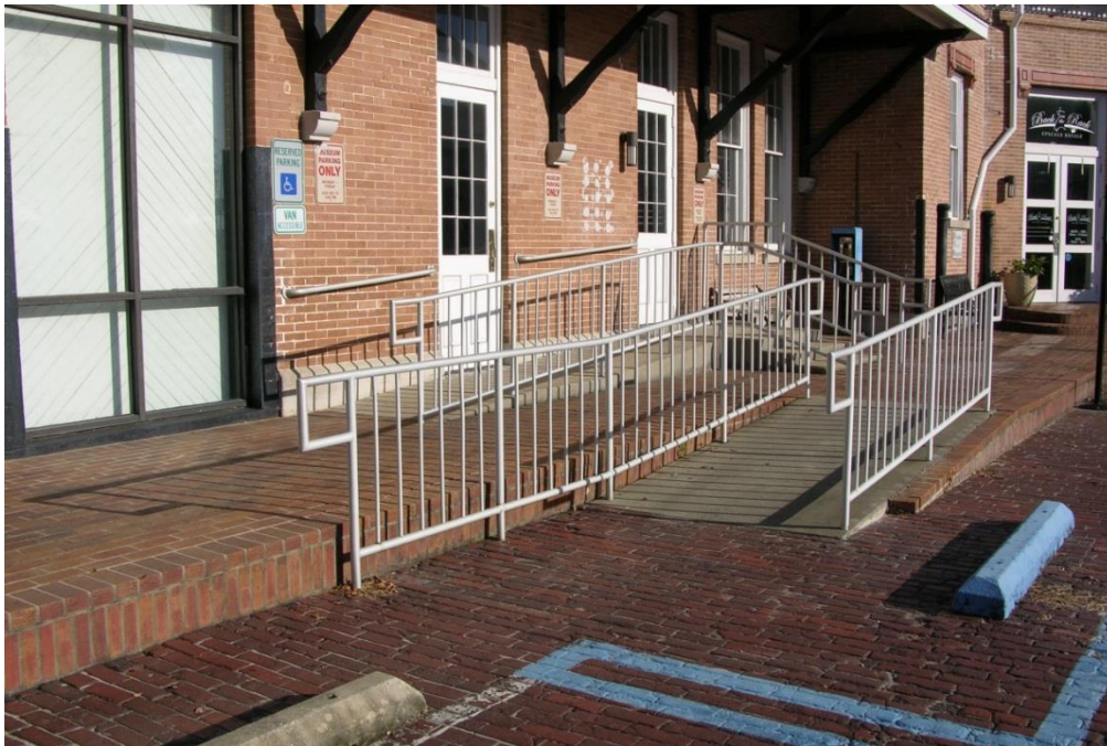
FIG GUF.08 – Access ramp #2
