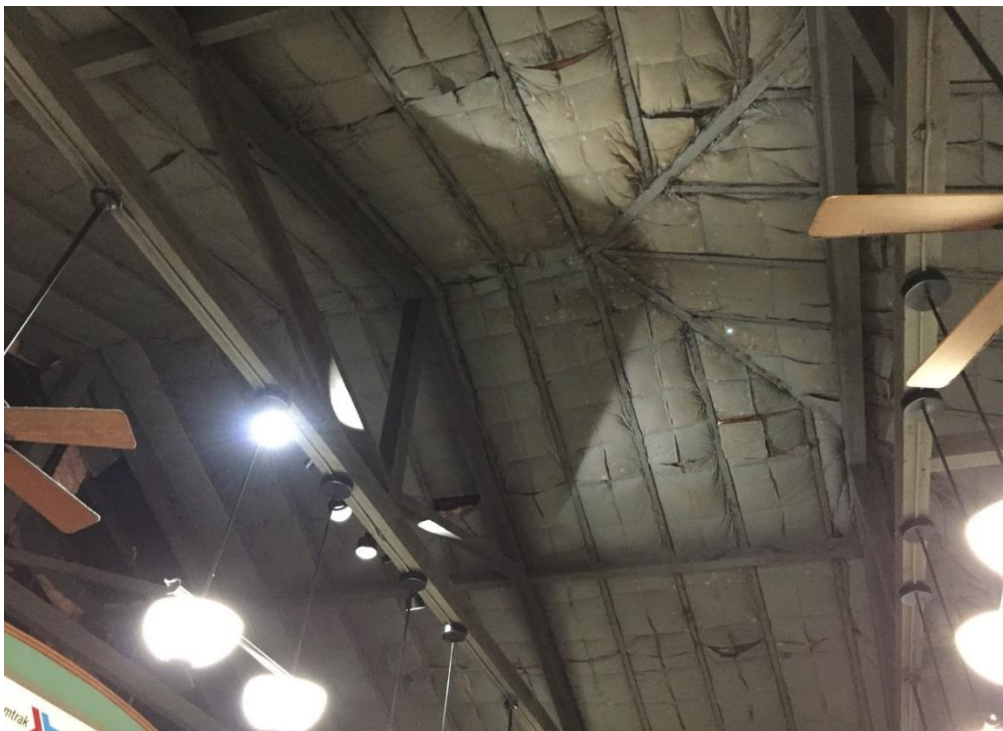
FIG TLH.34 – Exposed wood ceiling rafters and insulation
