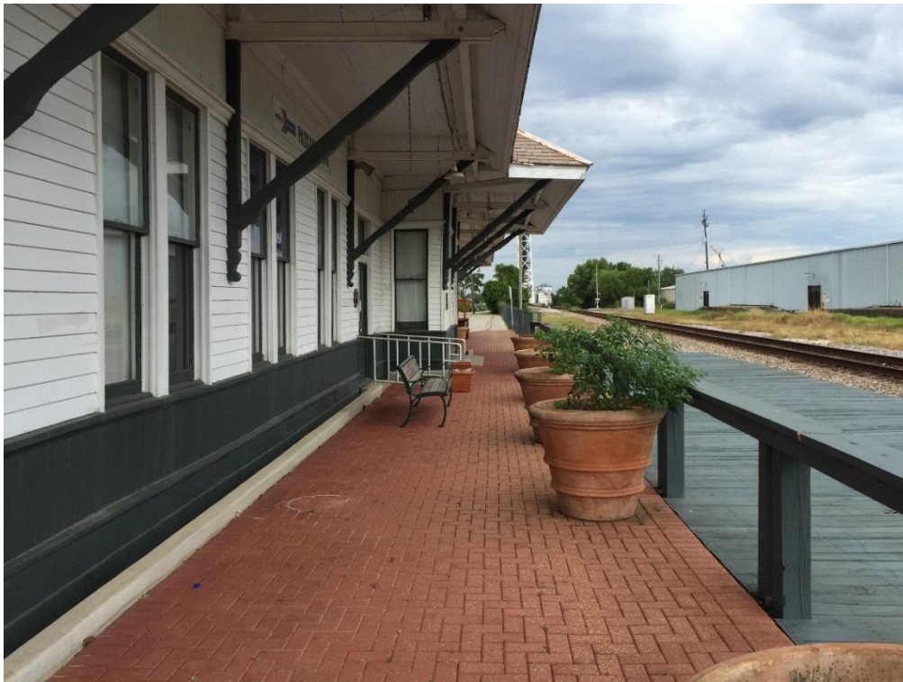
FIG PAG.04 – Brick apron between station building and platform
