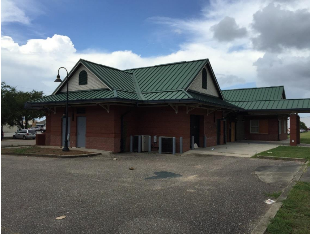
FIG PNS.13 – Baggage cart area (through roll-up door) with access ramp to the right
