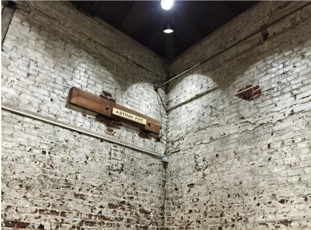
FIG TLH.33 – Exposed brick wall in waiting room
