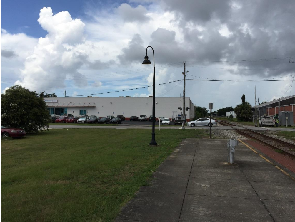
FIG PNS.50 – Candy-cane lamp on platform that needs to be adjusted
