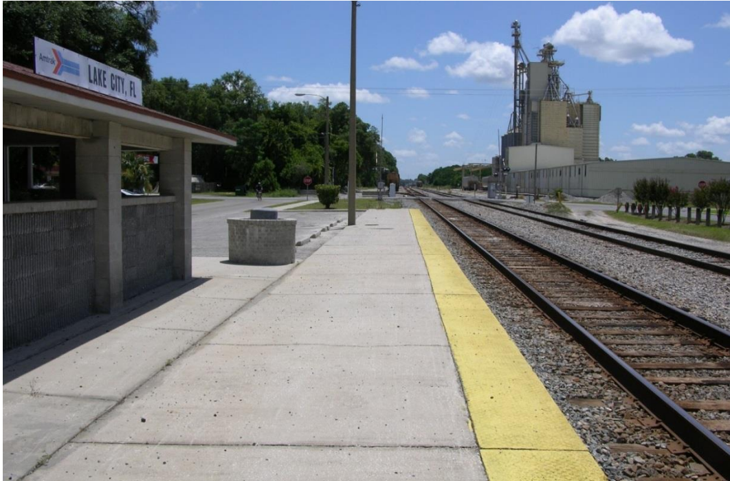
FIG LAC.03 – The platforms walking surface has minor cracks that need to be patched. Also, non-compliant site ID signage visible on shelter. The tactile surface is worn and needs replacing due to “nubs” being worn down.
