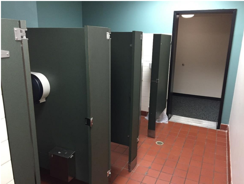
FIG TLH.46 – Stalls in Women’s restroom
