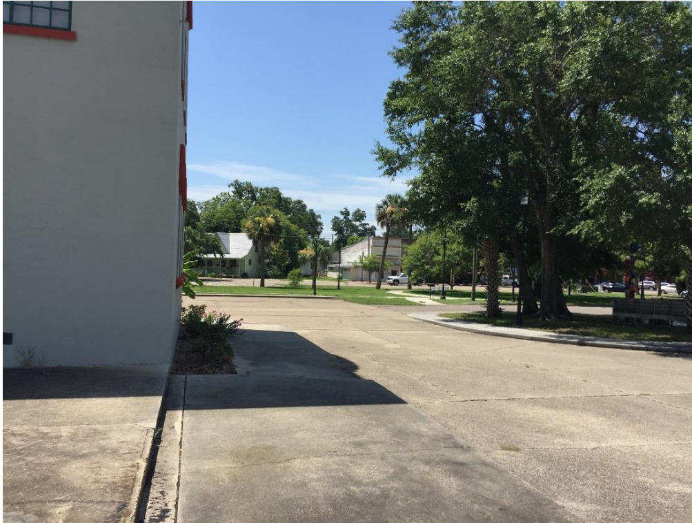
FIG BAS.13 – Non-compliant ADA curb-ramp can be seen along shaded section of sidewalk
