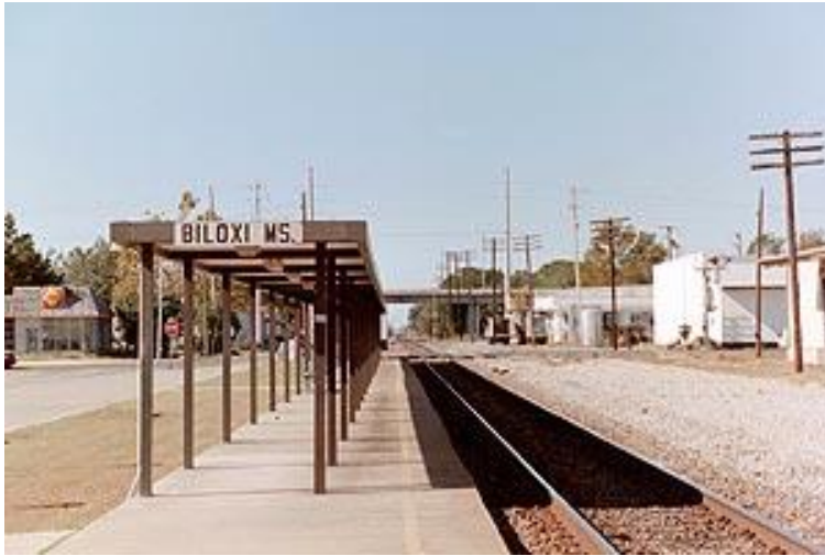
Photo of Station Shelter Looking West
