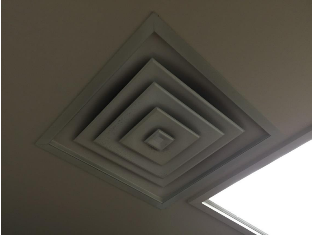
FIG TLH.49 – Ceiling vent in Men’s restroom
