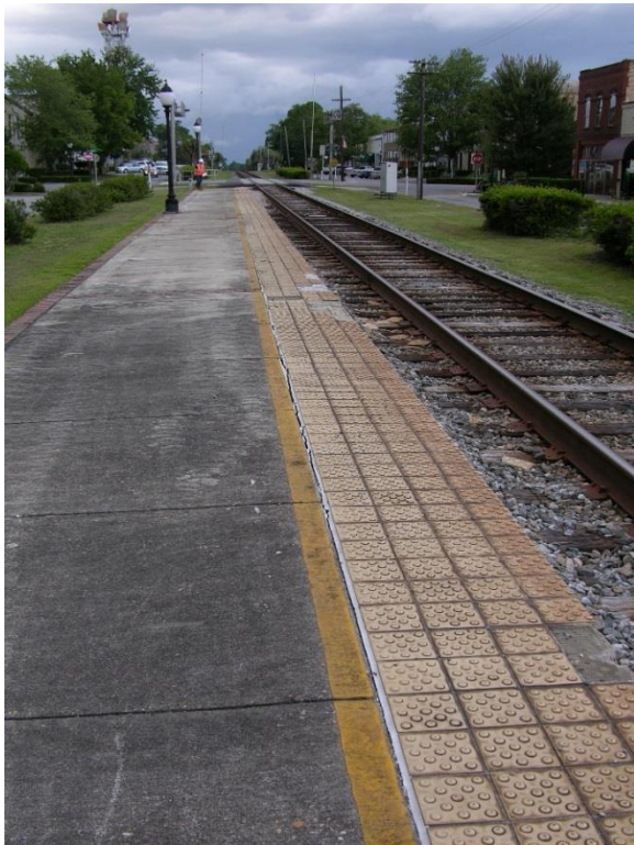
FIG CIP.12 – View from rail crossing at 7 th Street—looking west
