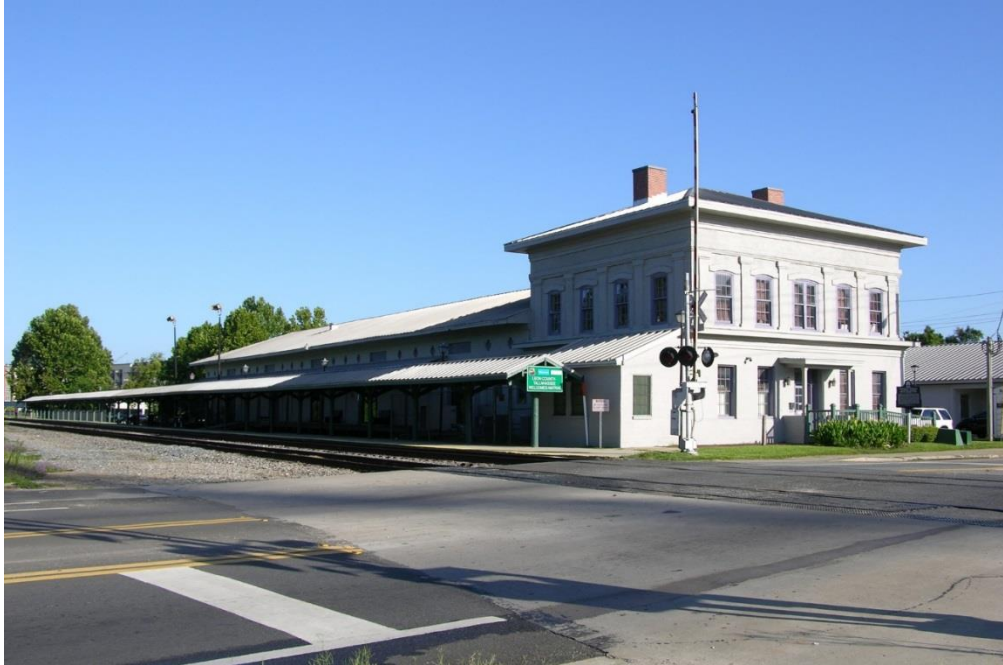
FIG TLH.03 – View of station building / railroad crossing from opposite side of the tracks
