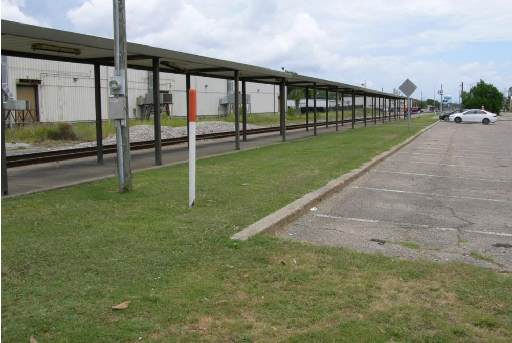
FIG BIX.03 – Parking showing curb and canopy looking east
