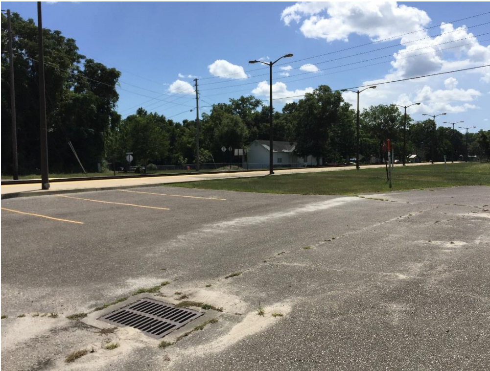
FIG MDO.08 – Site drain located near parking lot vehicle entrance.
