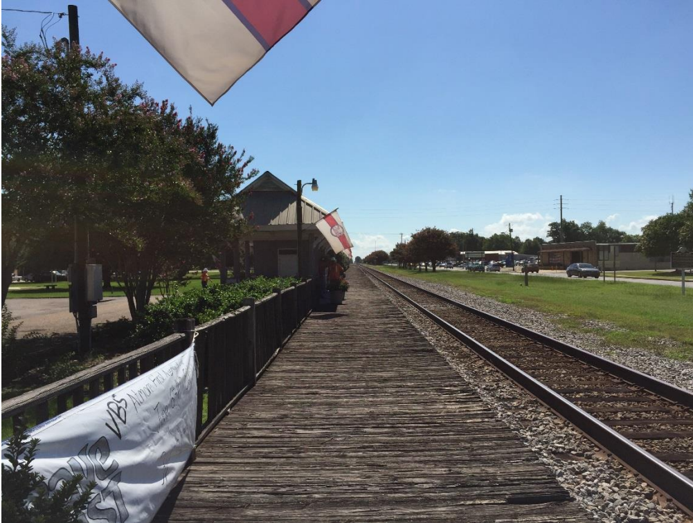
FIG ATR.09 – Existing platform – looking eastward
