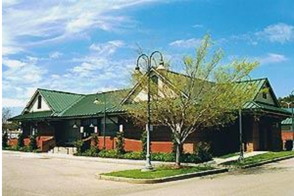
Photo of Station Shelter (Looking North)
