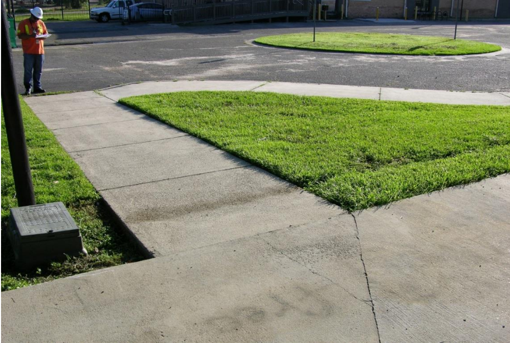
FIG TLH.09 – Curbs, ramps, and sidewalk connecting parking are to platform
