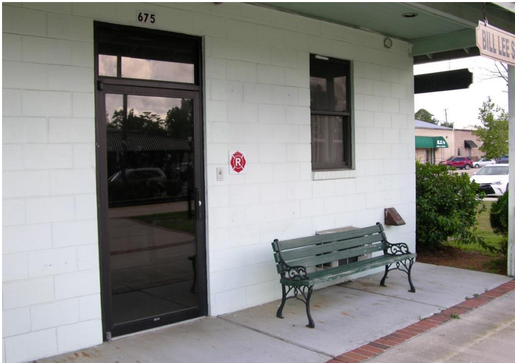
FIG CIP.18 – The door and hardware of Chipley FL station
