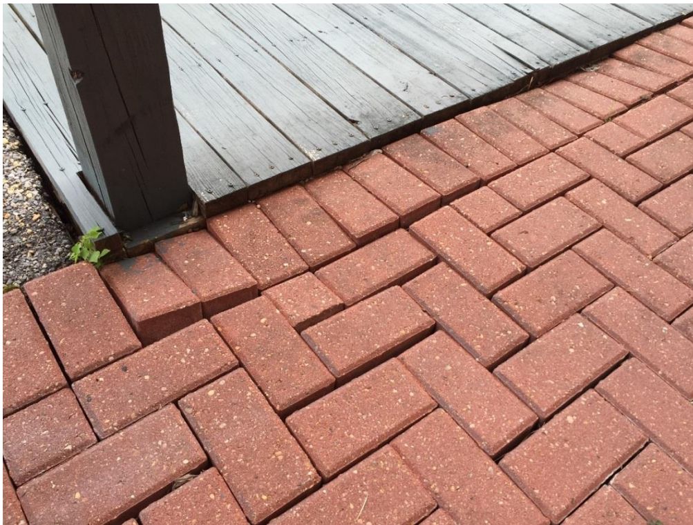
FIG PAG.06 – Close-up view of brick apron
