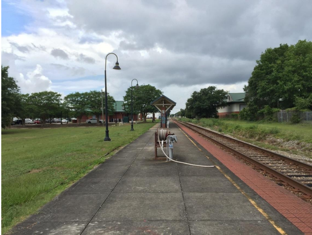
FIG PNS.11 – View from eastern end of platform
