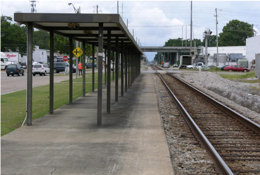
FIG BIX.04 – Platform showing canopy looking west
