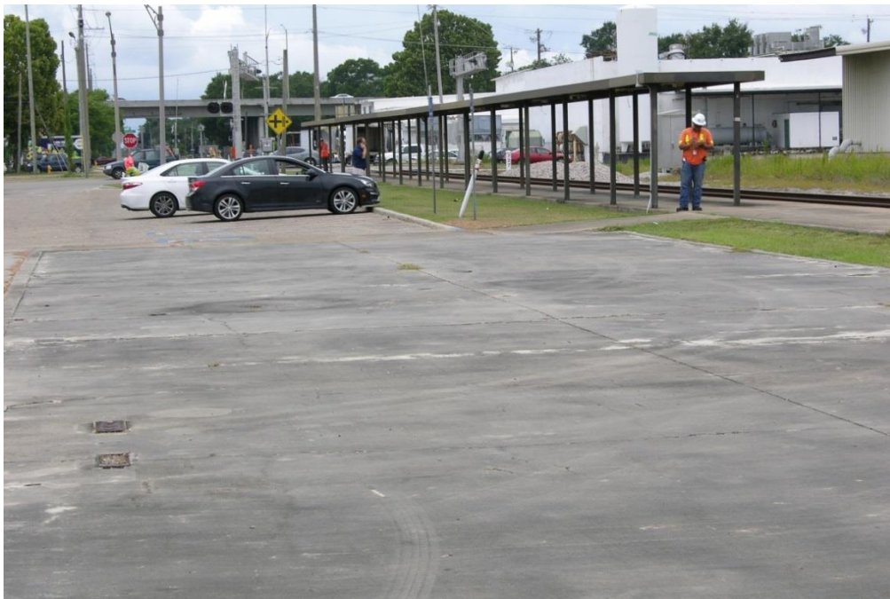
FIG BIX.02 – Parking showing canopy structure looking west – note the remnants of the demolished station building foundation in the foreground of the picture
