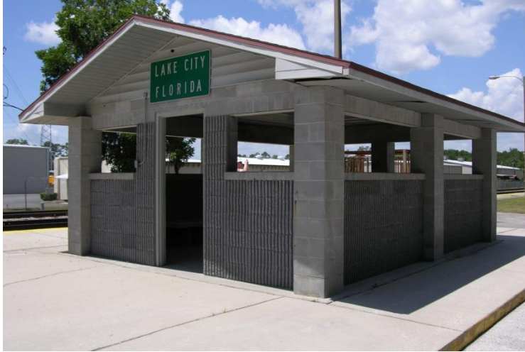
Photo of Station Shelter (Looking Southeast)
