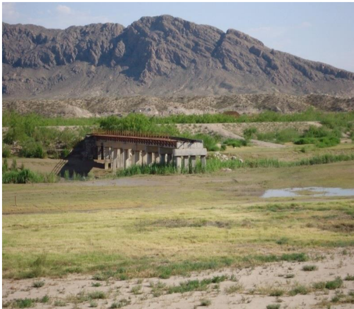
Presidio-Ojinaga International Bridge – the concrete structure is on the Mexican side, while the missing section on the U.S. side was destroyed in a fire (Photo Credit: FRA)
