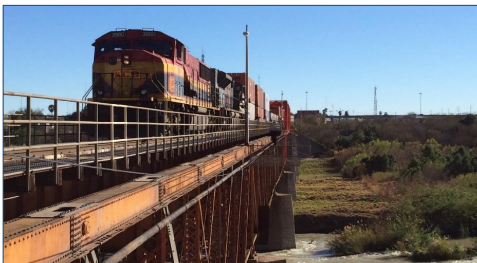
Laredo, TX International Bridge (Photo Credit: FRA)
