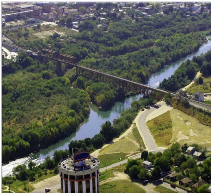
Laredo International Bridge (Mexico on left side) (Photo Credit: FRA)
