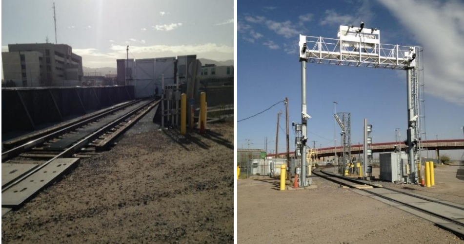
From Left: UP El Paso Bridge on Mexican Side (Photo Credit: FRA); UP El Paso Bridge on U.S. side (Photo Credit: FRA)
