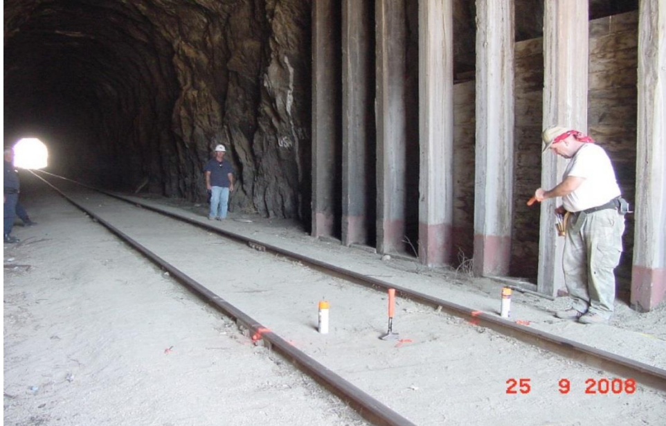
Campo Border Crossing – view at the end of tunnel is the U.S. side (Photo Credit: International Boundary & Water Commission)
