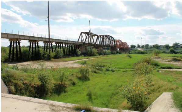
UP International Railroad Bridge in El Paso, TX (Photo Credit: FRA)
