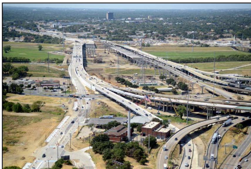
Figure 3-15: Reconstruction of I-30/I-35E Interchange
