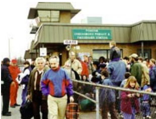
Figure 6-12: Existing Greensboro Station
