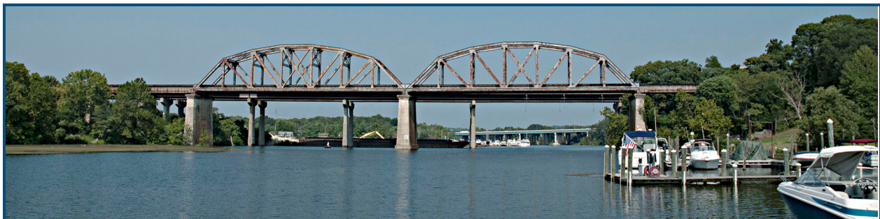
Occoquan River Bridge
