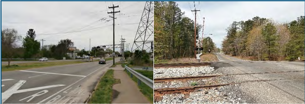
Figure 3.15-4. Examples of Public At-Grade Crossings in the DC2RVA Corridor
