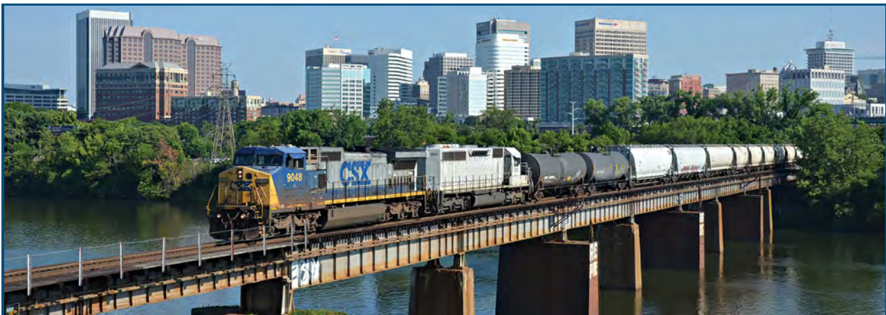
James River Bridge
