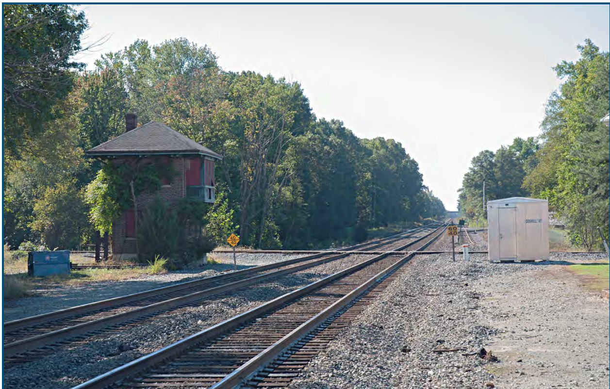
Existing Corridor in Area 4: Central Virginia
