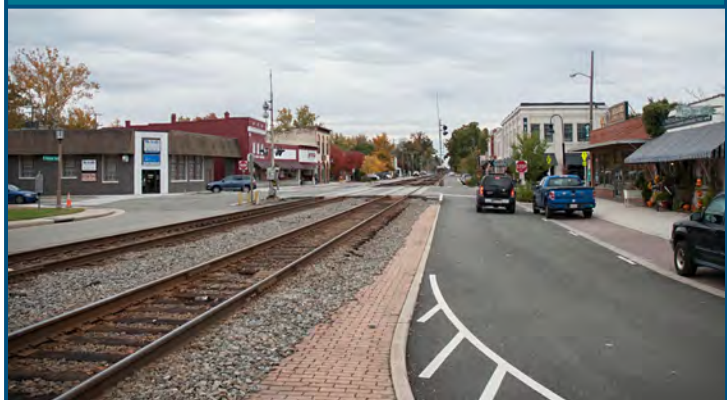
View of Tracks through Downtown Ashland
