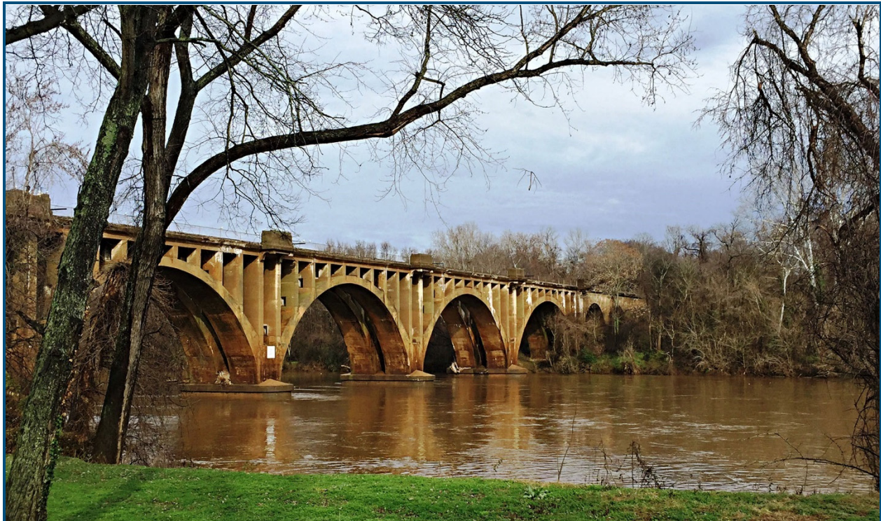
Existing Rappahannock River Railroad Bridge
