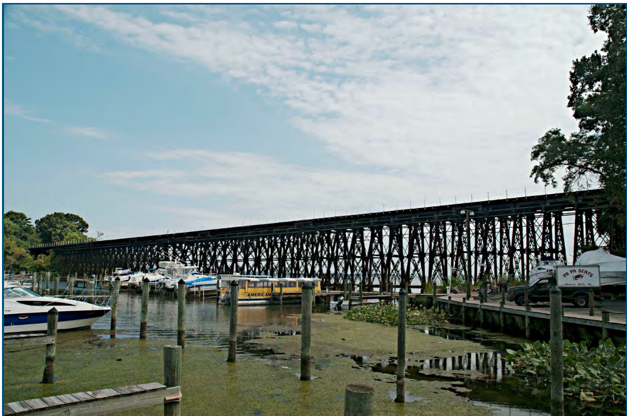
Rail Bridge Over Neabsco Creek
