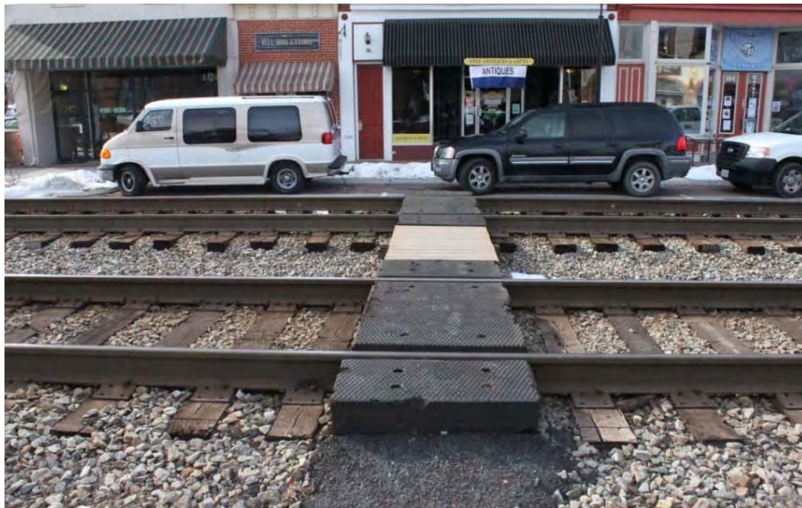
FIGURE 7-2: AT-GRADE PEDESTRIAN CROSSINGS
