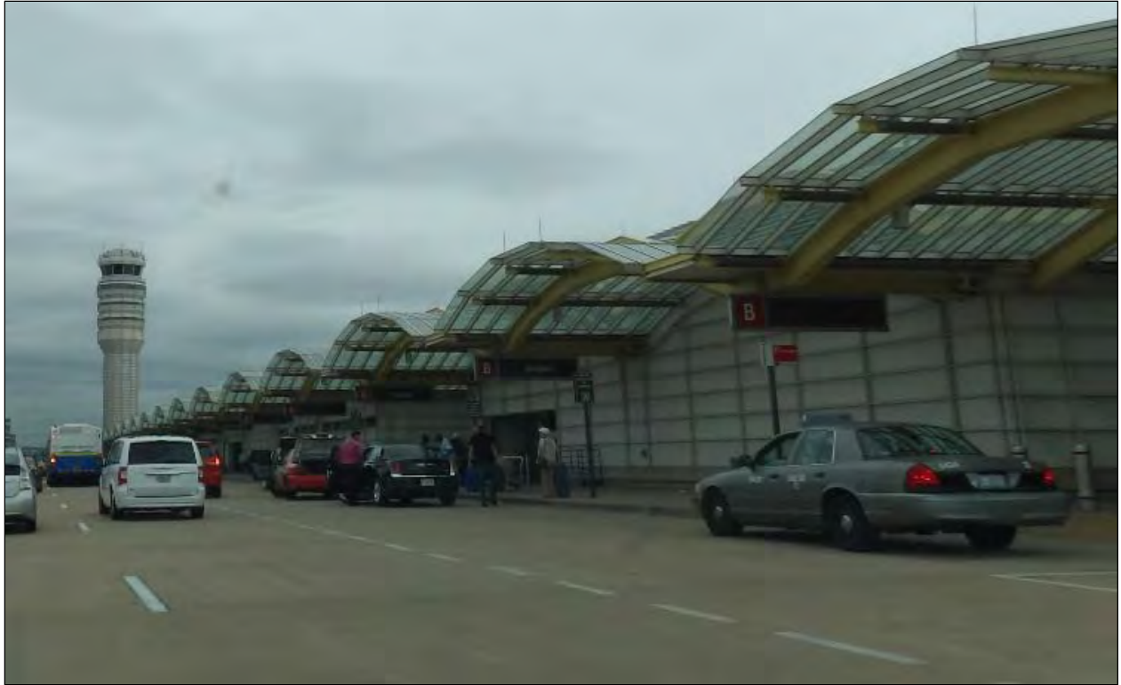
FIGURE 5-12: WASHINGTON NATIONAL AIRPORT TERMINAL AND SOUTH HANGAR LINE (000-0045)
