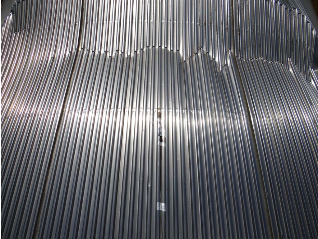
Figure B21. Post-test — Roof Buckle near Section 8
