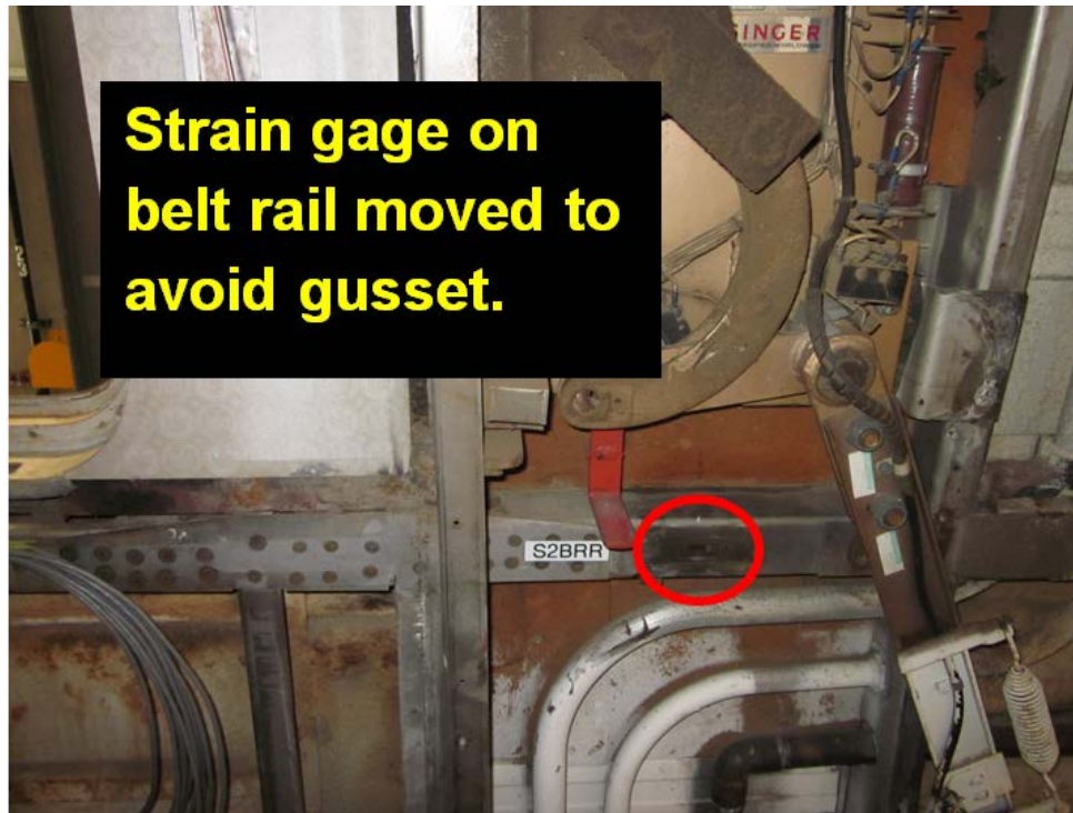
Figure B5. Strain Gage on Belt Rail
