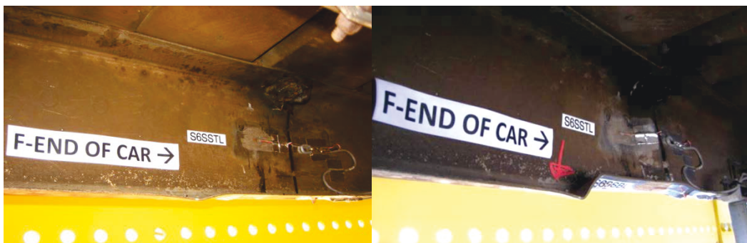
Figure 68. Pre- (left) and Post- (right) Test Photographs of Left Side Sill, Cross-Section 6
