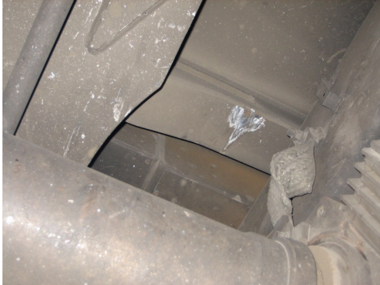
Figure A.2.1-11. Scar on Carbody Above B End Outboard Axle Bearing Housing
