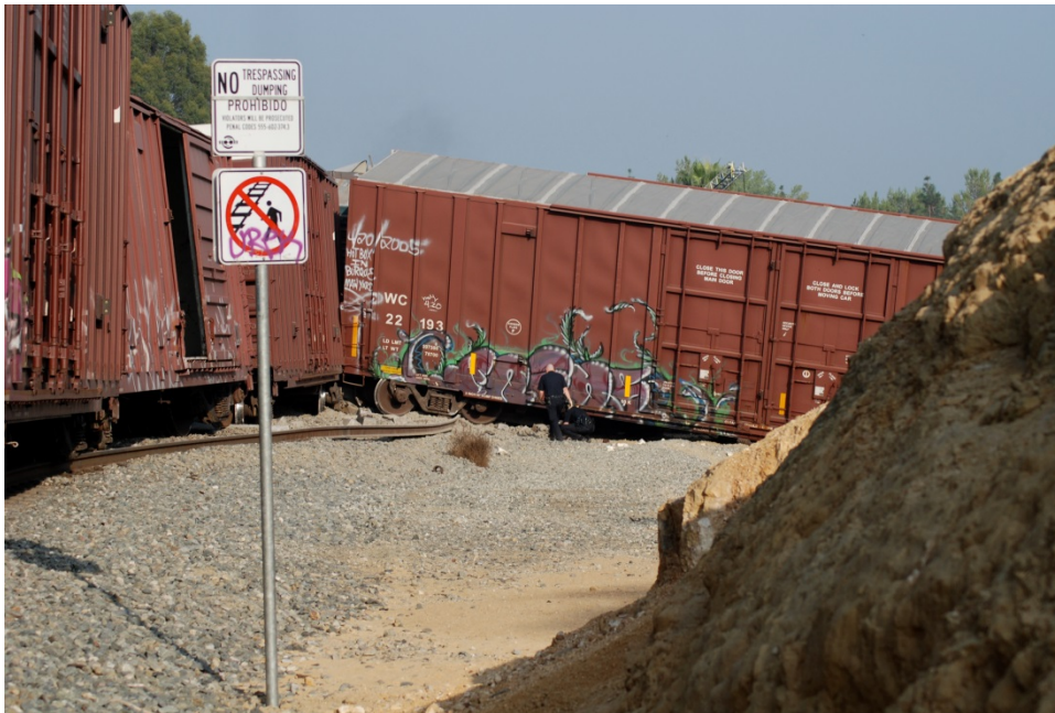
Figure A.2.2-8. Displaced Rail and Derailed Freight Cars
