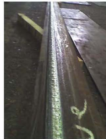
Photograph 10: Completed Rail Glaze
