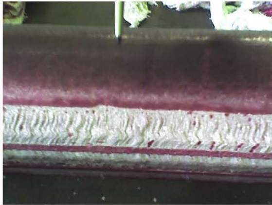
Photograph 12: Dye Penetrant Inspection Showing Center Section of Rail With Clean Ground Surface.
