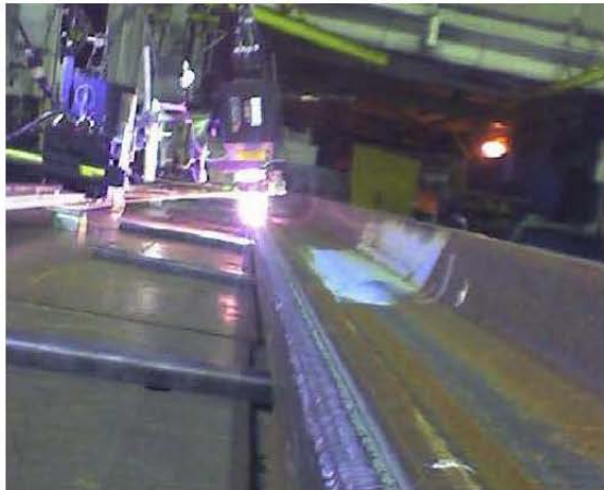
Photograph 9: In Process Gazing of Entire 40' Section.
