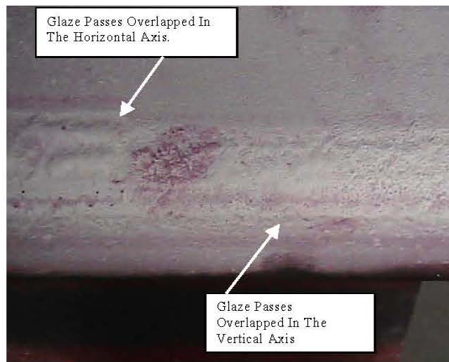
Photograph 4: Dye Penetrant Testing Of Overlapping Sections
