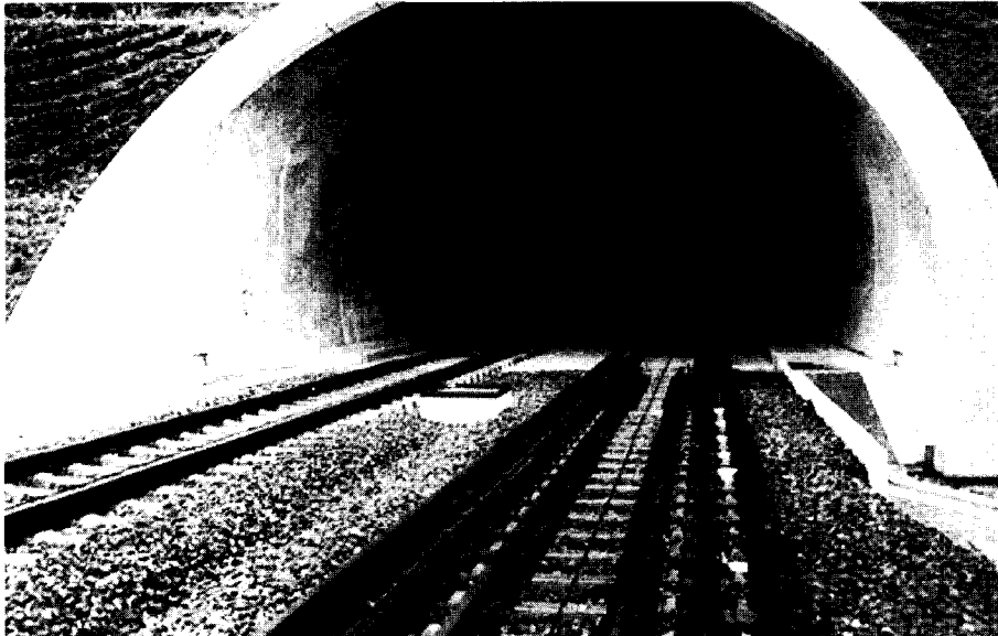
Figure 6. Transition Section Which Utilized Additional Rails, DB (Schrewe, 1987)
