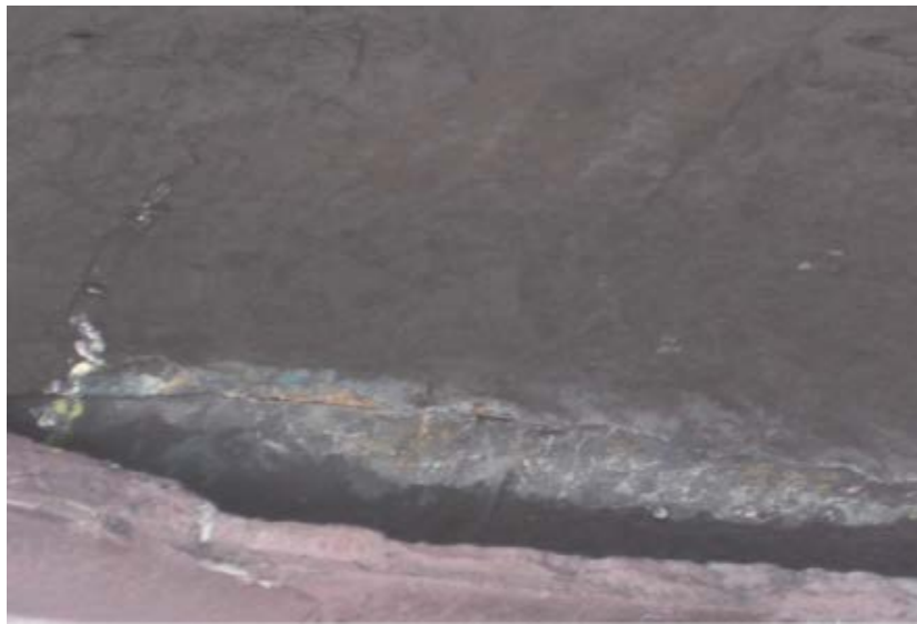
Figure 6: Burn through of tank shell located at the outboard A-end right side of draft sill.
