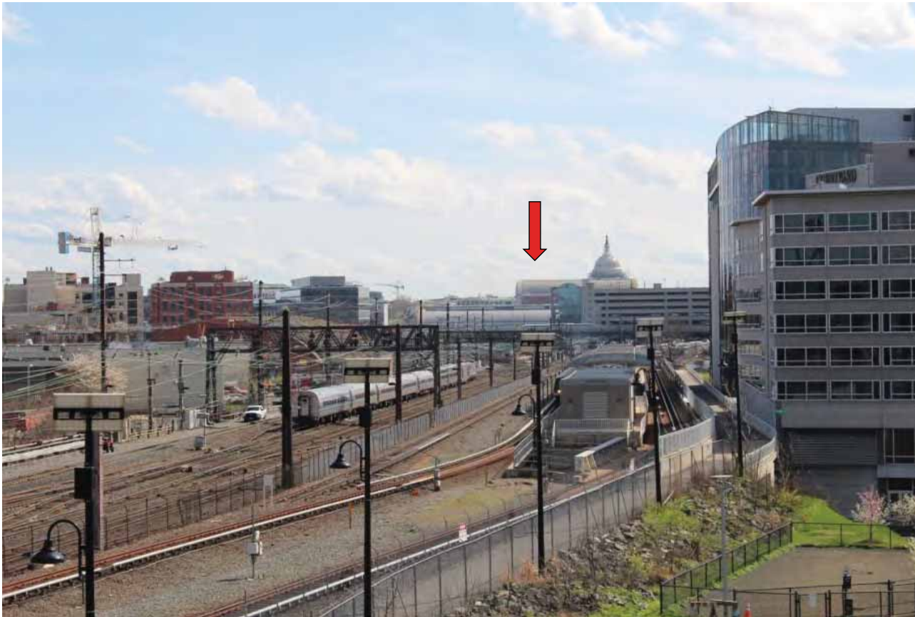
View looking south to WUS and Terminal Rail Yard from New York Avenue NE
