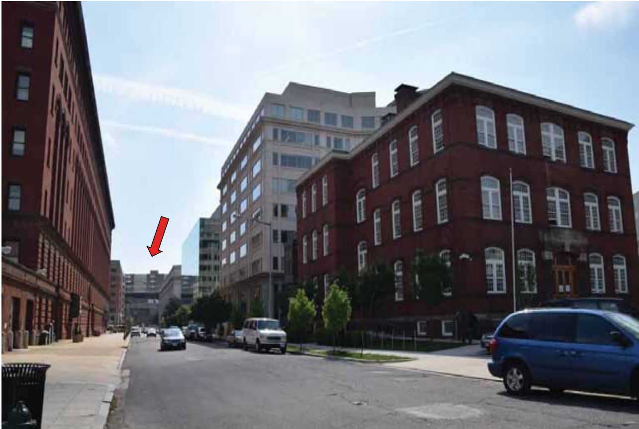
View looking east towards the WUS parking garage from G Street NW and Massachusetts Avenue
