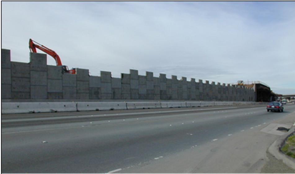
Figure 11: MSE Wall, Route 85/US 101 (South) Interchange Project, CA
