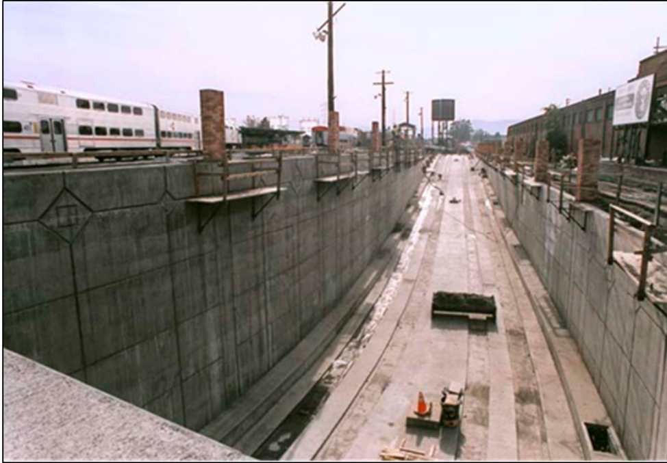
Figure 10: Trench Diridon Tunnels, San Jose, CA
