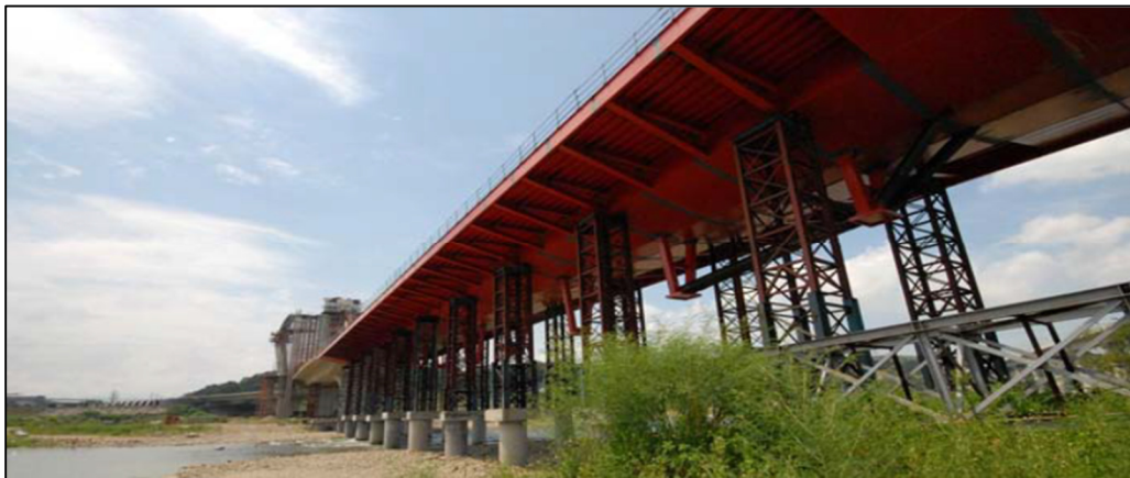
Figure 3: Staging and Falsework Supporting the Formwork for In Situ Construction ( Photo courtesy of Taiwan High-Speed Rail Corporation [THSRC] )
