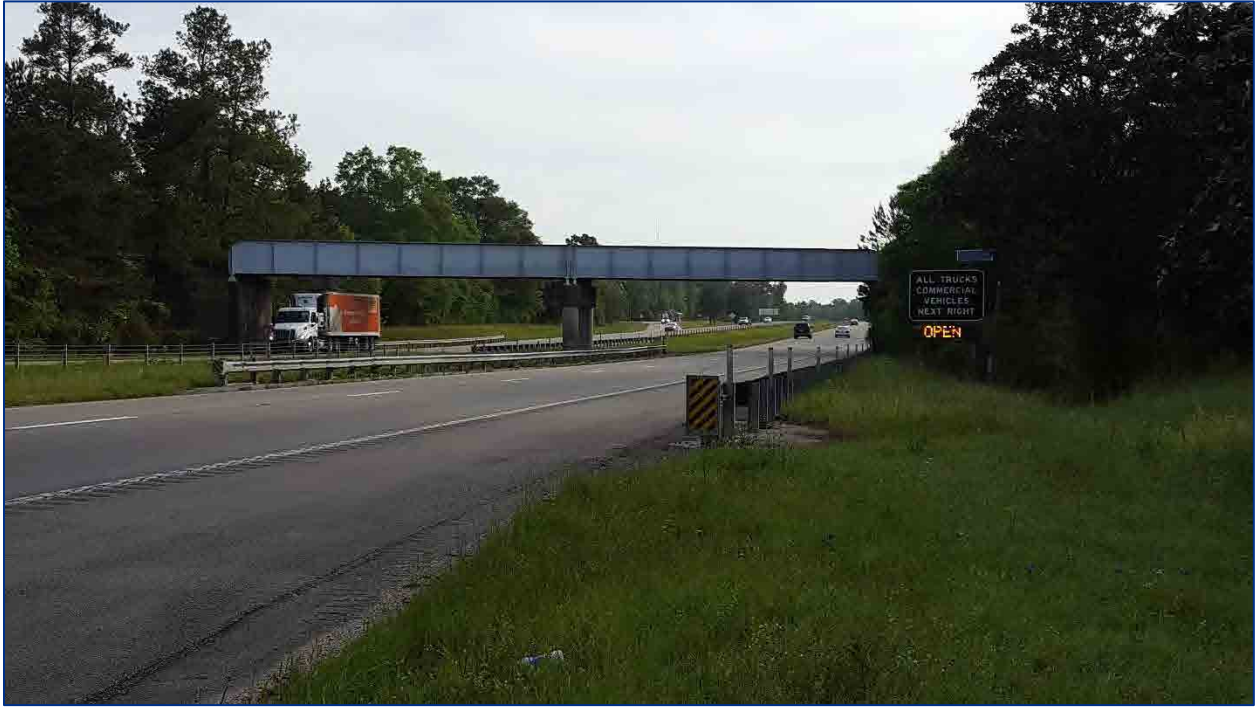
Figure 6-10: Resource 2, Looking North
