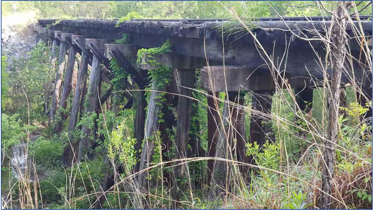
Figure 6-7: Resource 1, Looking North
