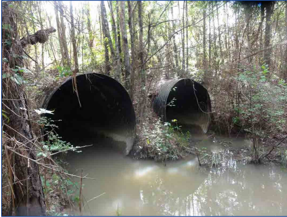
Figure 6-13: Resource 3, Looking East
