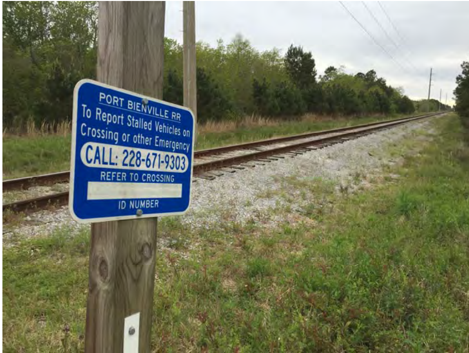
Photo 9 - Existing Port Bienville Railroad (near south project tie-in)
