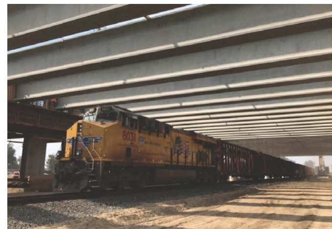
San Joaquin Viaduct
