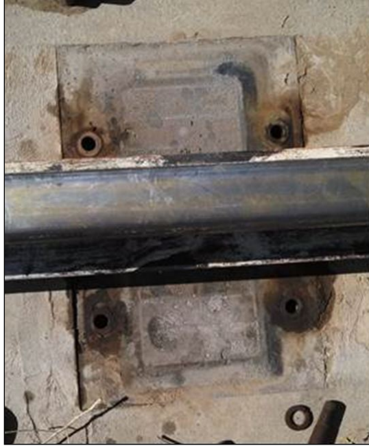
Figure 22. Concrete Slab Under a DFST Fastener
