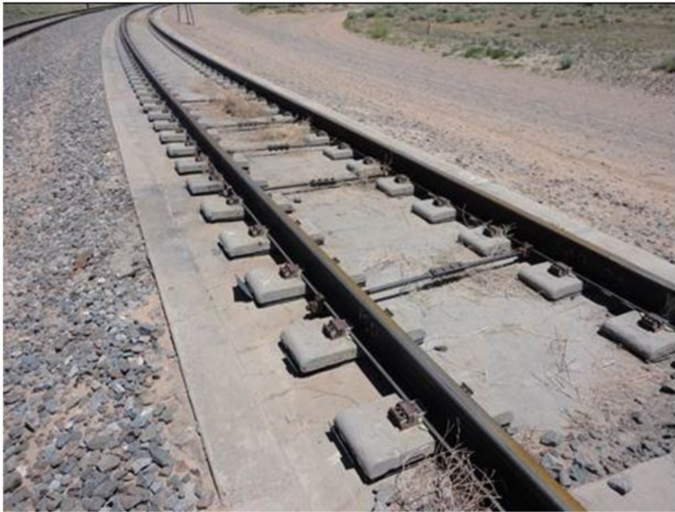
Figure 2. Installation of Gage Rods in IDBT Section at Curve Spiral
