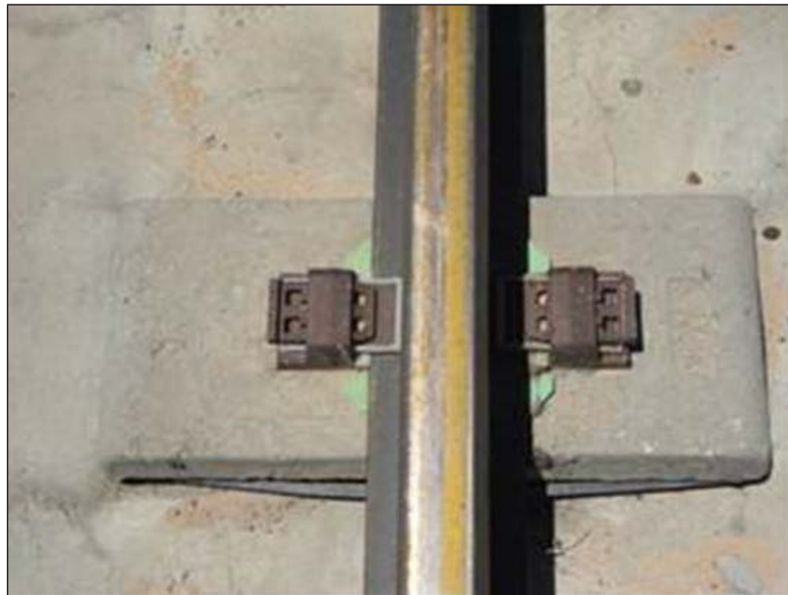
Figure 13. Typical IDBT Fastener Installation
