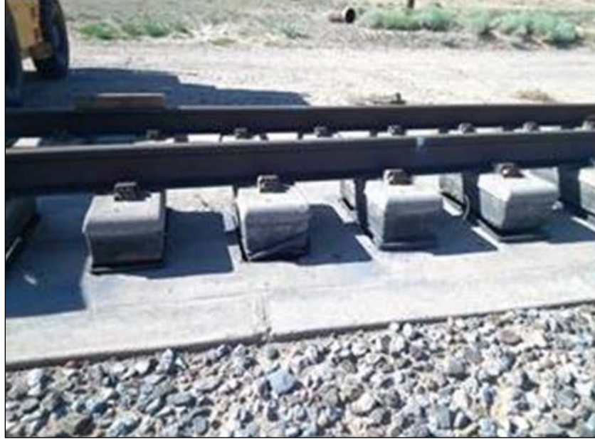
Figure 14. Concrete Boots for the IDBT Fastening System
