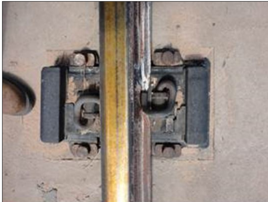
Figure 19. Typical DFST Fastener Installation
