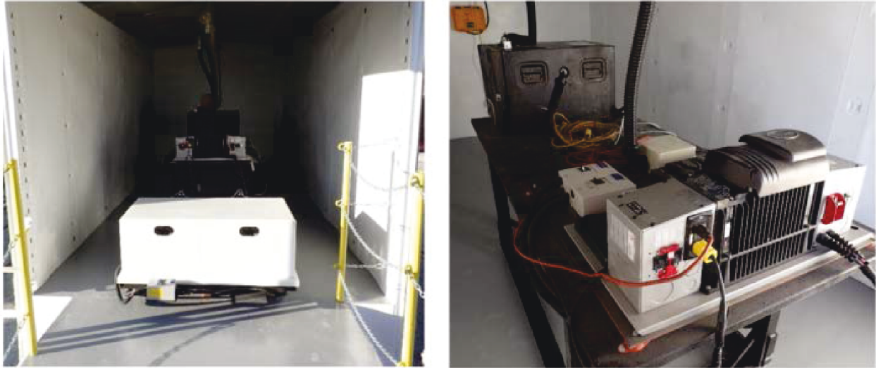
Figure 51: Freight ATGMS Power System Installation
