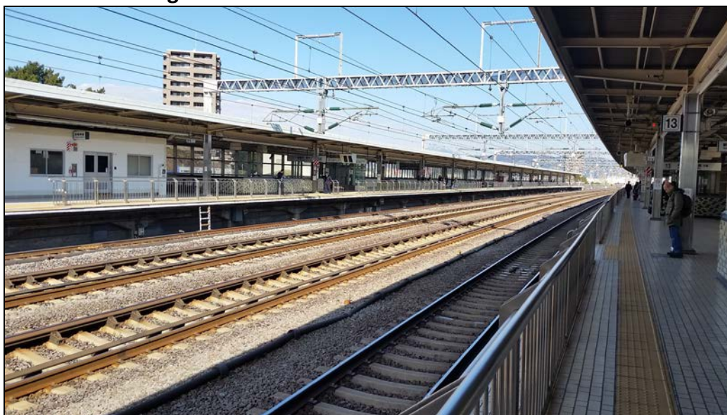
Figure 2-11: Station Platform Infrastructure
