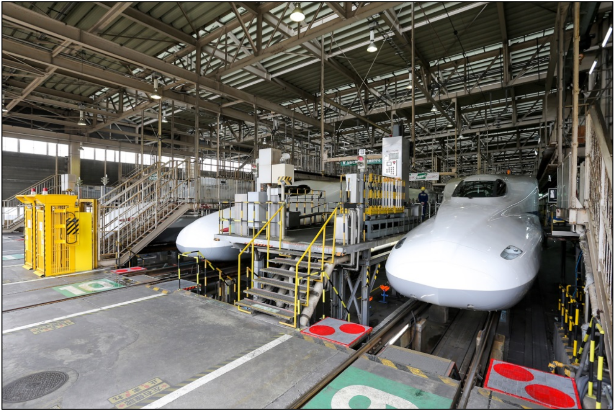
Figure 2-13: Trainset Maintenance Facility
