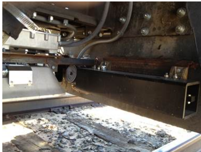
Figure 11. Transponder Scanner Antenna and Track Receiver
