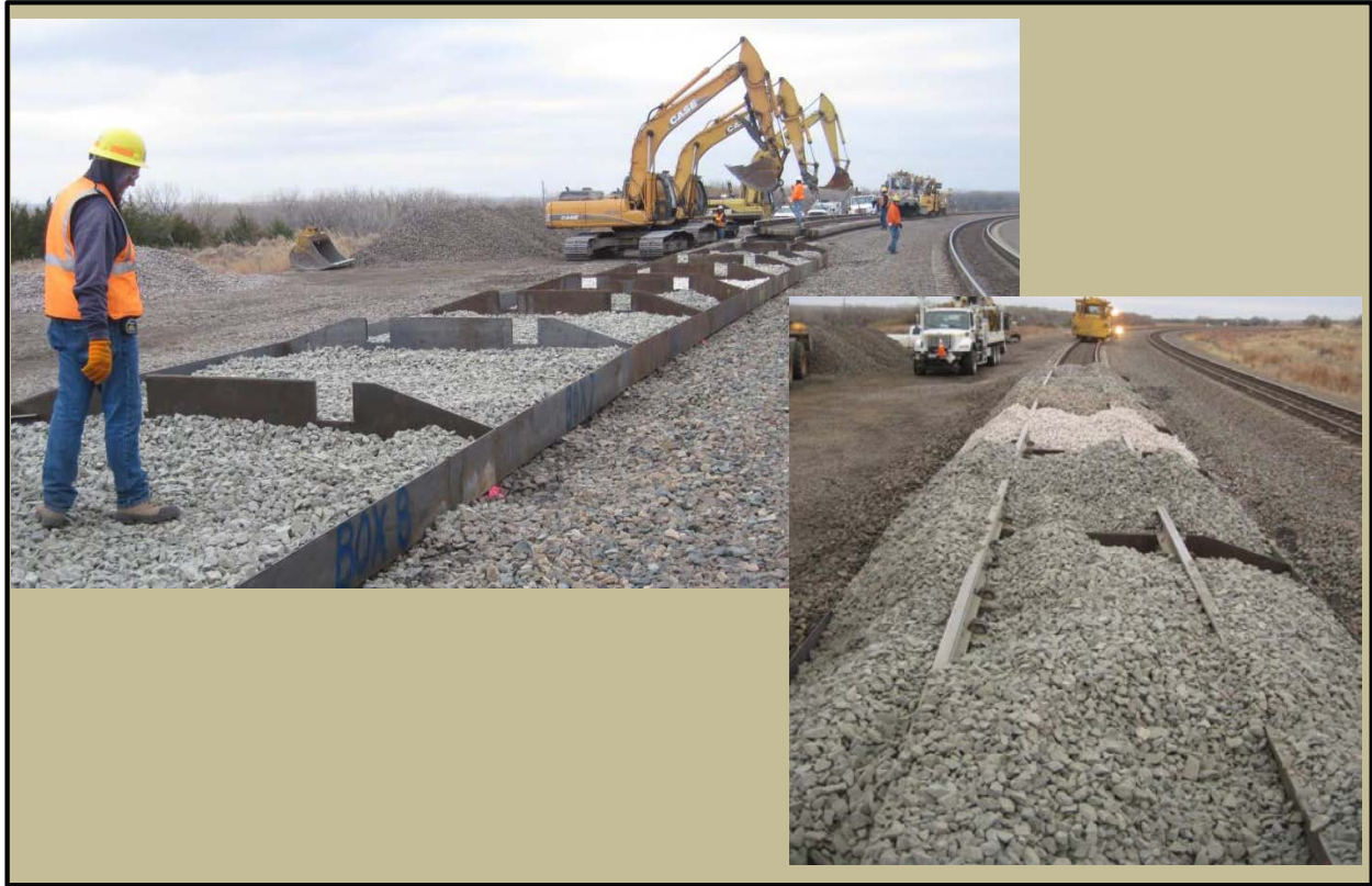
Figure 13. Installation of the UP Ballast Box Test
