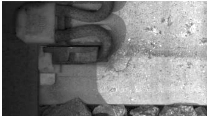
**Figure A-2. Example of a Typical Clip Crack**
