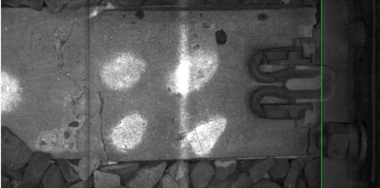
**Figure A-9. Example of a Typical Mid Gauge Crack**
