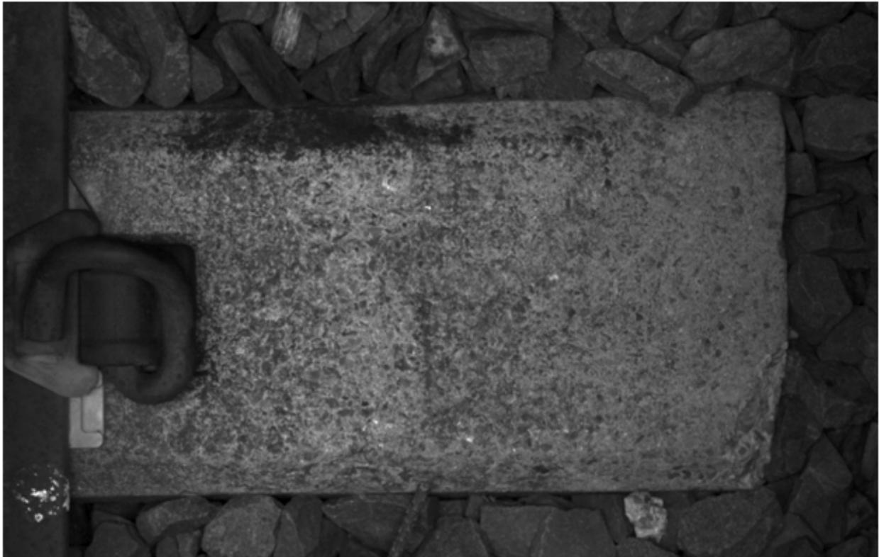
**Figure B-3. Tie Shoulder with Minor Chip on One Corner—Tie Grade = 1**
