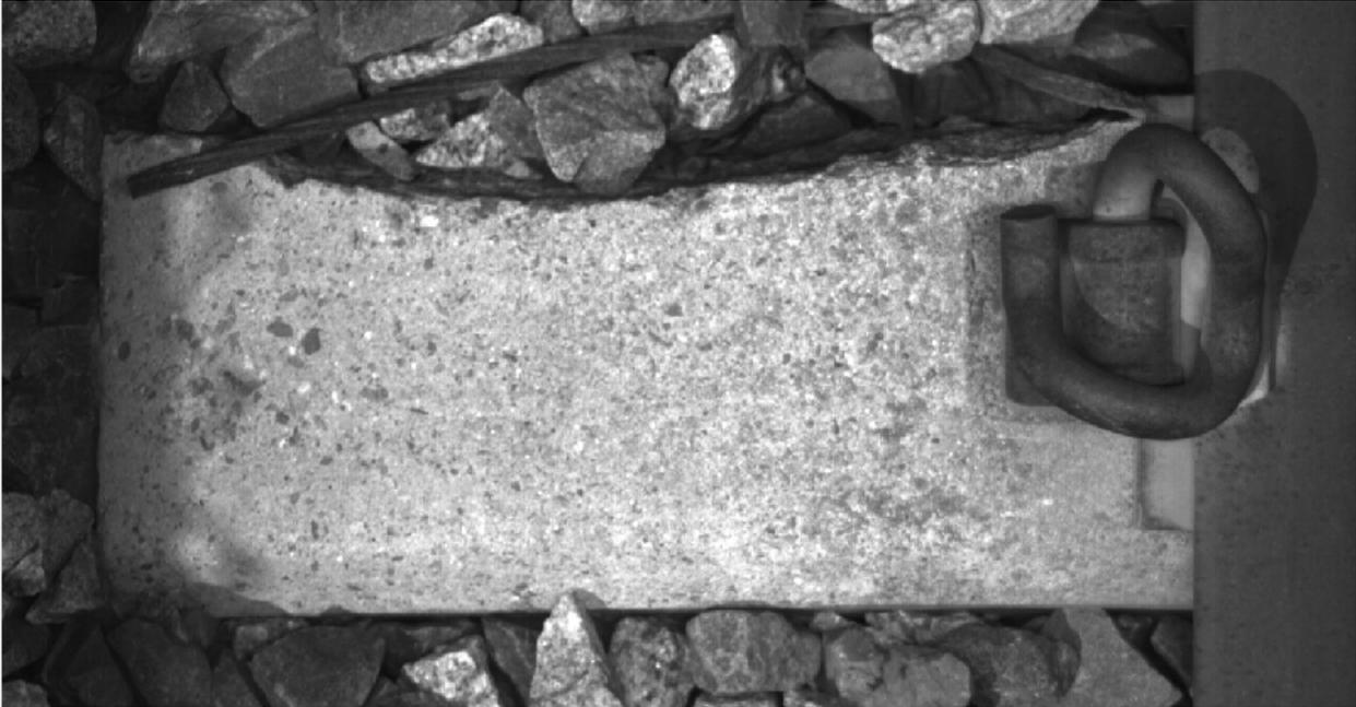
**Figure B-15. Tie with One Pre-Tensioning Wire Exposure Site—Tie Grade = 4**
