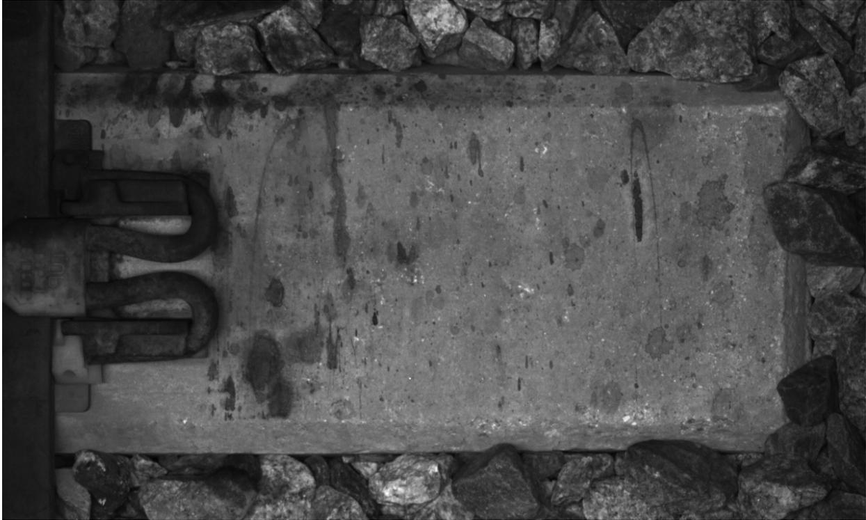
**Figure B-4. Tie Shoulder with Surface Contamination—Tie Grade = 1**
