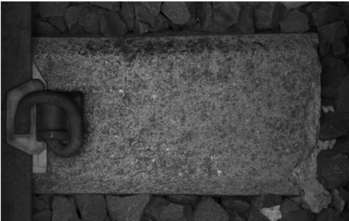
**Figure B-5. Tie Shoulder Exhibiting Preliminary Signs of Crumbling Impacting Less Than 10 Percent of Shoulder—Tie Grade = 1**
