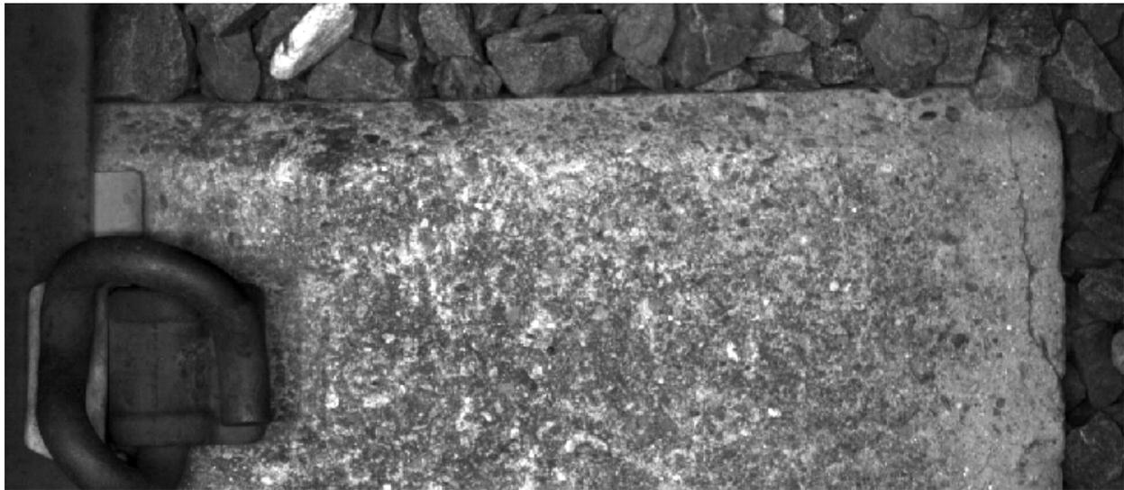
**Figure A-4. Example of a Typical End Crack**
