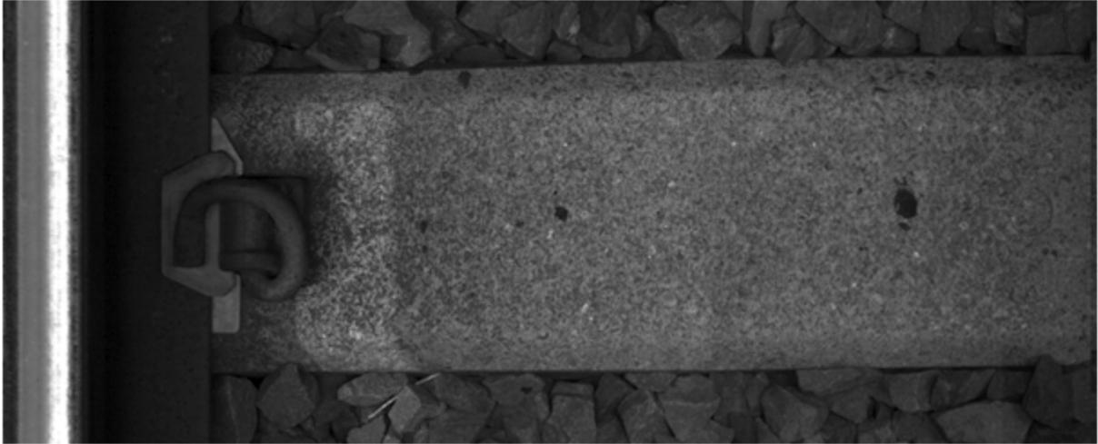
**Figure B-2. Section of Tie Between the Rails in Excellent Condition —Tie Grade = 1**
