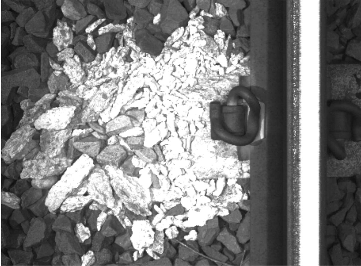
**Figure B-21. More Than 60 Percent of Tie Shoulder in Crumbled State—Tie Grade = 5**
