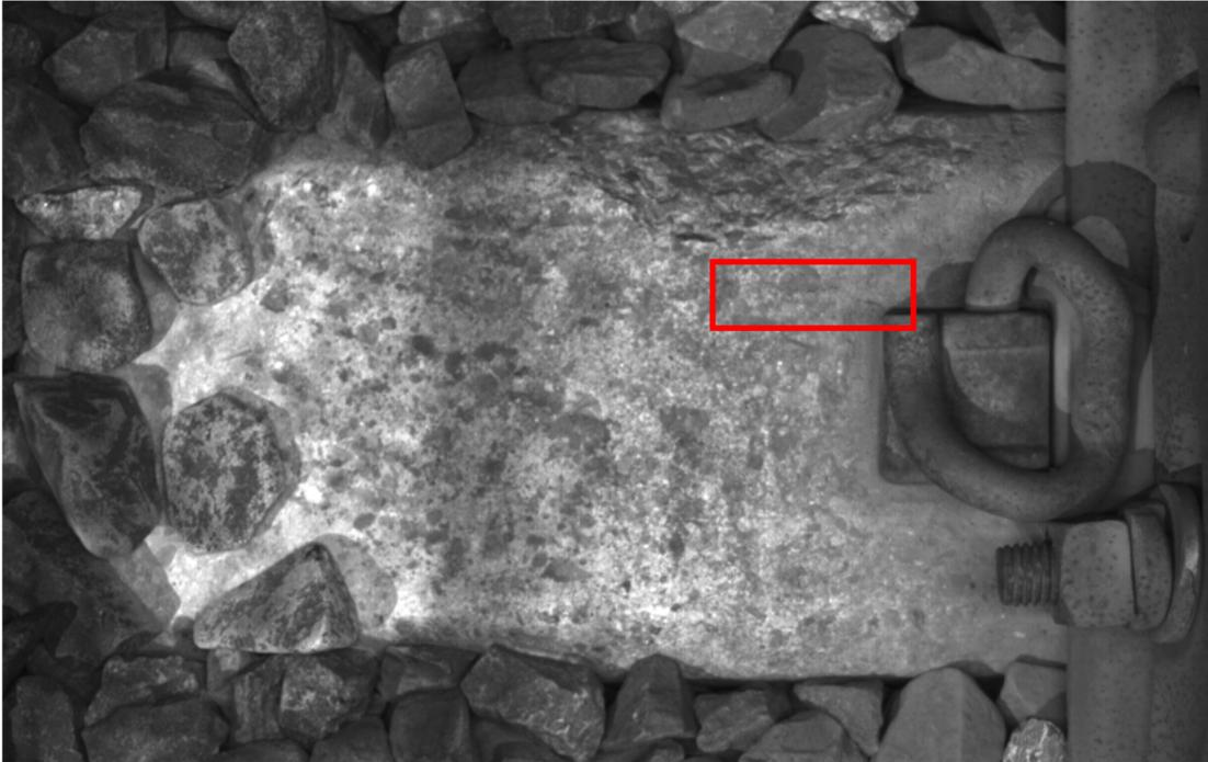
**Figure B-9. Tie Chip Not Reducing Width of Rail Seat Zone by More Than 1 Inch, One Rail Seat Zone Impacted by a Crack, and Total Crack Length Less Than 9 Inches—Tie Grade 2**
