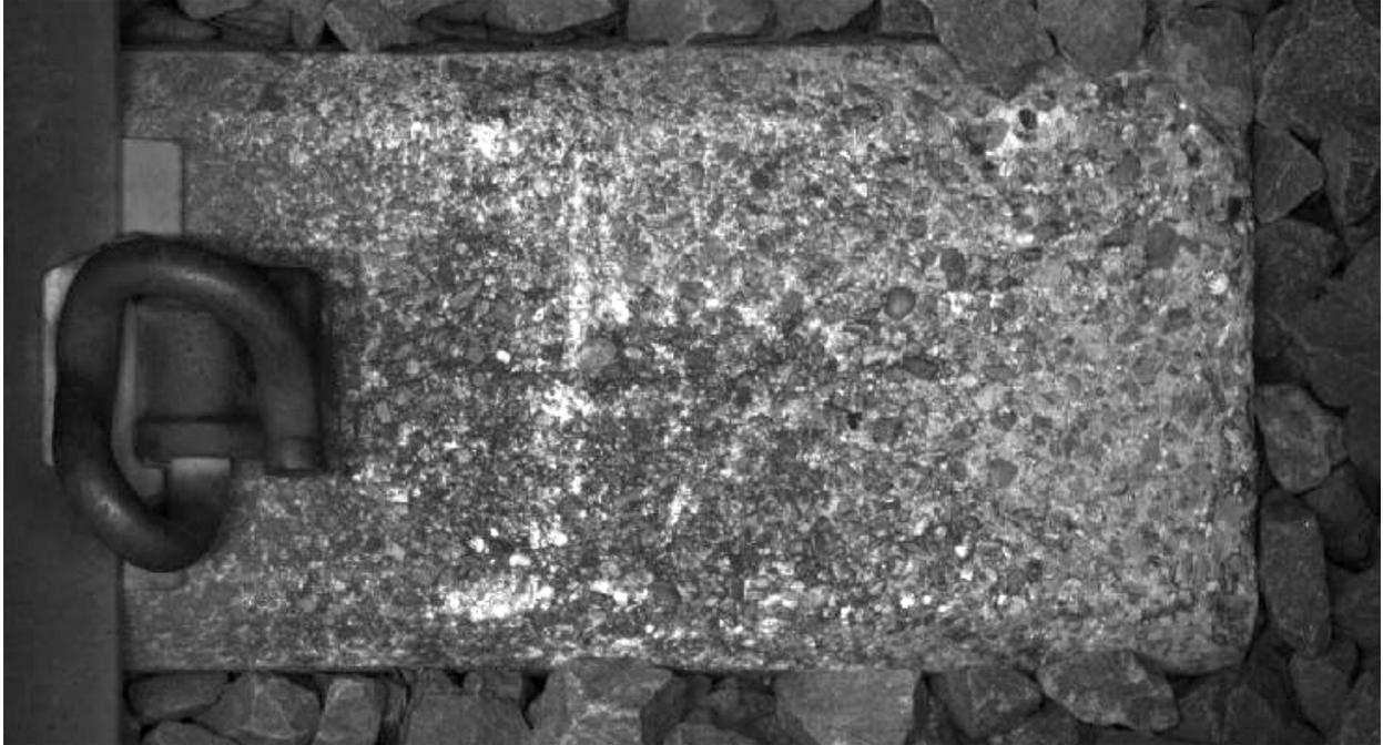
**Figure A-5. Example of a Typical Eroded Crack**
