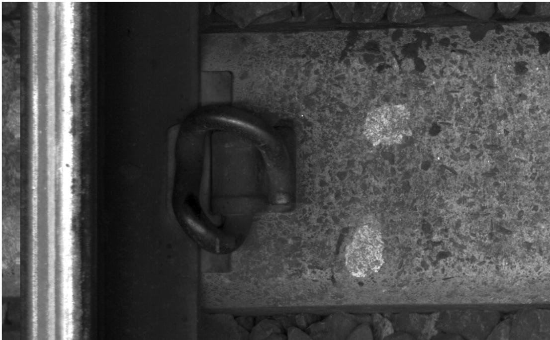
**Figure B-10. Marking Between the Rails (Two White Dots) Applied by Amtrak to Indicate a Tie Grade 2 for the Tie Shown in Figure B-9**
