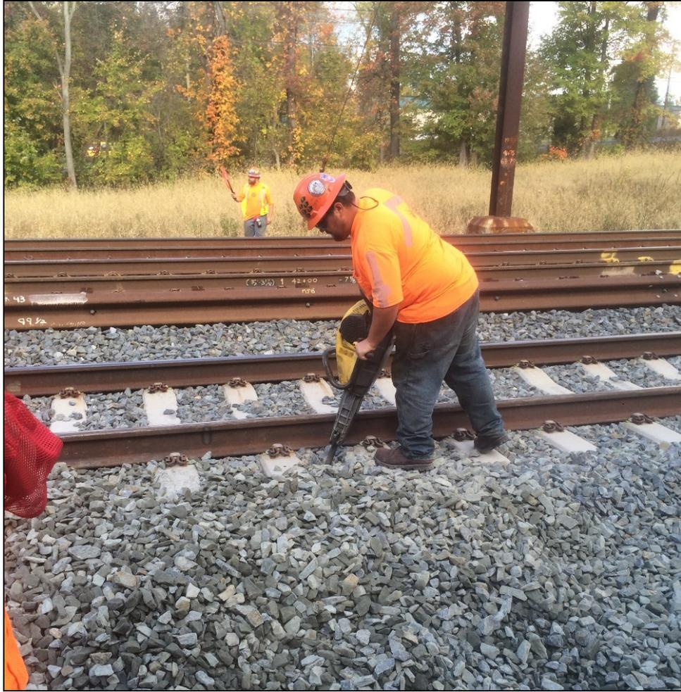
**Figure 69: Tamping the Ballast Around the Ties**
