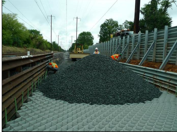
**Figure 25: Geocell Layer and Infill Material**
