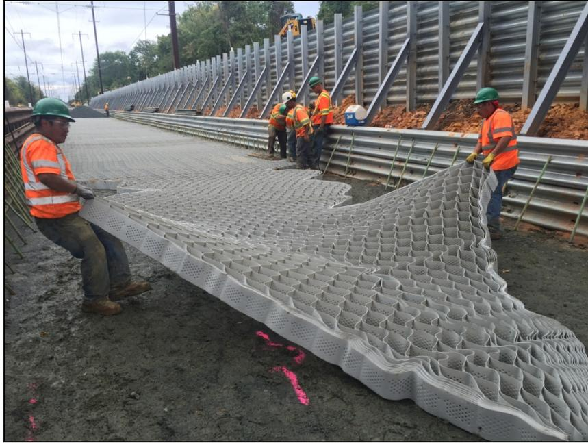
**Figure 23: Opening the Neoweb™ Material**
