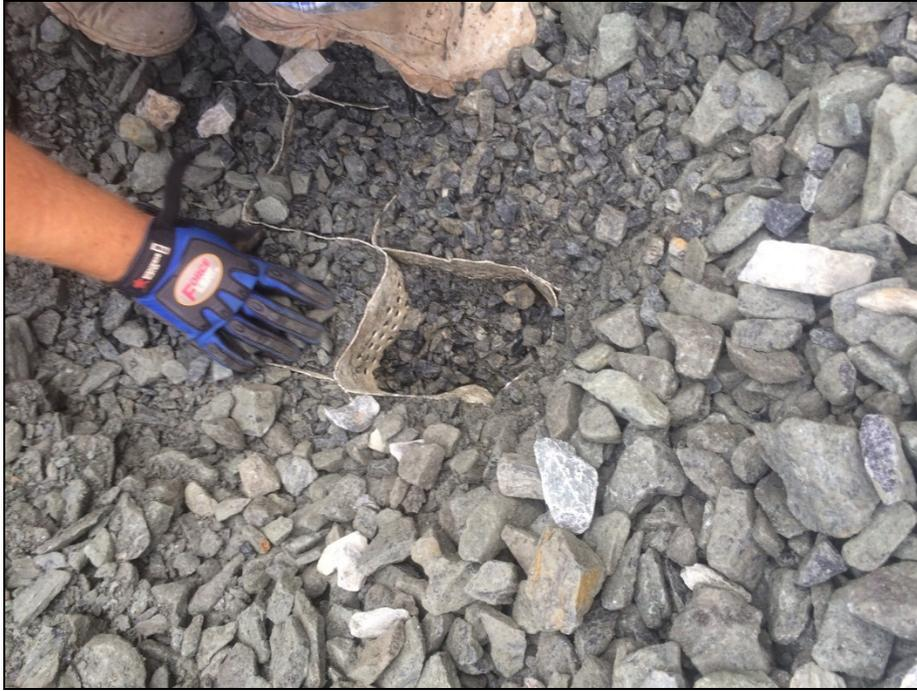
**Figure 64: Removing the Sub-Ballast by Hand**
