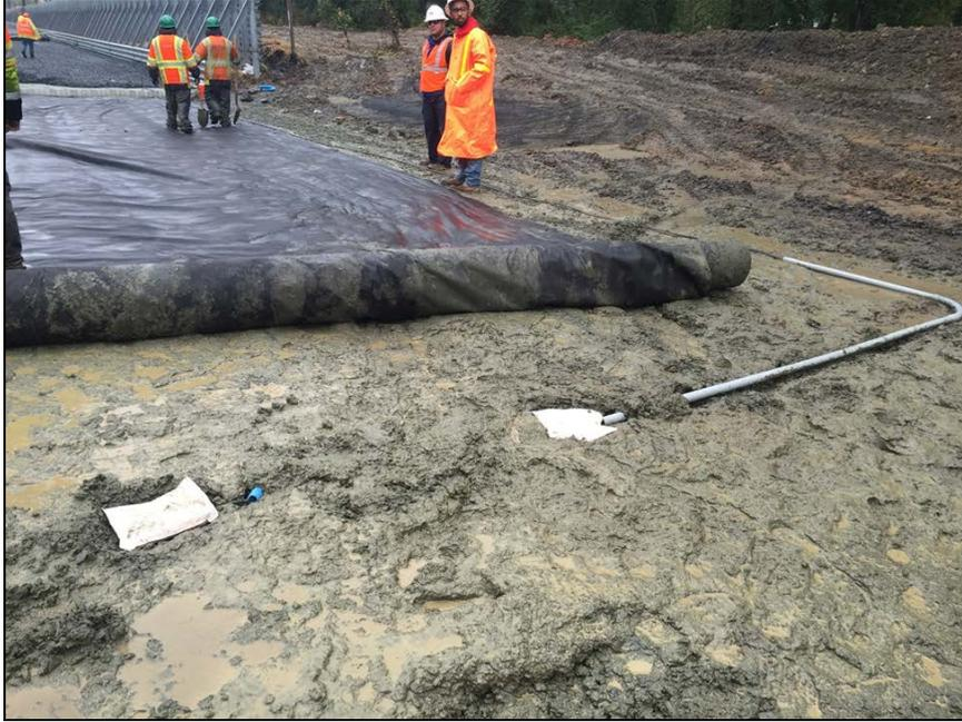
**Figure 33: Pressure Cells in Zone Without Geocell Material**
