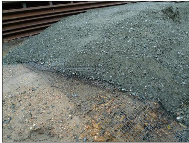
**Figure 28: Overlapping Biaxial Geogrid Layers at End of Reinforced Zone**
