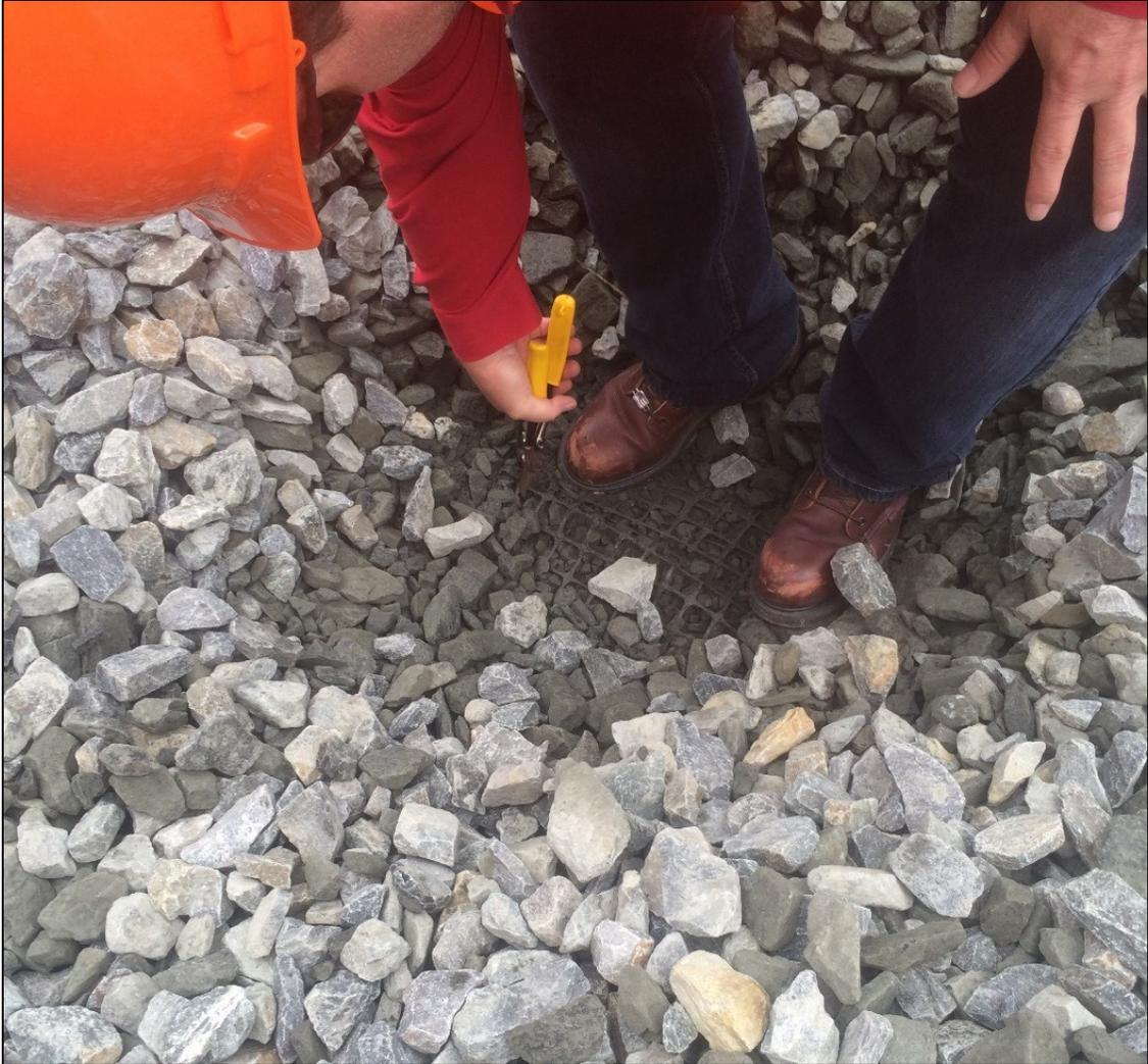
**Figure 58: Geogrid Layer Installed Between the Ballast and Sub-Ballast**
