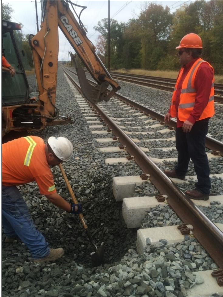
**Figure 62: Hand Held Tools Were Used to Reach the Geocell Material Without Damaging It**
