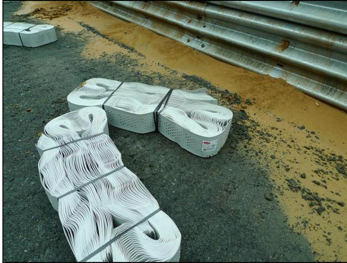
**Figure 21: Geocell Ready for Deployment**
