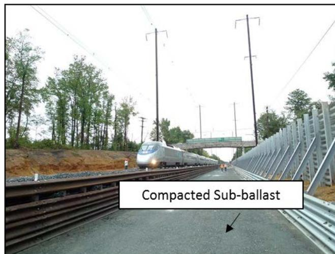
**Figure 20: Compacted Sub-Ballast Layer**
