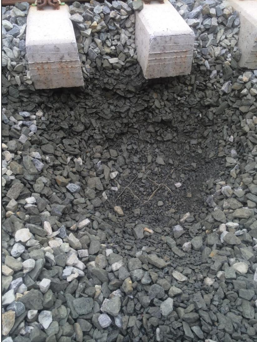
**Figure 63: Top Surface of Geocell Layer**
