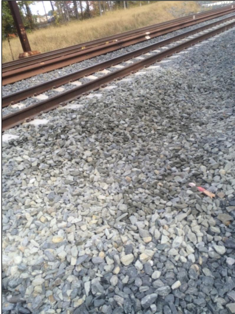
**Figure 70: Second Pit Completely Covered and Tamped**
