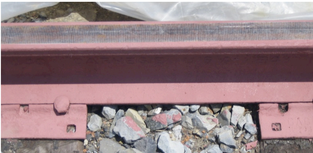
Figure 12. Red Metallic Primer Coating
