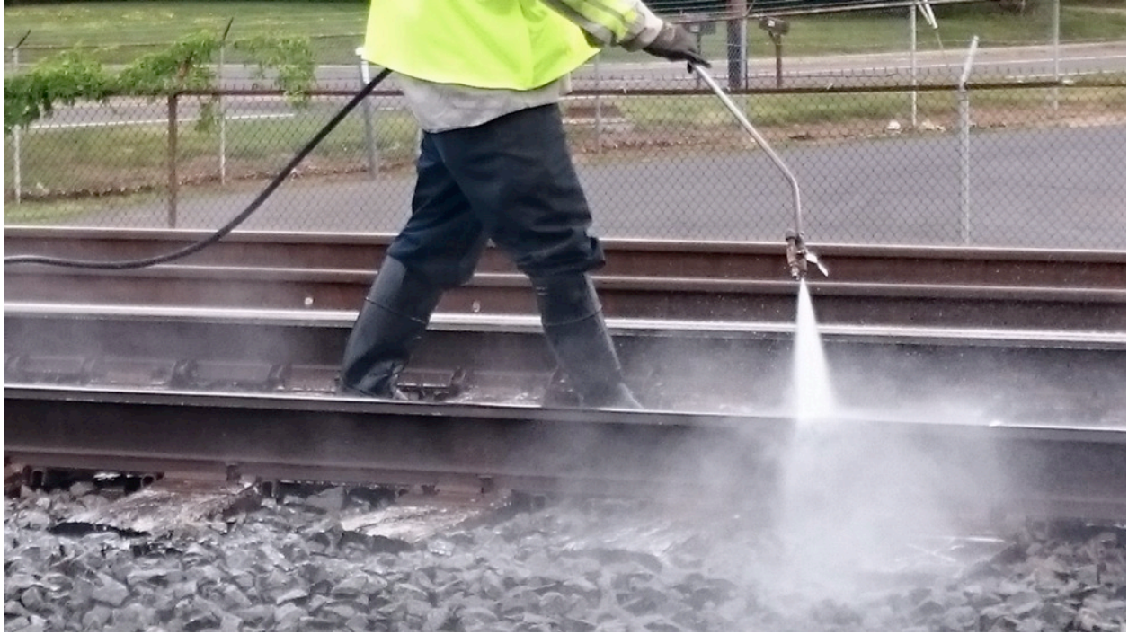
Figure 14. Surface Preparations Before Coating Using High Pressure Power Washing
