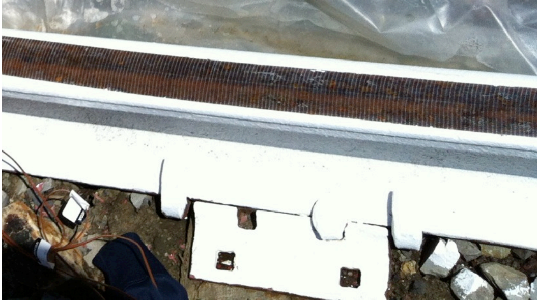
Figure 13. White Reflective Coating
