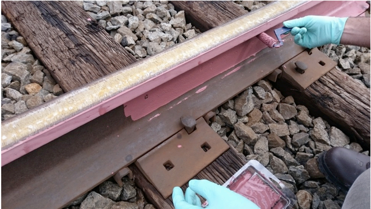
Figure 16. Application of Red Metallic Primer to Rail with Roller
