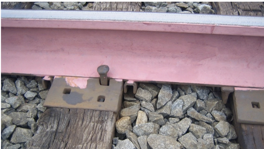
Figure 17. Dried Red Metallic Primer Coating on Rail
