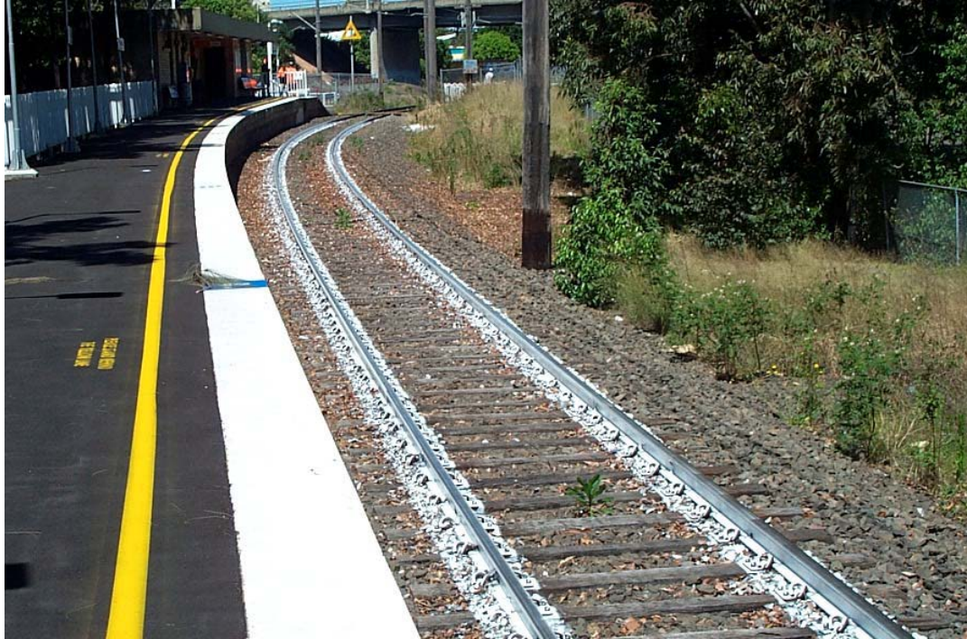
Figure 1. Coated Rails Near Sydney in Australia [19]
