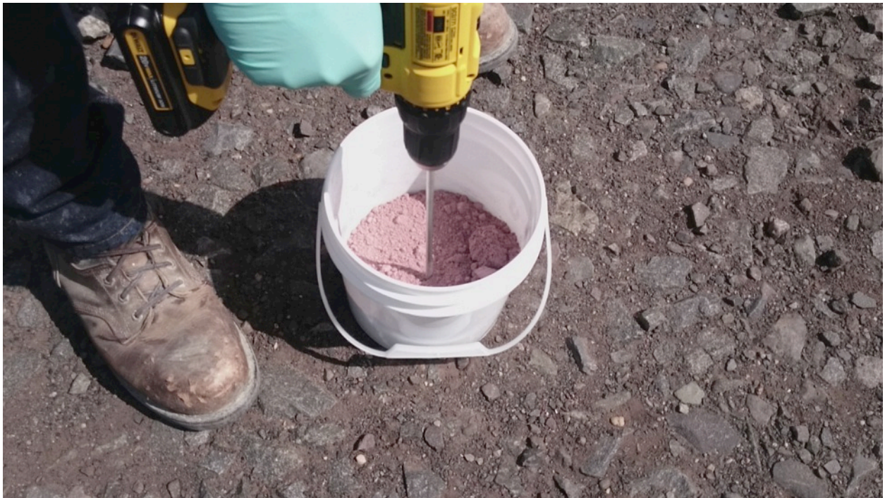
Figure 15. Preparation of Red Metallic Primer Coating Mixture
