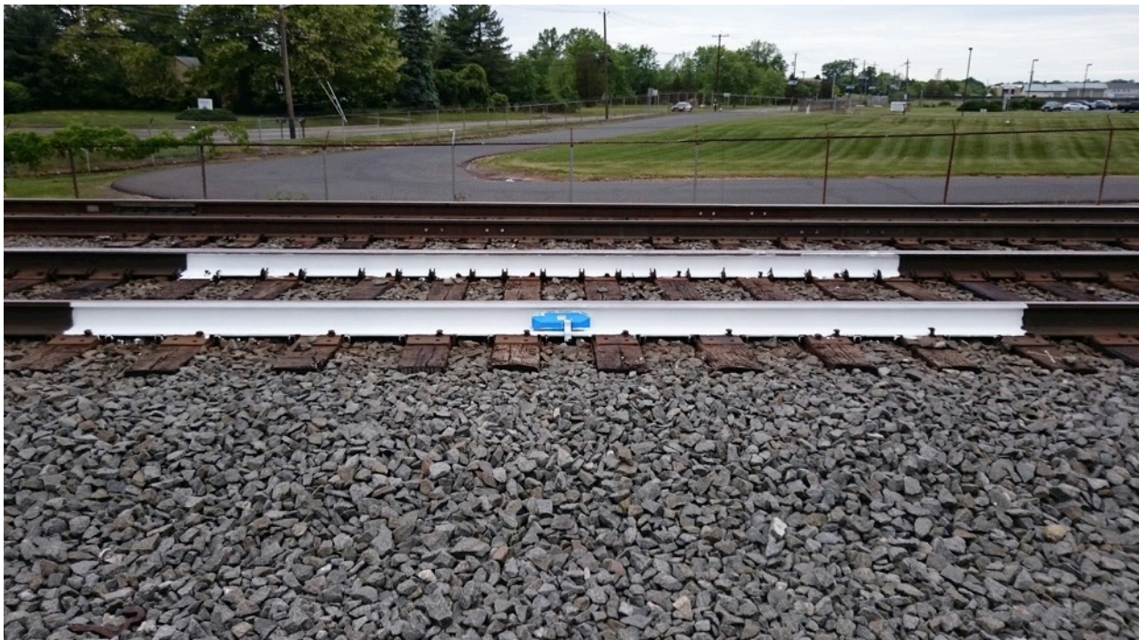
Figure 21. Completed Coating Application and Sensor Installation on Rail
