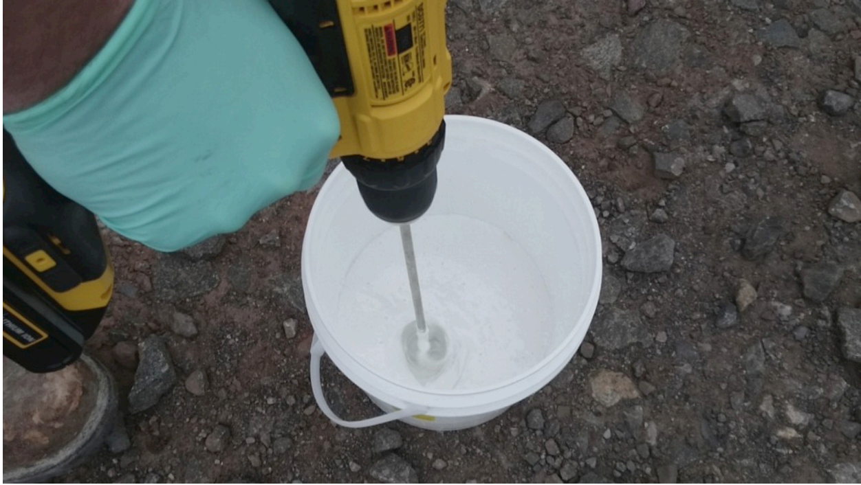
Figure 18. Preparation of White Surface Coating
