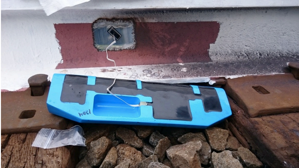
Figure 20. Sensor Installation on Rail with Coating
