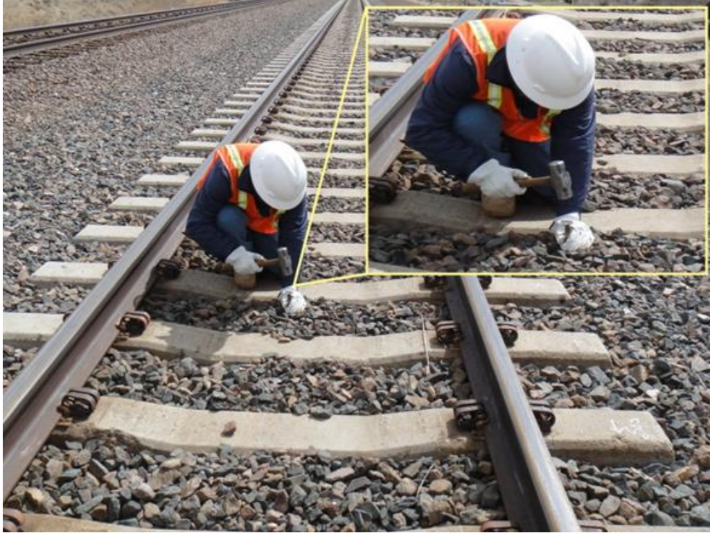
Figure B.2. Driving Spikes into Ballast to Couple Receivers to Ballast
