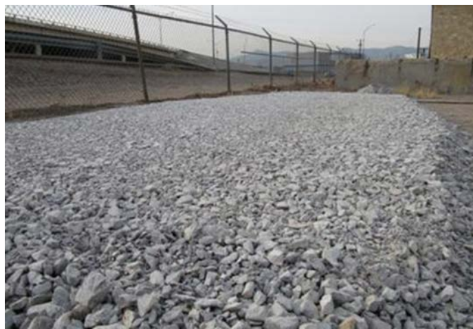
Figure 30. Ballast Test Pad for Large Scale Seismic Testing Near UTEP
