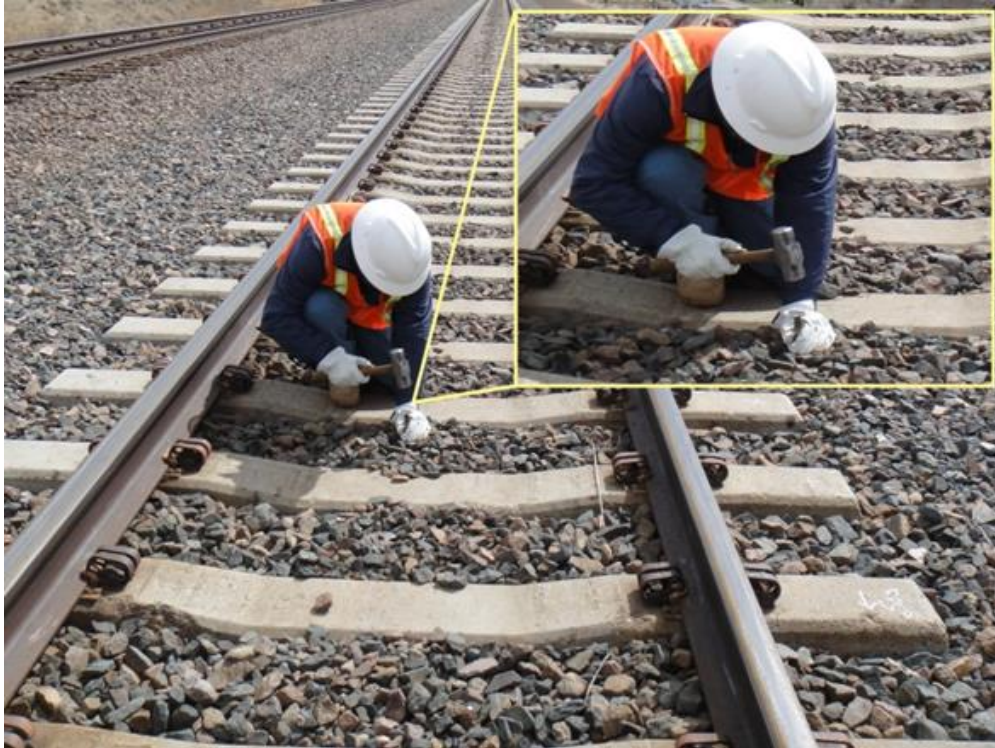
Figure 59. Driving Receiver Spikes into Ballast with Small Hammer
