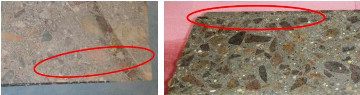
**Figure 10.33. Cracking due to stress release from saw-cutting**
