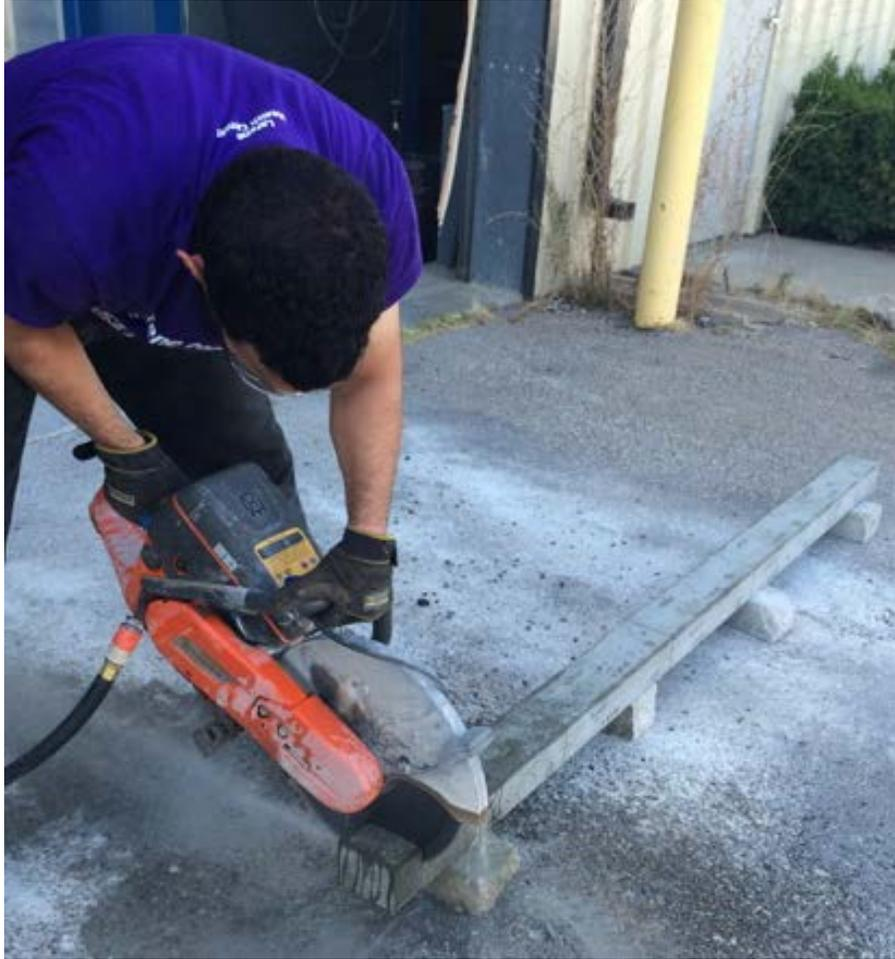
**Figure 5.38. Saw-cutting long beams**
