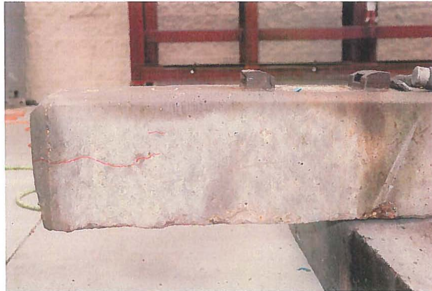
Figure 52. Opposite side view of south end of tie NDT #2. L3672 102312 63
