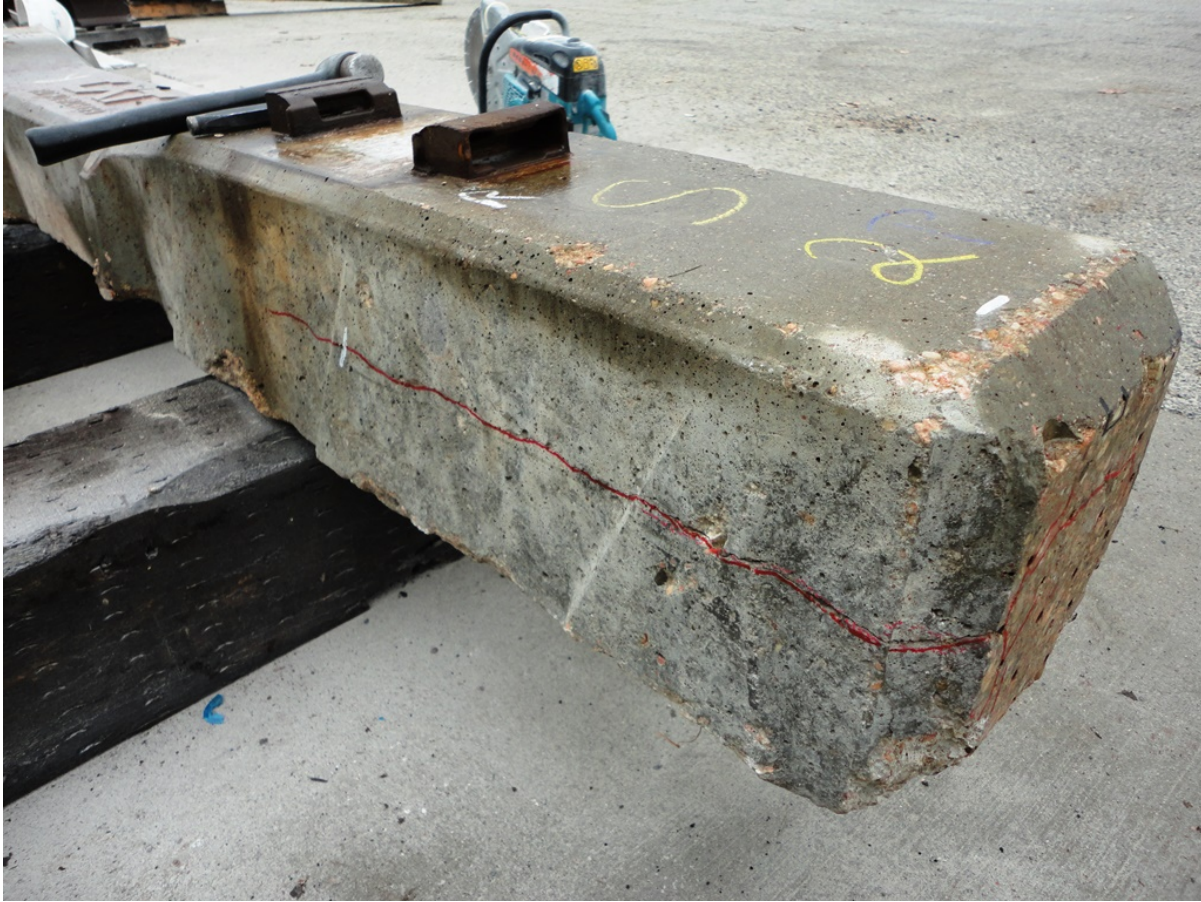
Figure 4. Tie 2, South, Showing Horizontal Crack
