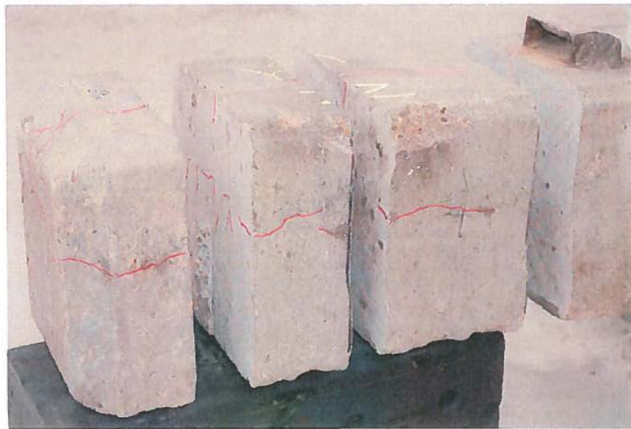
Figure 32. Side view of successive sections removed at north end of tie NDT #69. L3672 102312 41
