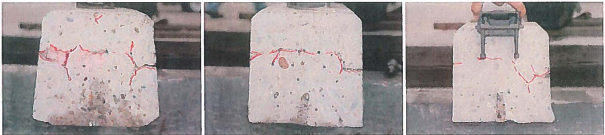
Figure 48. North end cross-sections of tie NDT #2 at saw cuts at 6 inches (left), 10 inches (center) and 21 inches at center of rail pad (right), all visible cracks outlined in red.
