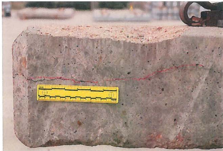
Figure 8. Closer side view at north end of tie NDT #7. L3672 102312 06
