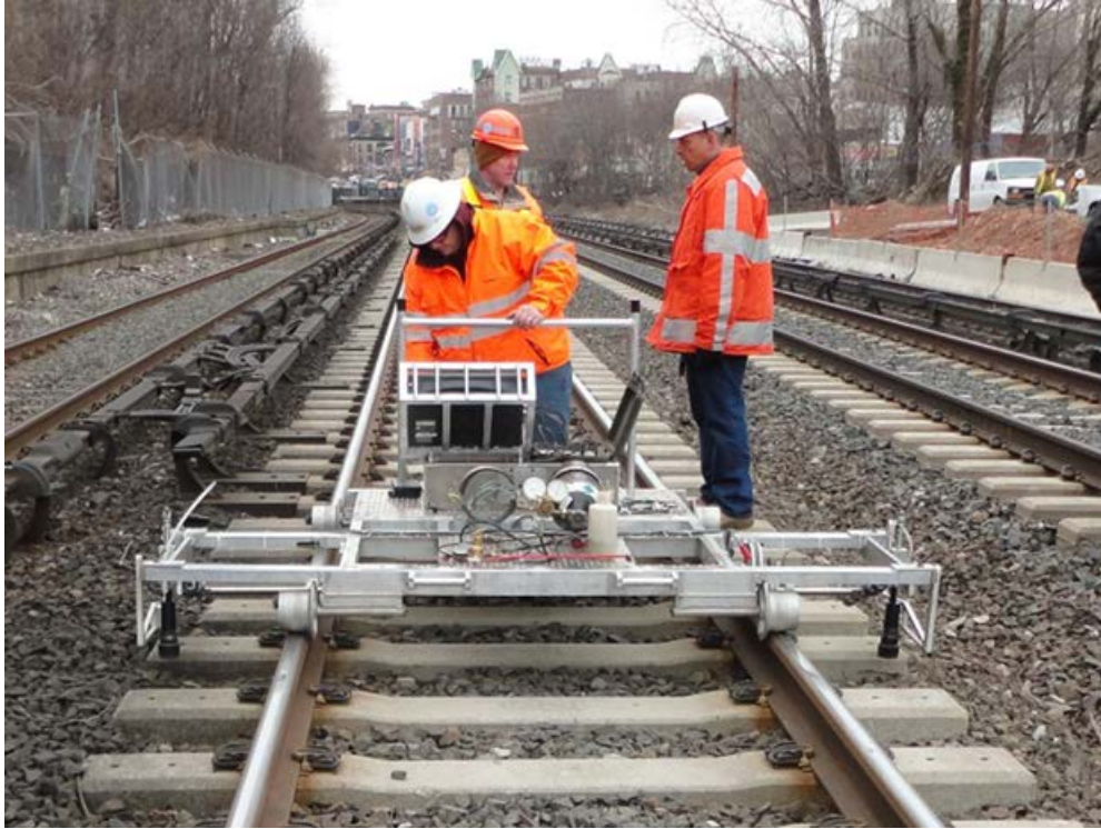
Figure 8. ACTT-1 System on Metro-North Railroad
