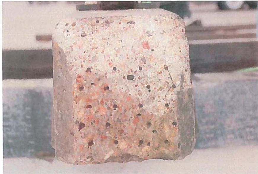
Figure 40. North end view of tie NDT #2, significant spalling at top chamfer. L3672 102312 48
