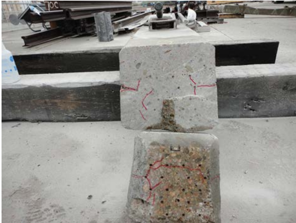
Figure 6. Example of Internal Cracking
