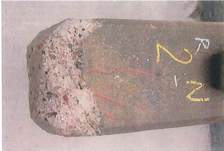
Figure 41. Top surface of north end of tie NDT #2. L3672 102312 46
