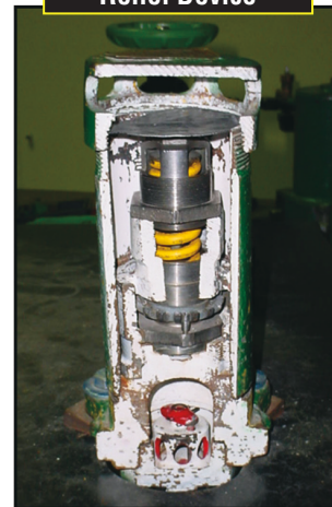
Chlorine Safety Relief Device
