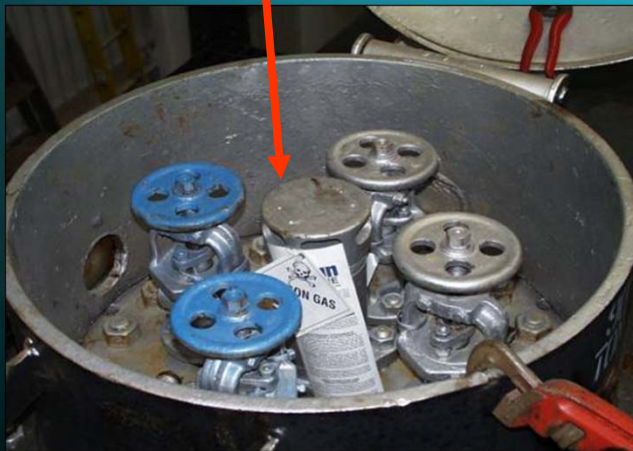
Pressure Relief Device (Chlorine – Combination)
