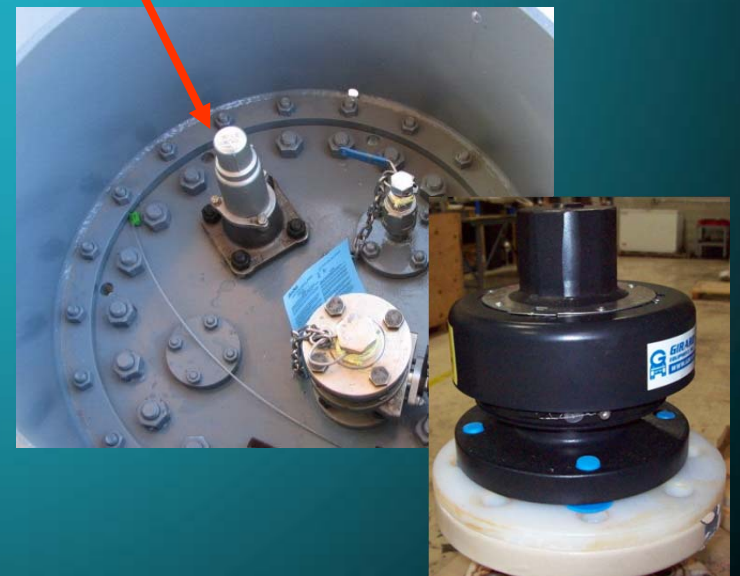
Pressure Relief Valve (Non-pressure – Reclosing)
