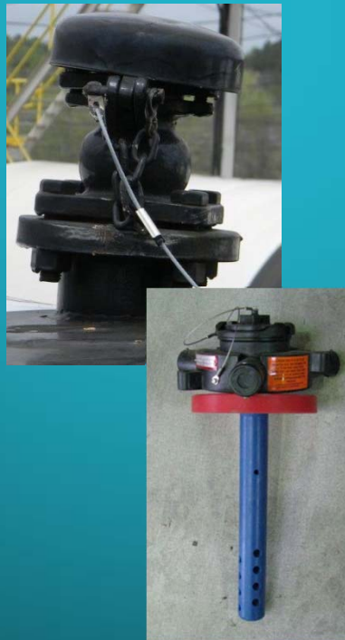
Rupture Disc Housing (Non-pressure – Non-reclosing)
